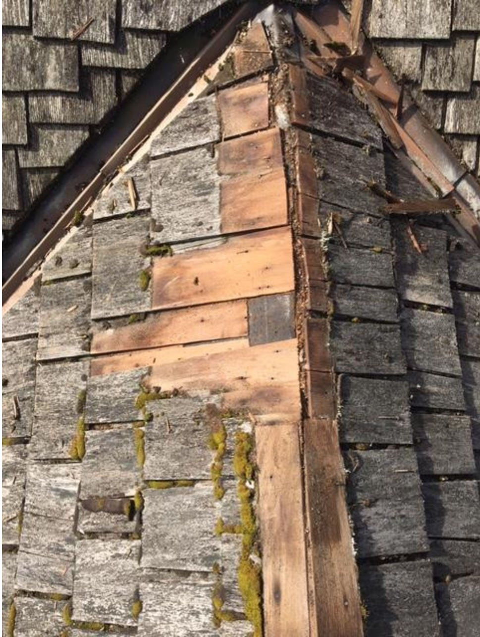
Lodge Building - Non-asbestos felt beneath cedar shingles.
