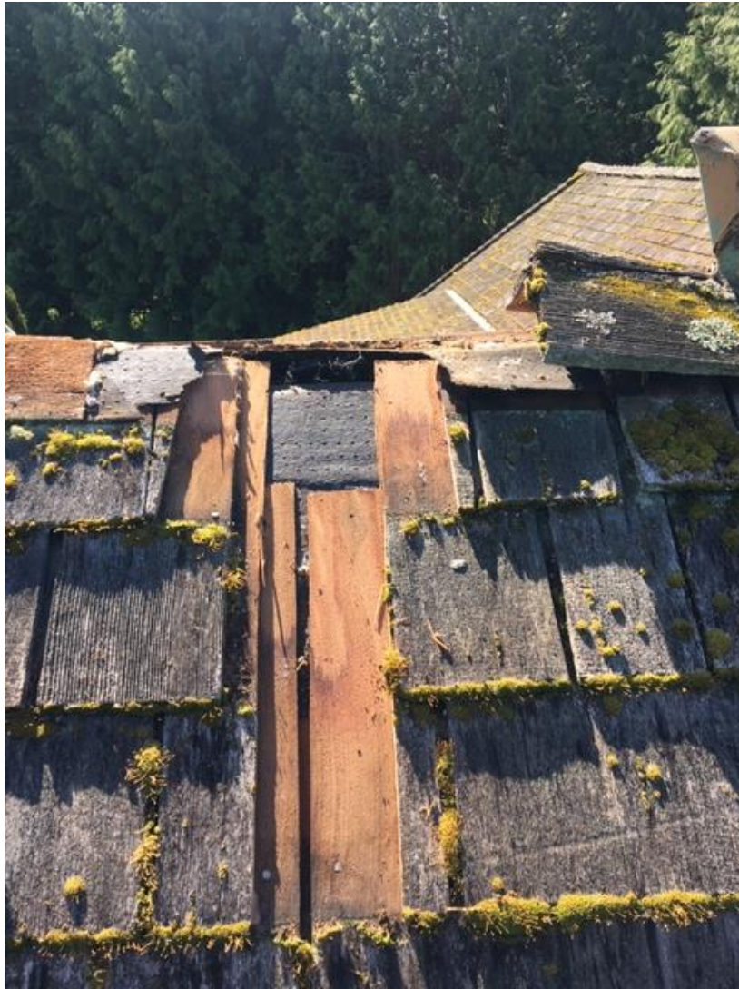
Science Building - Non-asbestos felt beneath cedar shingles.
