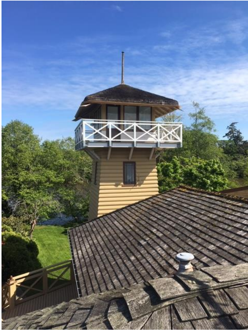
Lodge building roof and observation tower in background.
