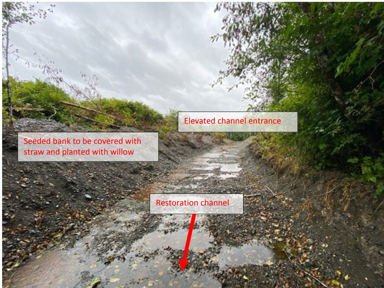
Figure 5: Restored Channel looking Upstream – adapted from Instream Fisheries Research Inc. Report.
