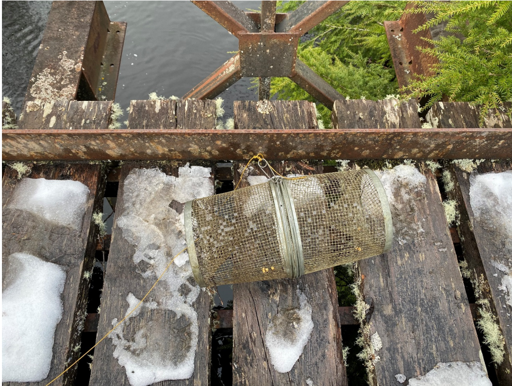
Photo 10: Empty Retrieved Trap Upstream of the Bridge.
