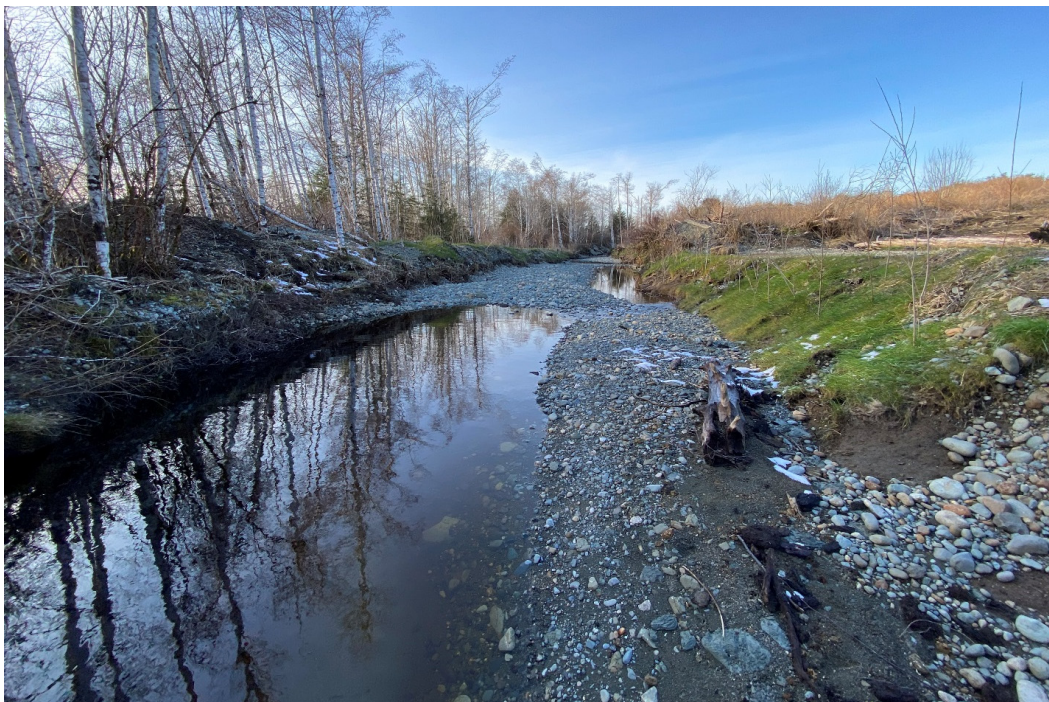
Photo 11: High Flow Bypass Channel looking downstream (northward).
