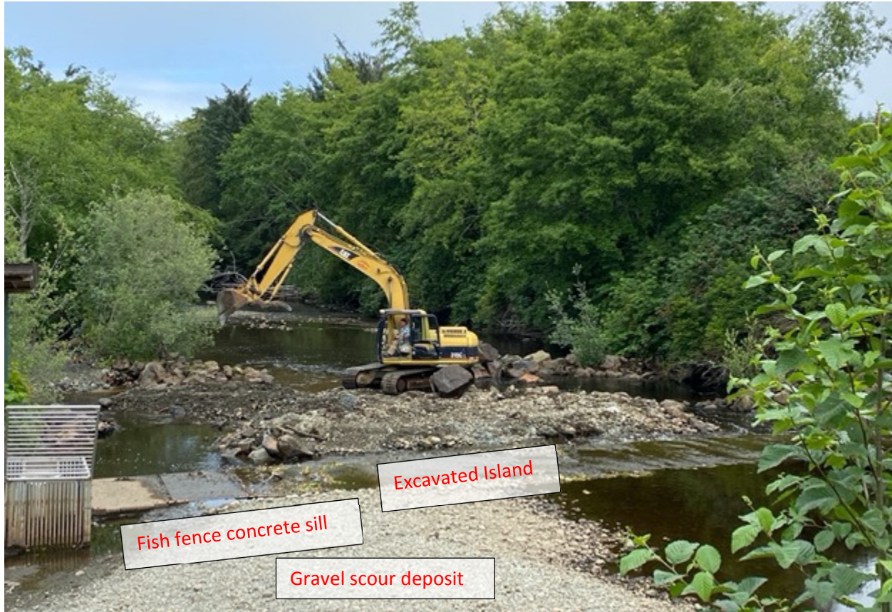
Figure 3: 2020 Outflow Channel Restoration Works – adapted from Instream Fisheries Research Inc. Report.
