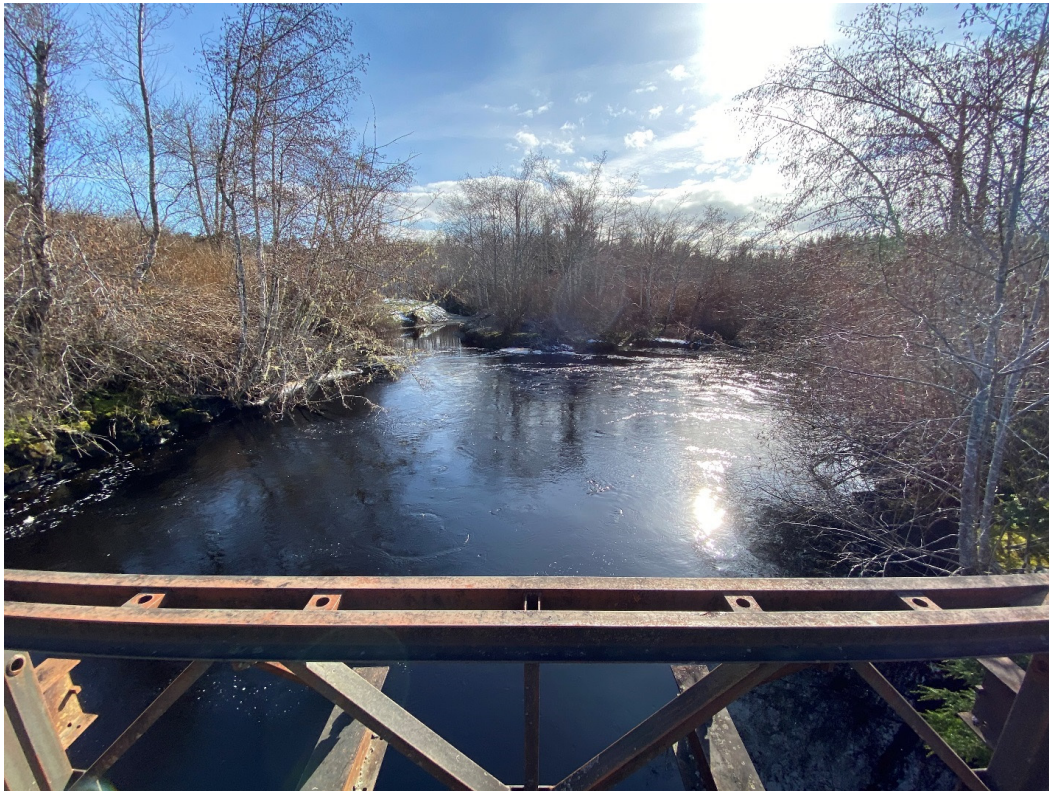
Photo 2: Keogh (Giuuyux) River looking upstream from the existing bridge.
