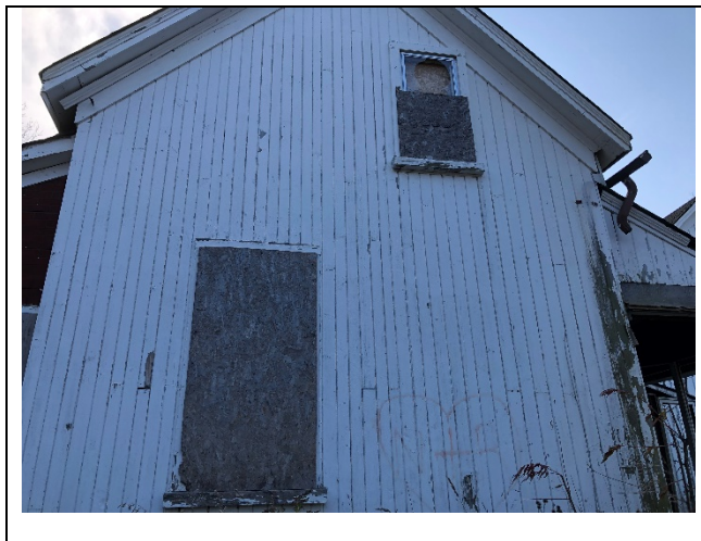
Photo 6: Lead-containing white paint on the exterior.
