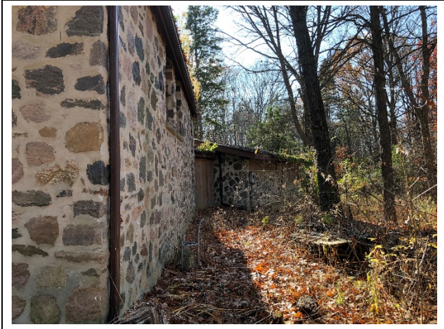
Photo 1: Exterior of 4 Reesor Road, Toronto, Ontario.
