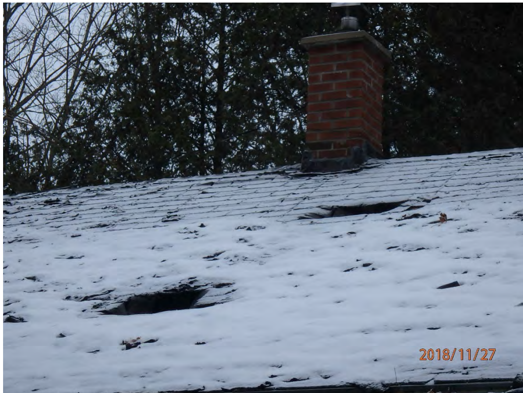
Photo 2: View of the holes in the roof of the building.
