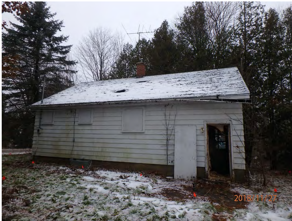
Photo 1: View of the south side of the subject building and potential asbestos-containing roofing materials.
