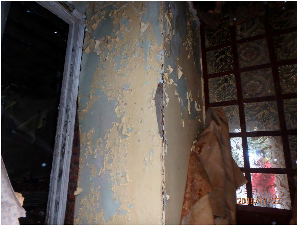
Photo 5: View of the lead-containing yellow paint on the side entrance walls.
