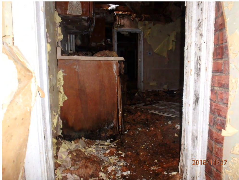
Photo 4: View of the condition of the kitchen at the subject building, including possible visible mould.
