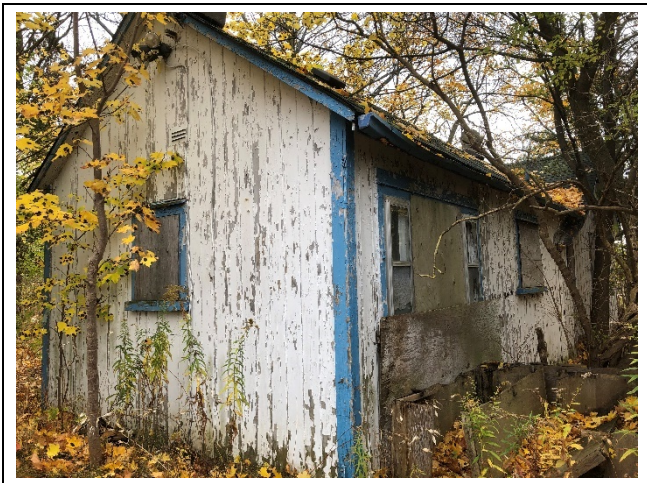
Photo 1: Exterior of abandoned house at 2260 Meadowvale Road, Toronto, Ontario.
