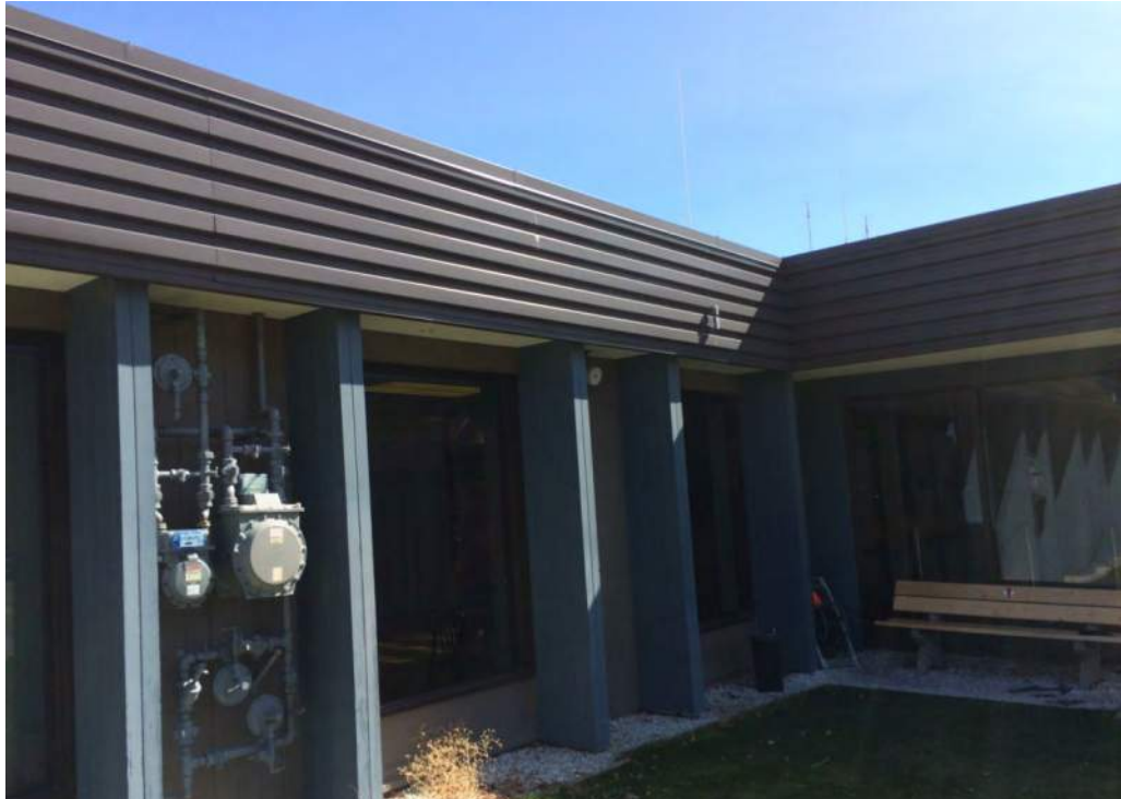
Photograph 1: West side of building (front entrance on right) – Facing southeast.
