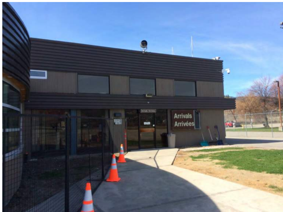
Photograph 6: Airside (east) arrivals entrance – Facing northwest.
