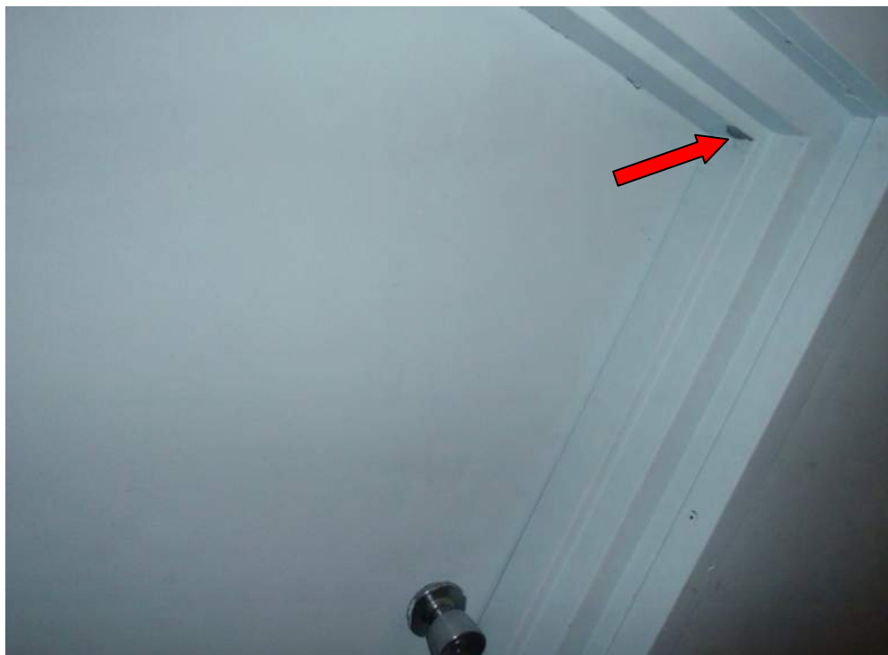
Photograph 68: Lead-based light blue/white paint on small door frame in Room 109 ( Sample P14 ).
