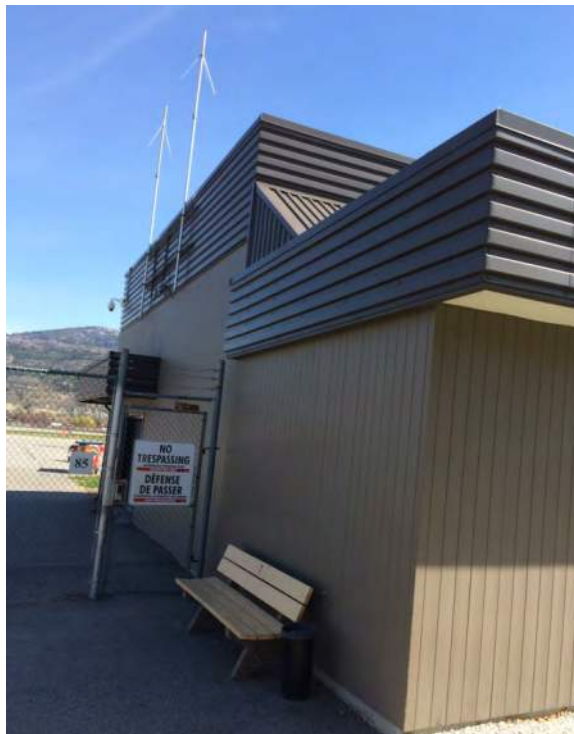
Photograph 2: North side of building – Facing east.
