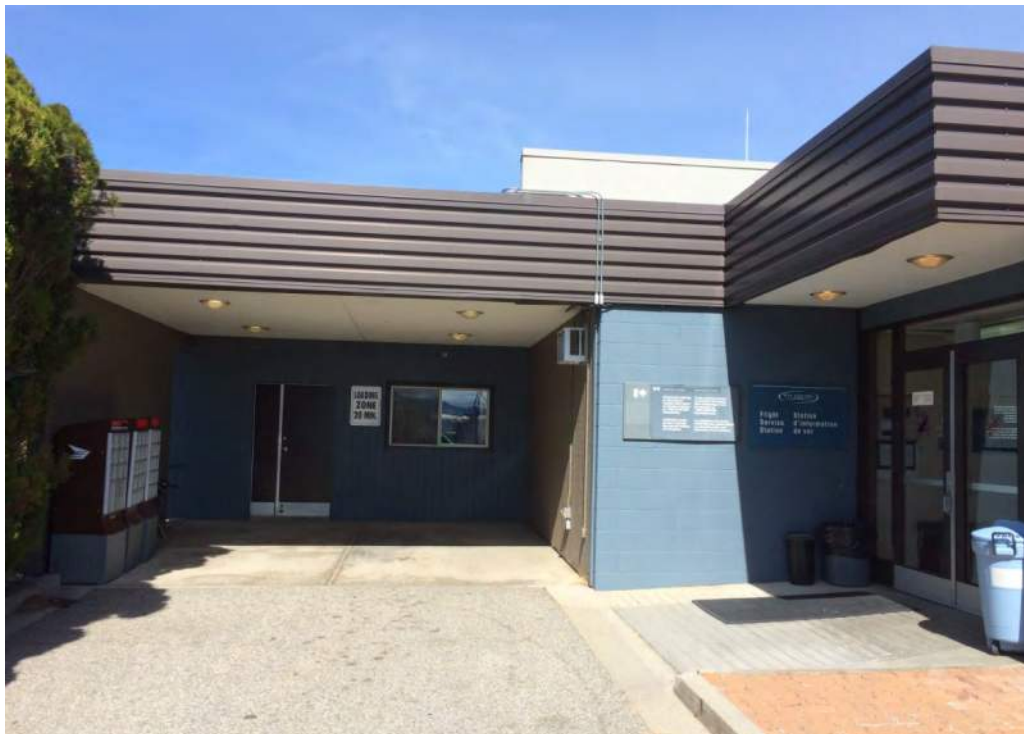
Photograph 4: South end of building – Facing north.
