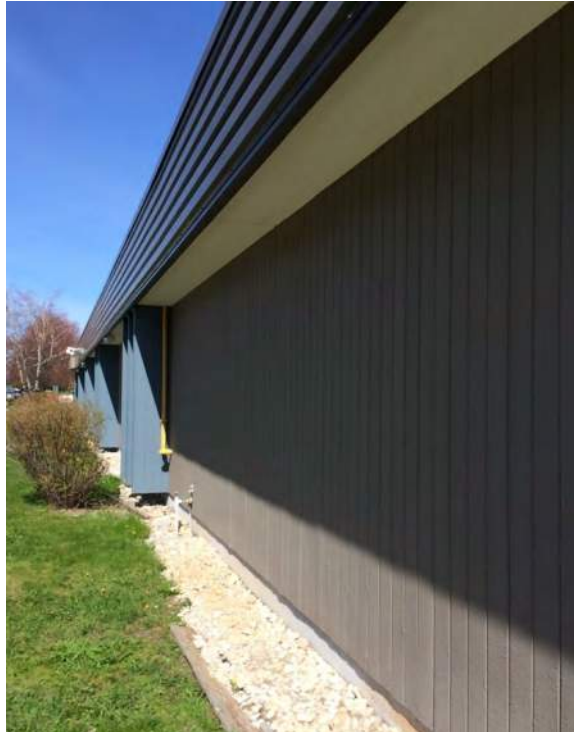
Photograph 3: Front (west) side of building – Facing north.
