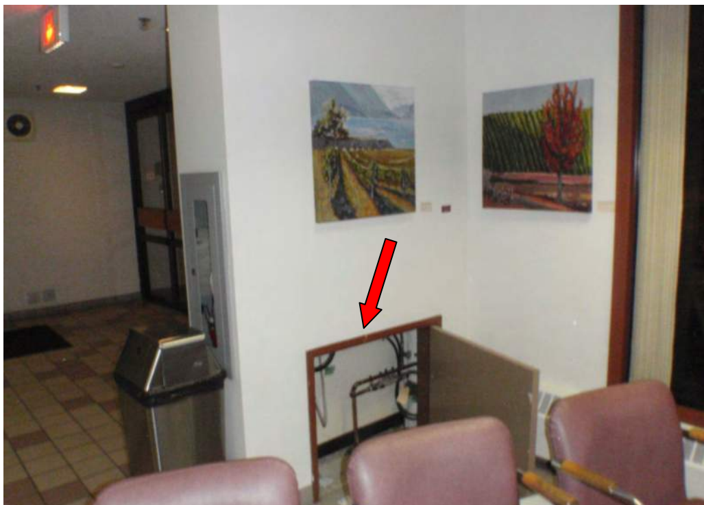
Photograph 12: Wall compartment in Room 106B (south wall), north of entrance – Facing southwest.
