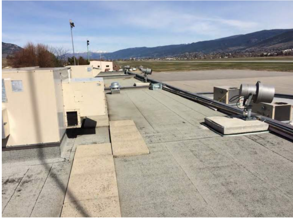
Photograph 9: Raised portion of roof – Facing north..
