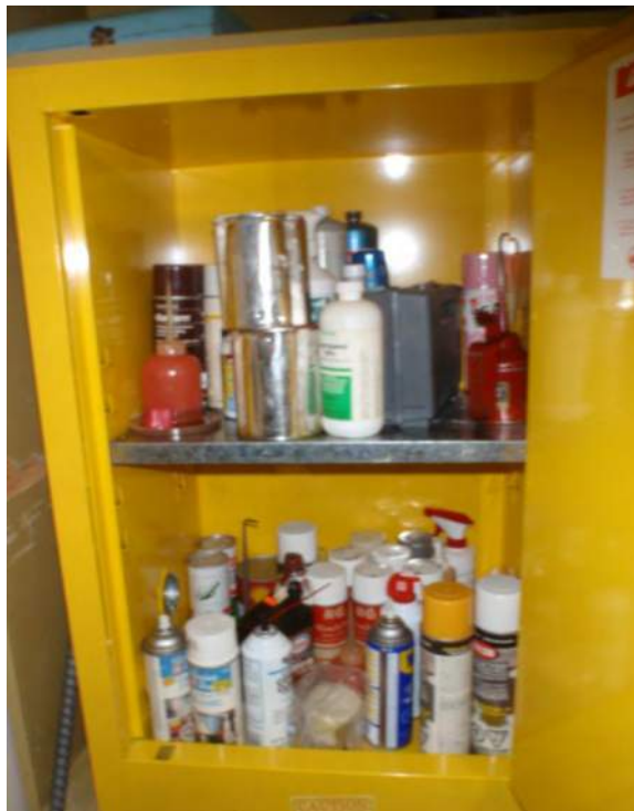
Photograph 20: Room 135 – Flammable storage box.
