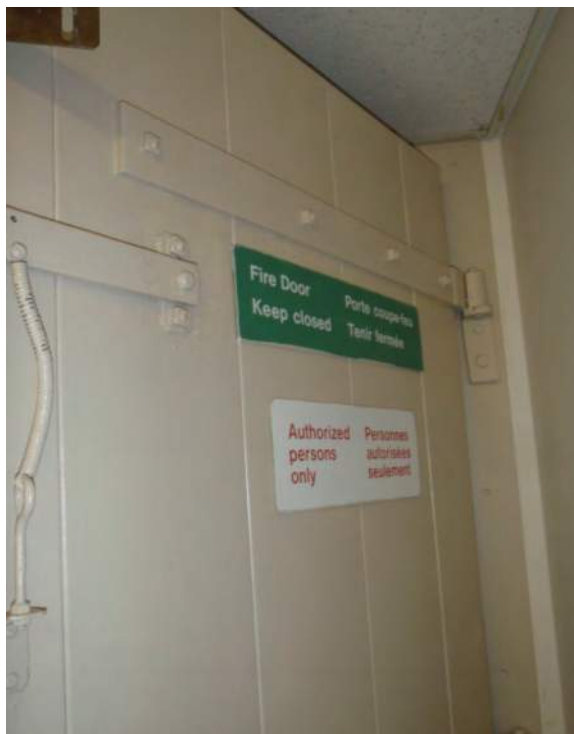
Photograph 58: Typical fire door to Room 137 (not sampled - inaccessible).
