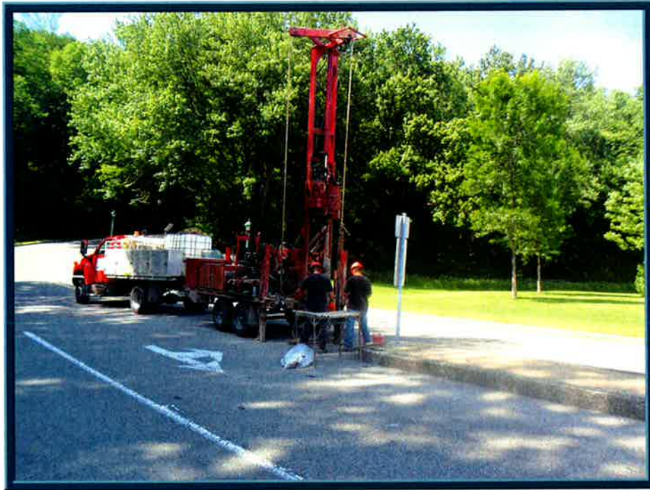
PHOTOGRAPH No. 5: Drilling rig at borehole TF-05-11 location.
