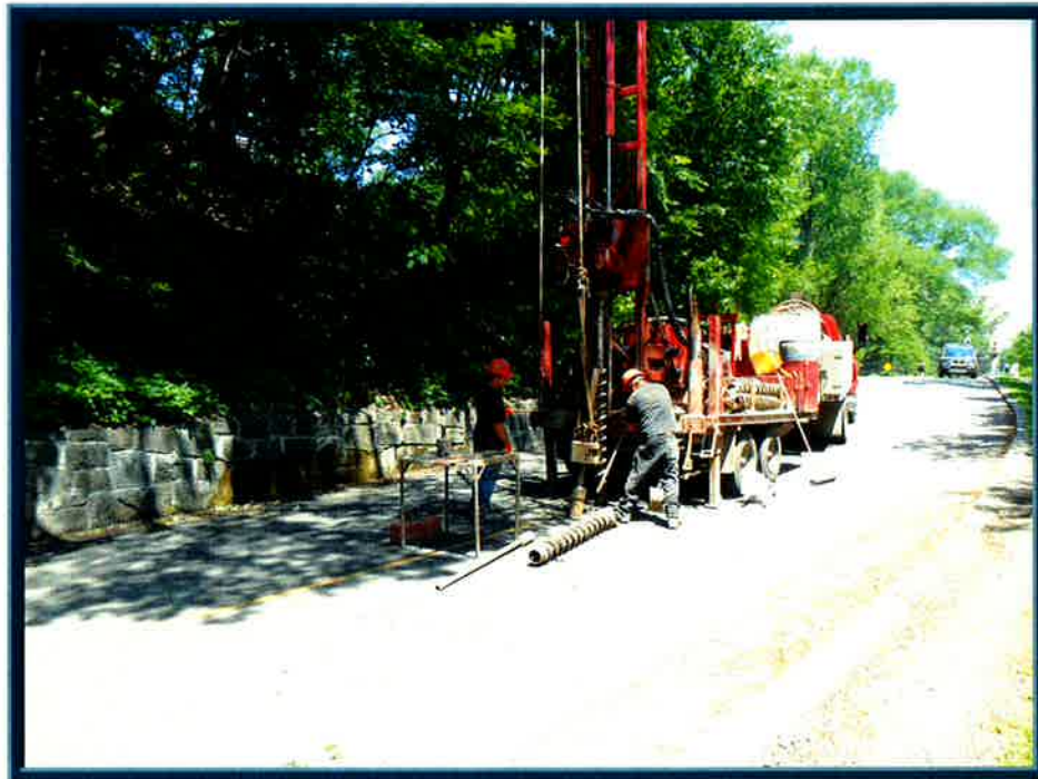
PHOTOGRAPH No. 2: Drilling rig at borehole TF-02-11 location.
