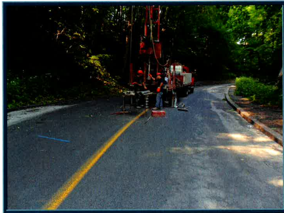
PHOTOGRAPH No. 4: Drilling rig at borehole TF-04-11 location.
