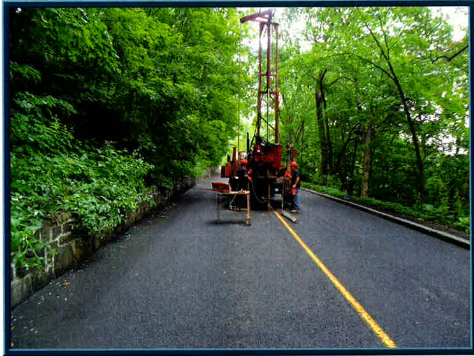
PHOTOGRAPH No. 3: Drilling rig at borehole TF-03-11 location.
