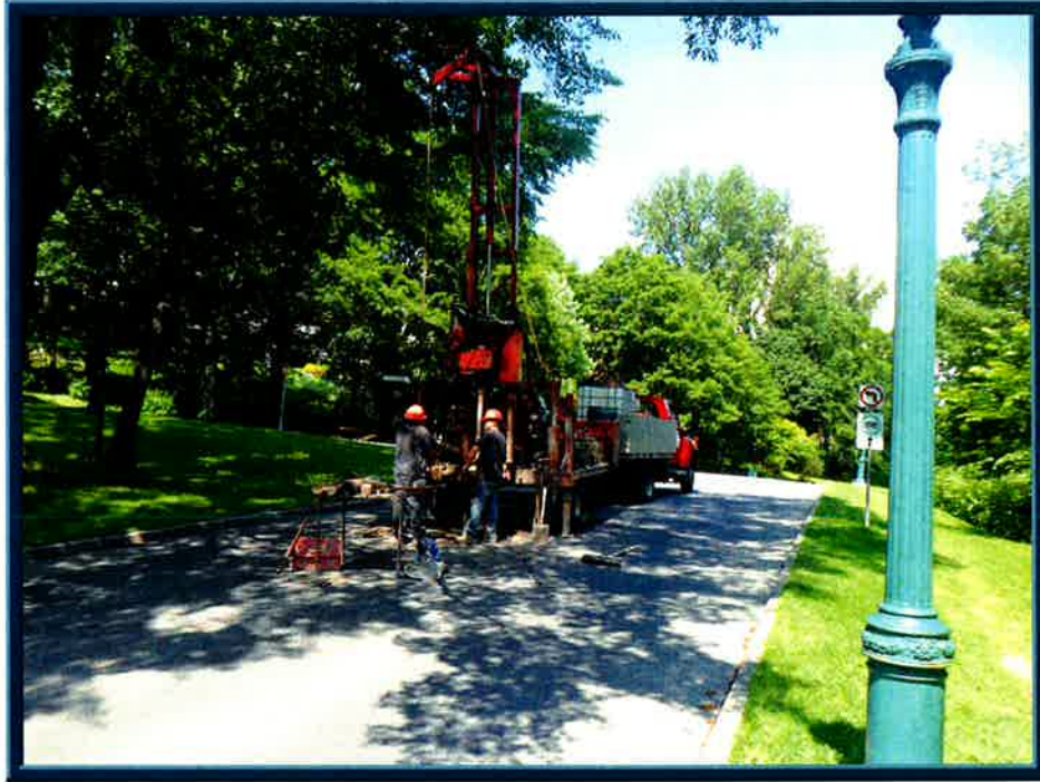
PHOTOGRAPH No. 1: Drilling rig at borehole TF-01-11 location.
