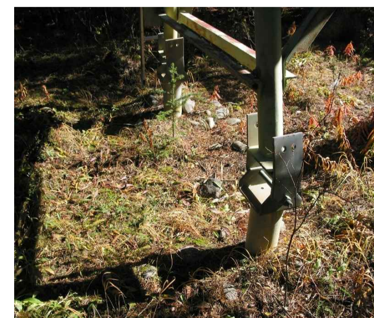
PHOTO 8: A-FRAME BASE AND TOP OF FOOTINGS
