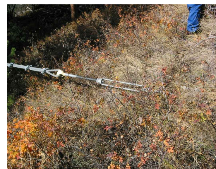
PHOTO 11: REPLACE HILL-SIDE ANCHORS SIDE VIEW
