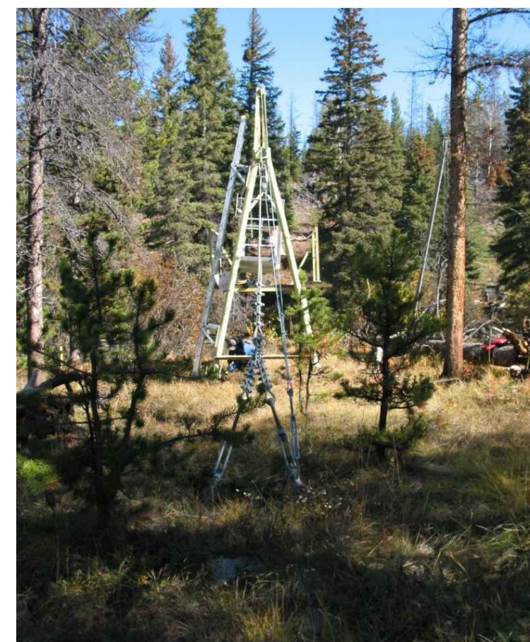
PHOTO 2: A-FRAME BACK VIEW
