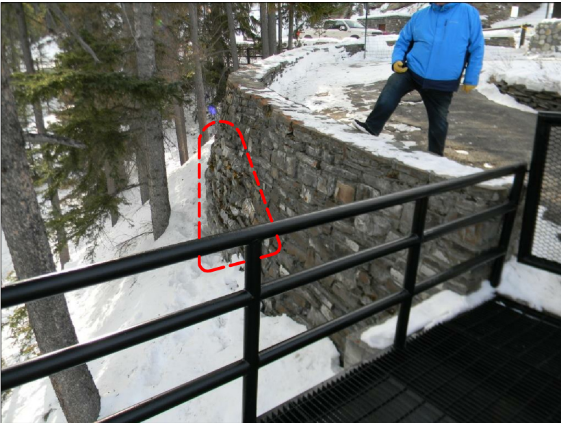
DET. 5/S2 - NORTHERN '3RD' OF CURVILINEAR LEG OF STONE RET. WALL (LOOKING SOUTHWEST). DASHED LINE SHOWS 'BULGE' IN STONE RET. WALL, INDICATIVE OF OVERLOAD.
