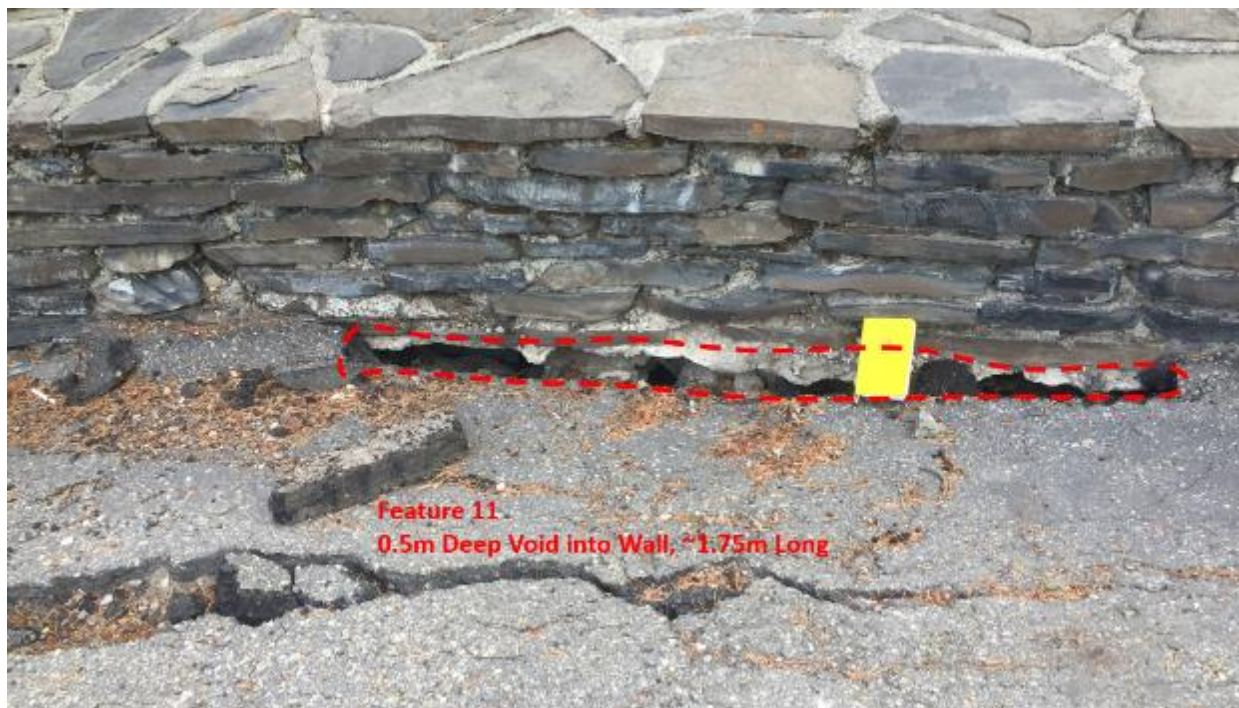
Photo 8: Void and asphalt degradation.
