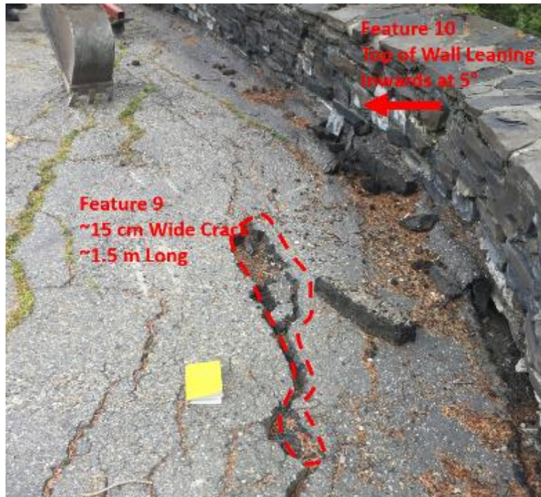
Photo 7: Asphalt deformations located approximately at the center of the wall.
