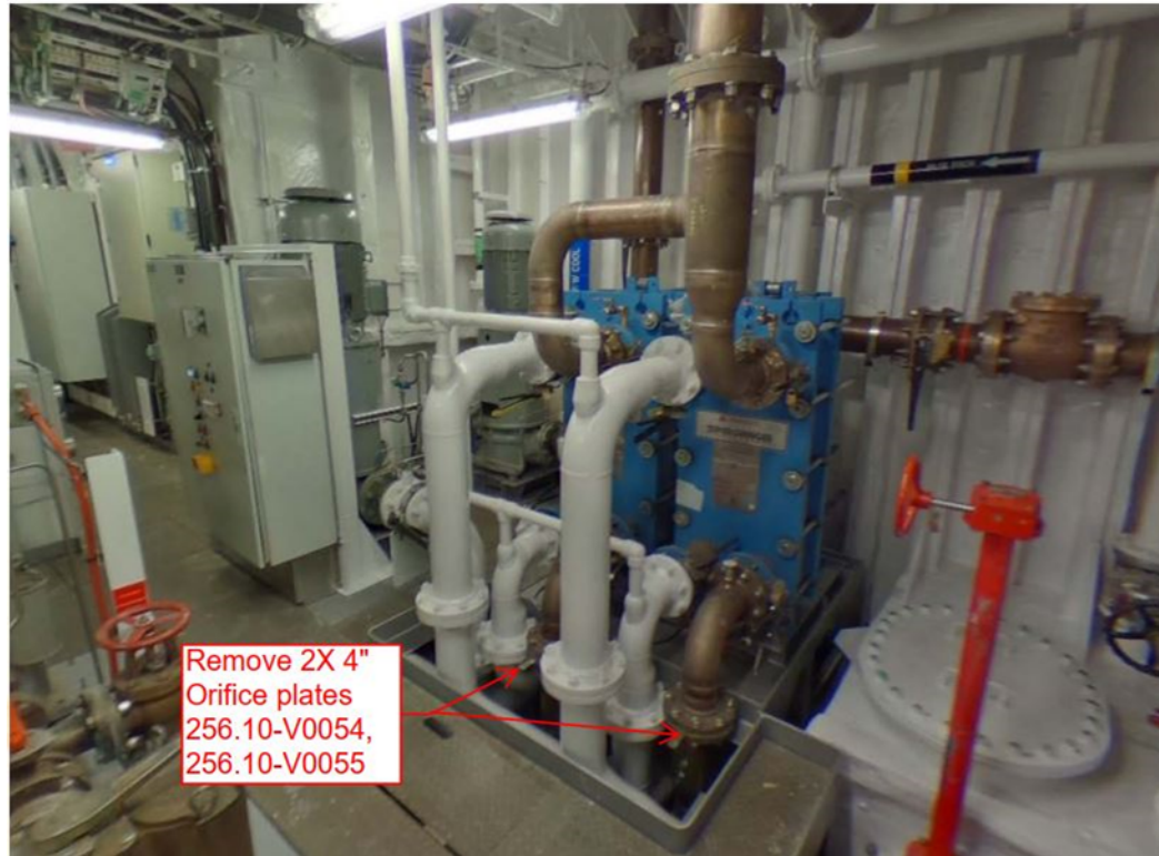
Figure 2: Orifice Plates at Heat Exchanger Inlet
