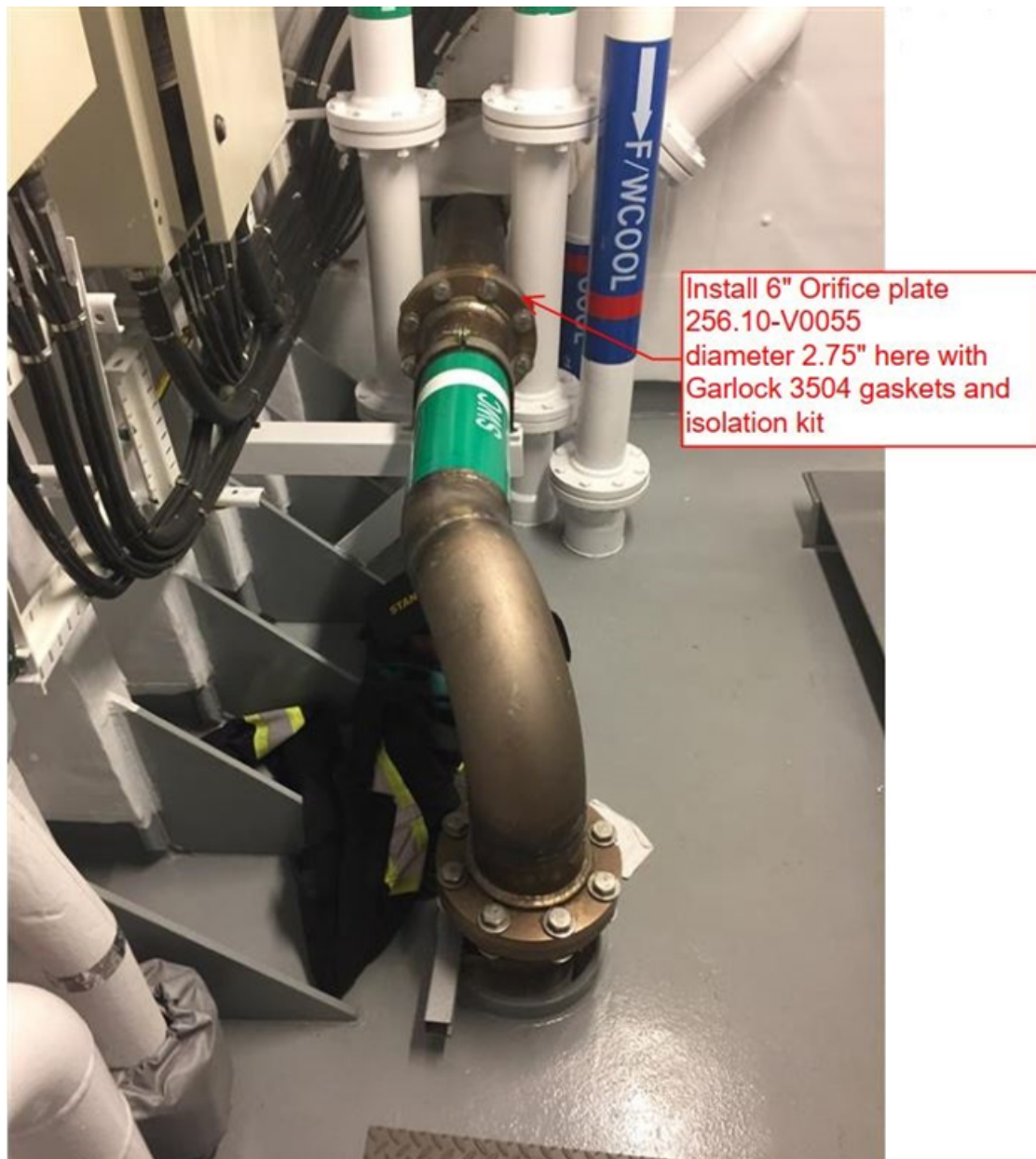
Figure 3: New Orifice Plate Location
