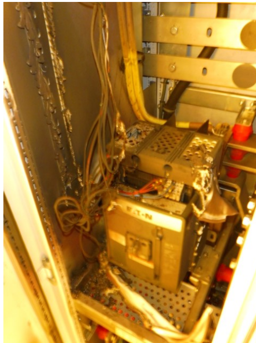
Figure 14: Failed Switch Disconnecter in Stbd VFD Cabinet +03.1
