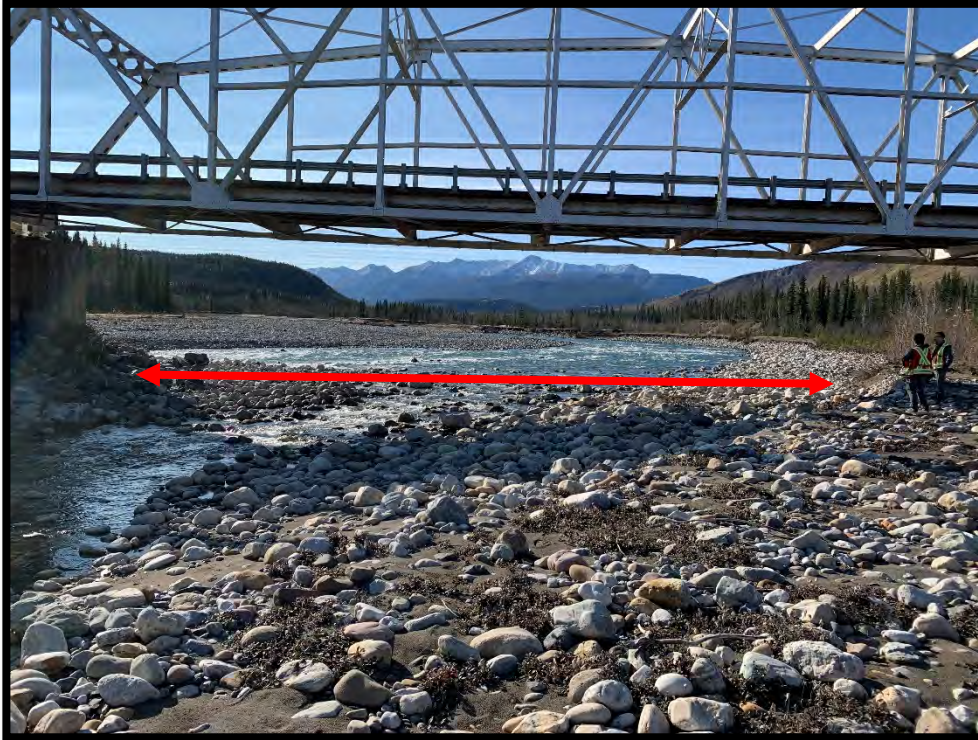
Photograph 7: Looking upstream along west channel at proposed access route.
