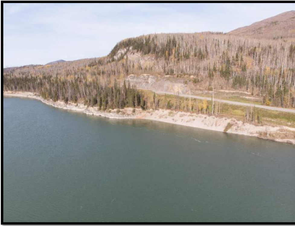
Photograph 4: Northern part of slope failure of Liard River bank
