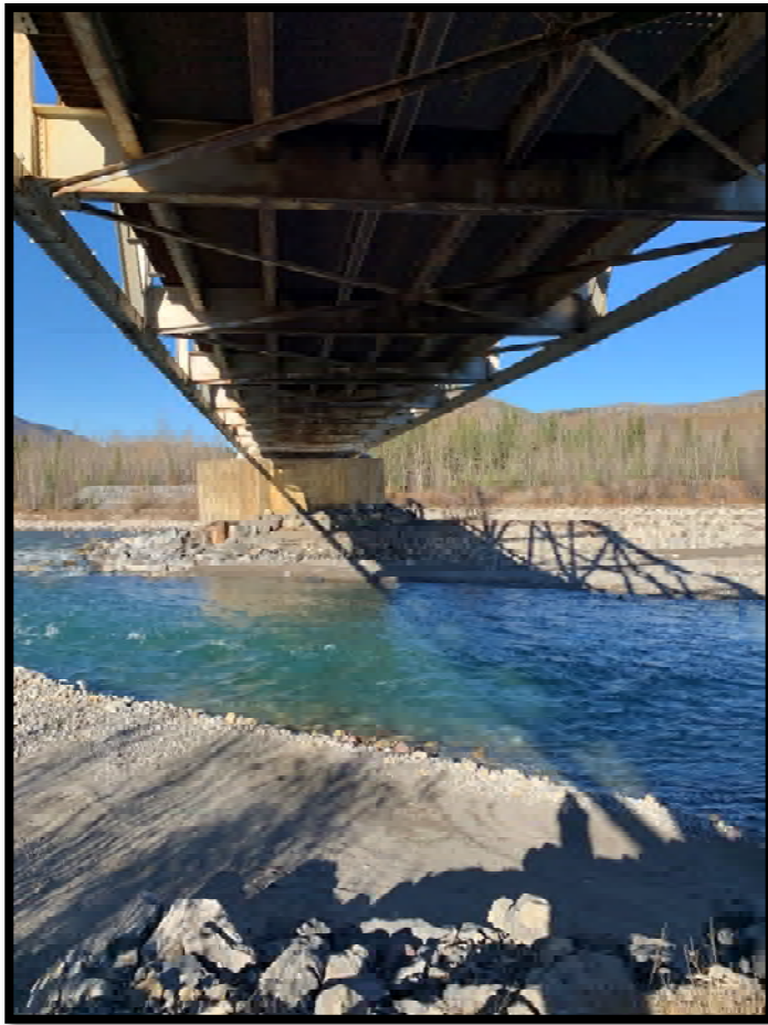
Photograph 11: View below bridge structure along east bank.
