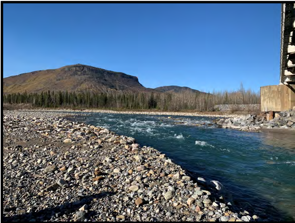
Photograph 8: Looking upstream along east channel.
