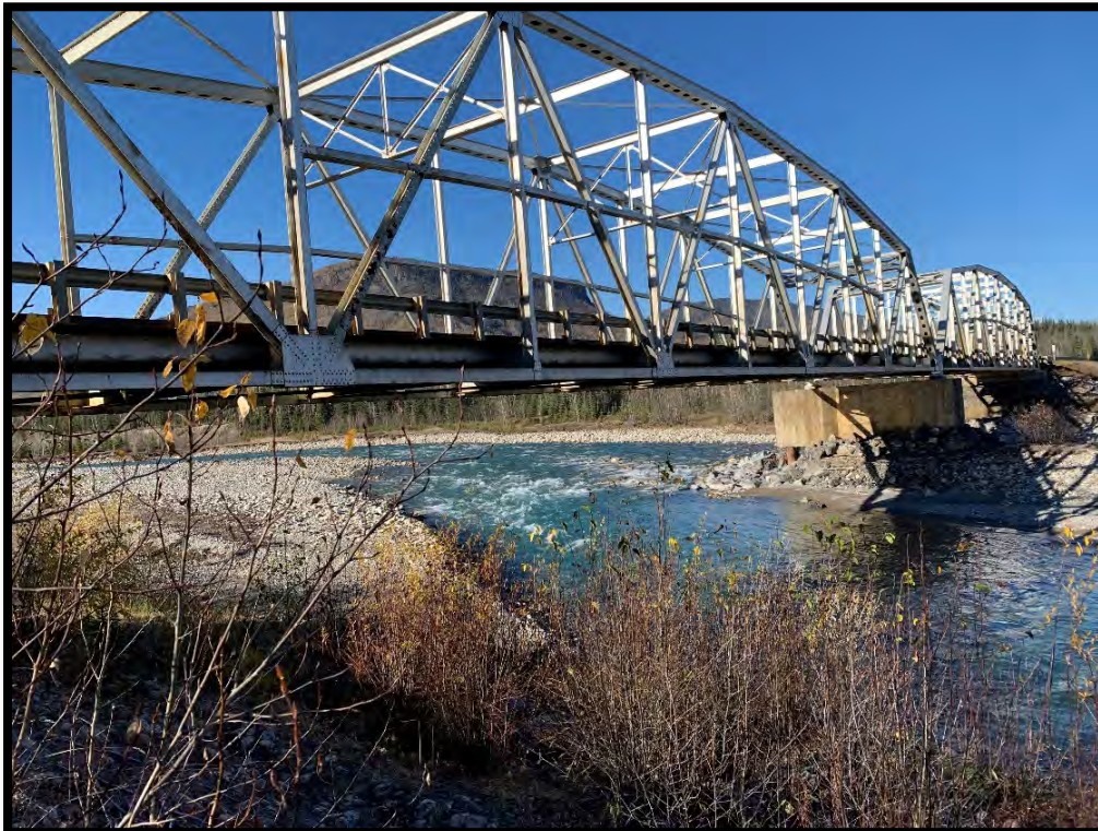
Photograph 10: View of bridge, downstream from east bank.
