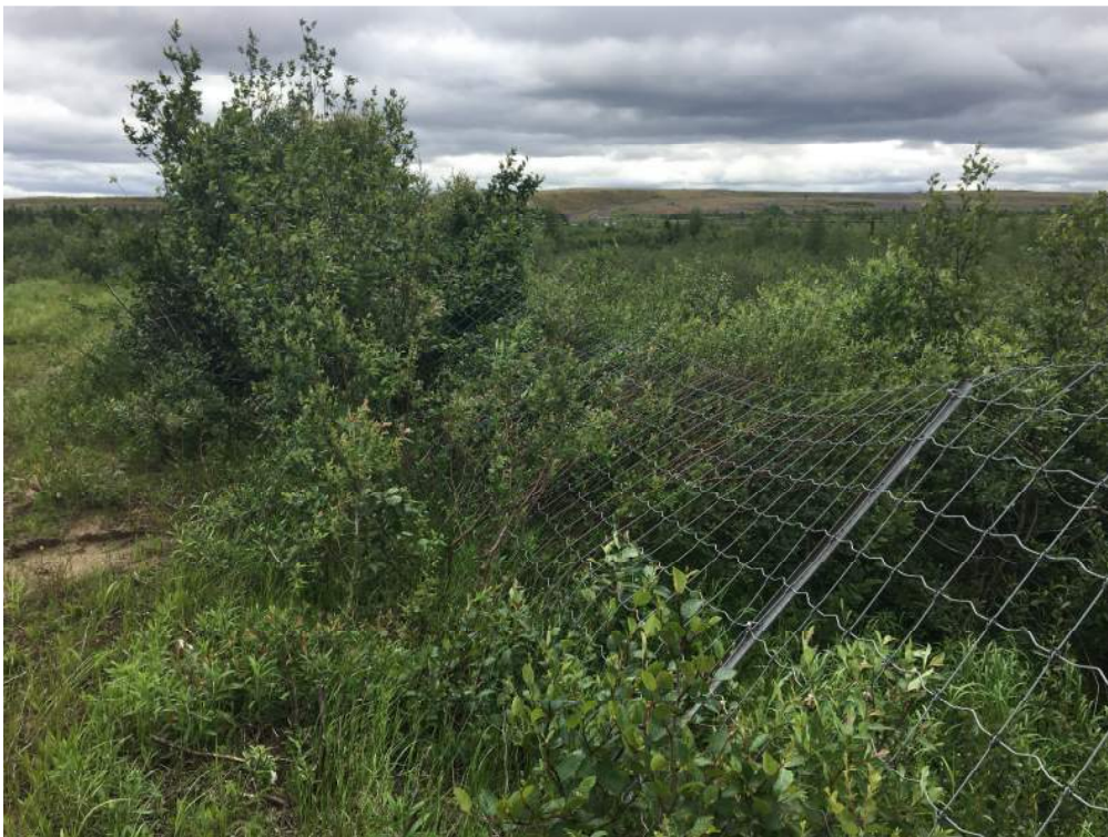
Photo 16 – Leaning fence and bent T-bar posts (Sta. 3+360).
