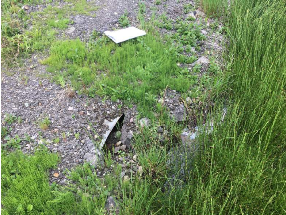
Photo 15 – Crushed culvert end and debris (Sta. 3+350).
