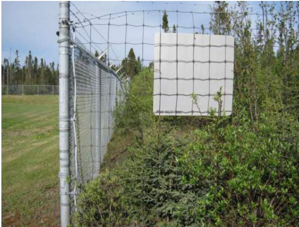
Photo 7 – Transition from chain link fence to wildlife fence. Heavy brush (Sta. 0+144).
