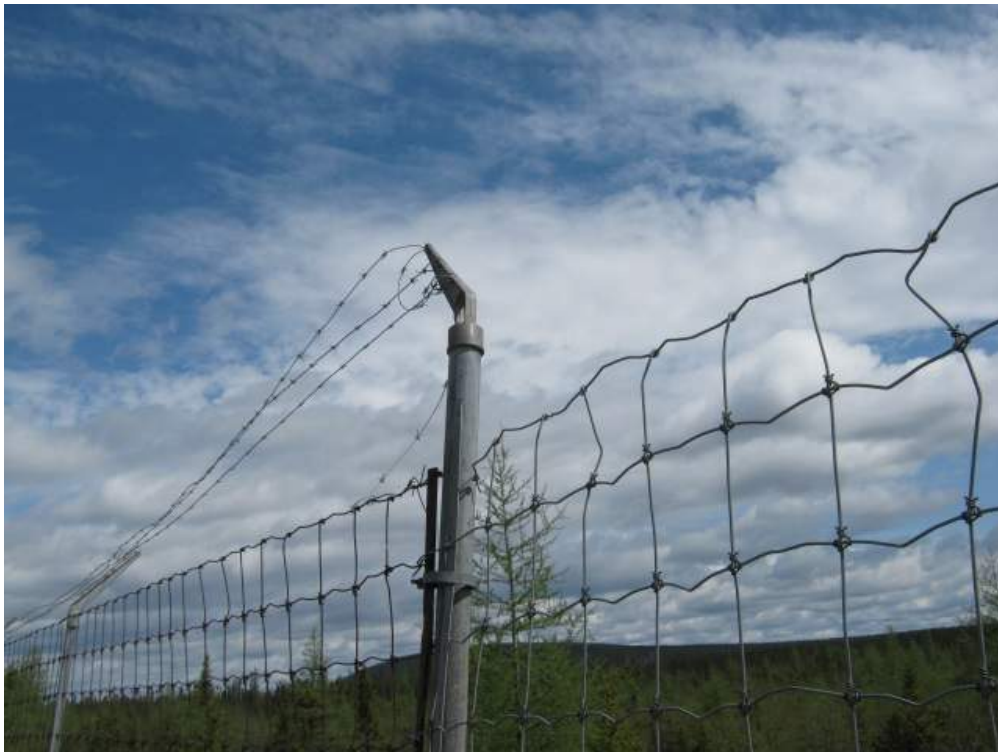
Photo 2 – Start of no barbed wire overhang (BWO) on east fence line (Sta. 1+884).
