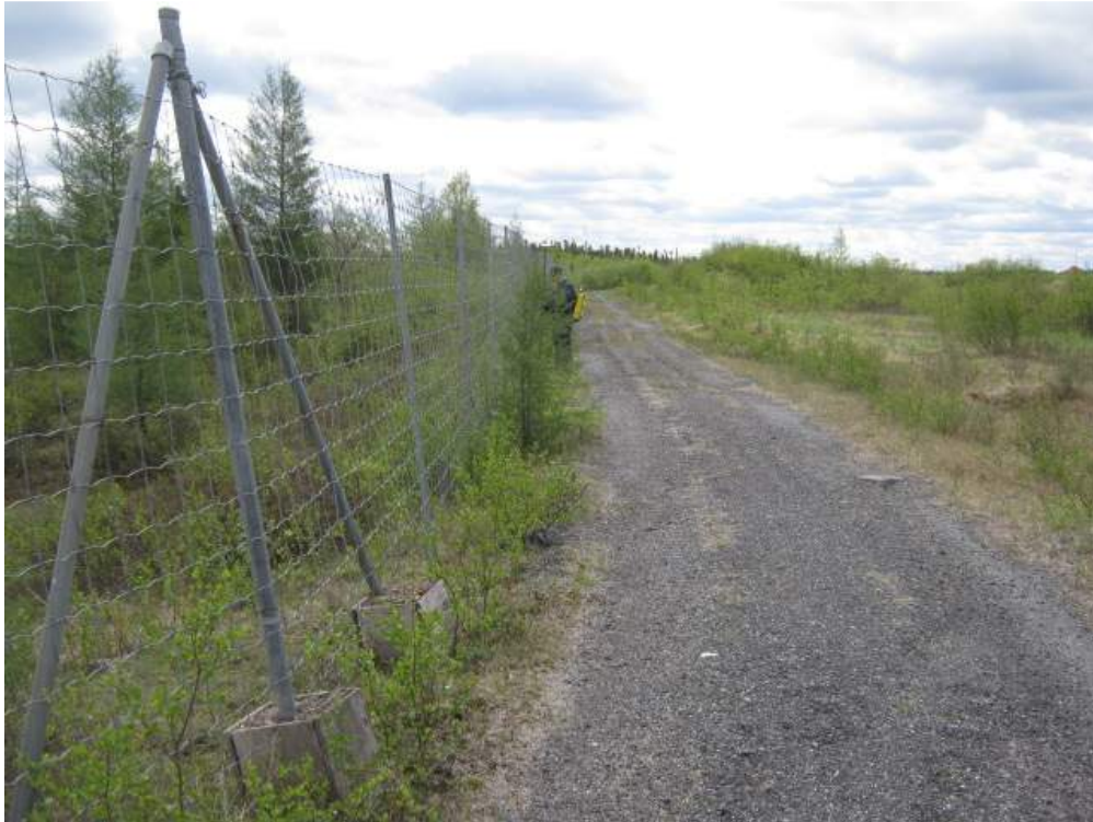
Photo 3 – Outward leaning fence along southeast fence line. Light brush and missing BWO (Sta. 2+631).
