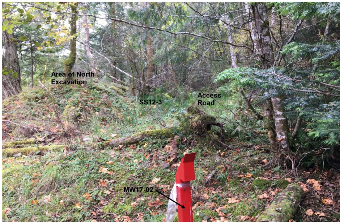
Photograph 10: North excavation area, looking southeast showing access road (excavation extent to be confirmed by contractor prior to start of work).
