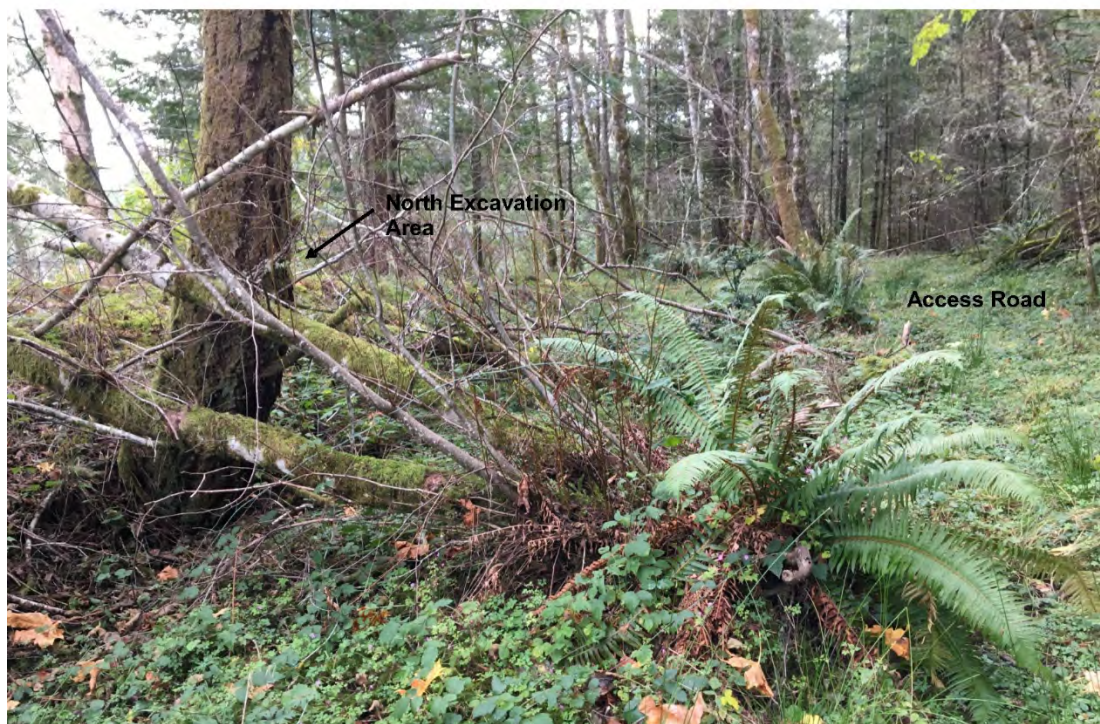
Photograph 12: North excavation area, looking southeast showing access road (excavation extent to be confirmed by contractor prior to start of work).
