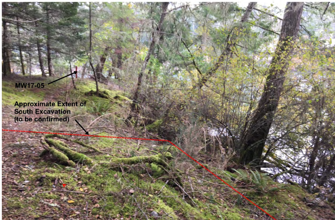
Photograph 8: Northern portion of south excavation, looking north (excavation extent to be confirmed by contractor prior to start of work).
