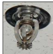
Showerhead of fire extinguishing system
