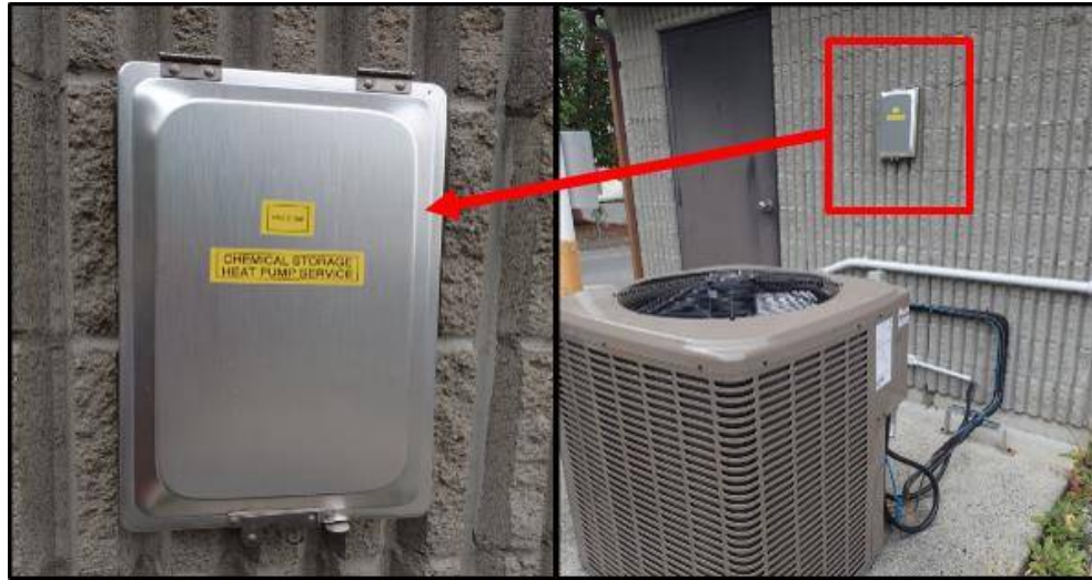
Figure 7: Example of aluminum, weather-resistant Service Record Storage Box for use with an exterior, Installed halocarbon system
