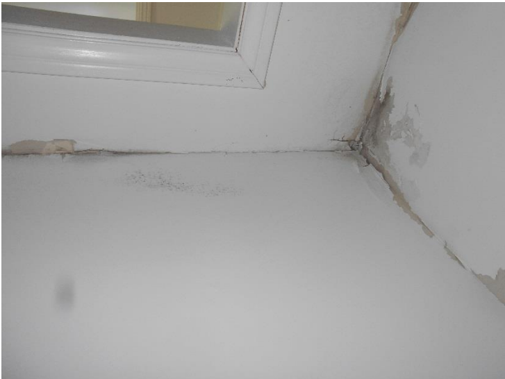
Photo 23 – View of suspected water leak and SVG observed in the Office Trailer, Room 1 (Porch).
