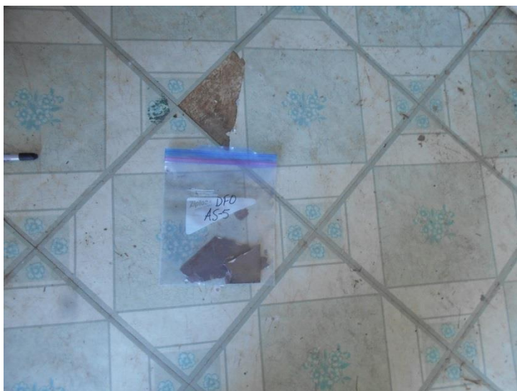
Photo 13 - View of bulk sample CA-AS-5 (green patterned vinyl floor tiles with brown mastic).
