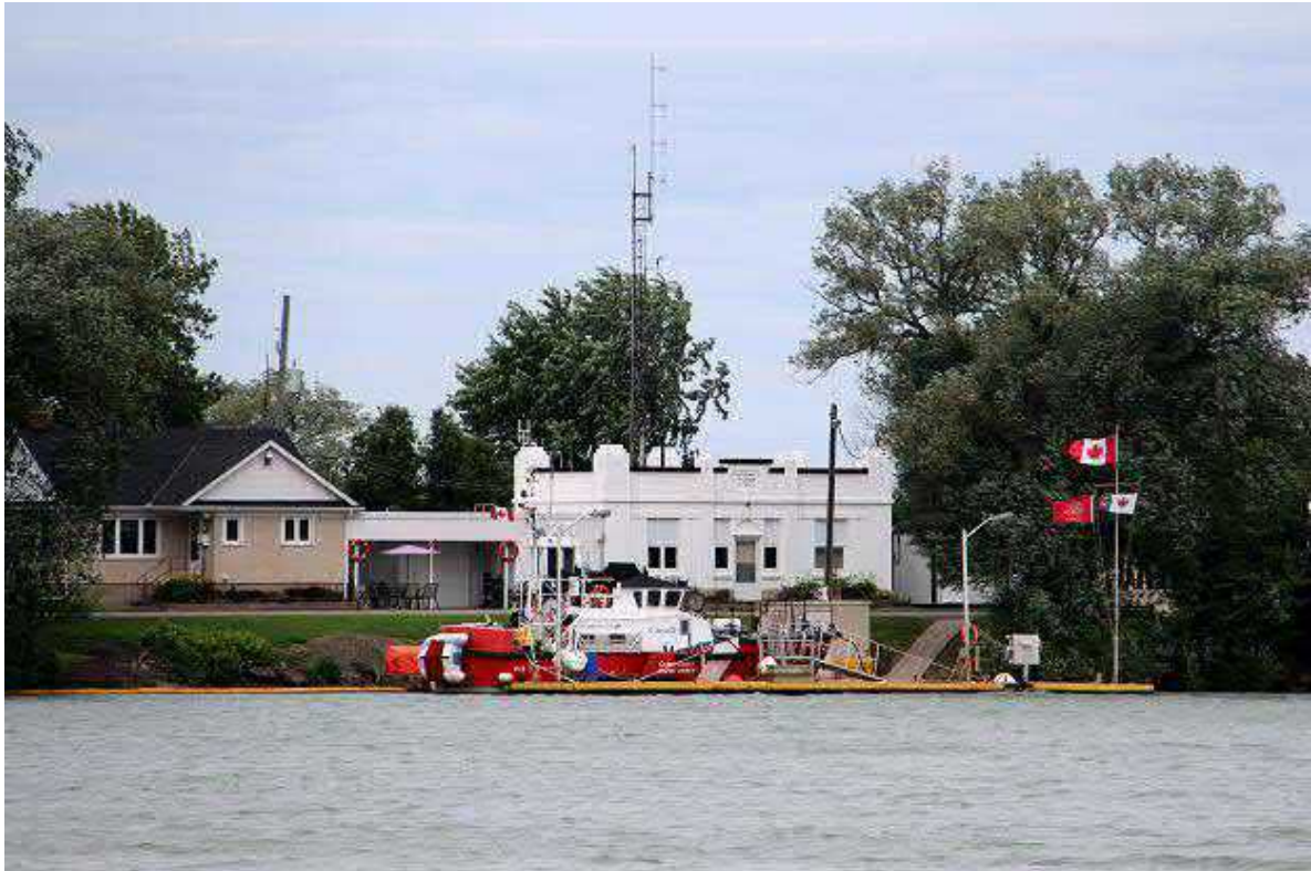
Photo 7: View looking west from the Welland Canal towards the Port Weller Search and Rescue Station (taken in July, 2017) (source: https://www.flickr.com/photos/21953562@N07/35892621973 ).
