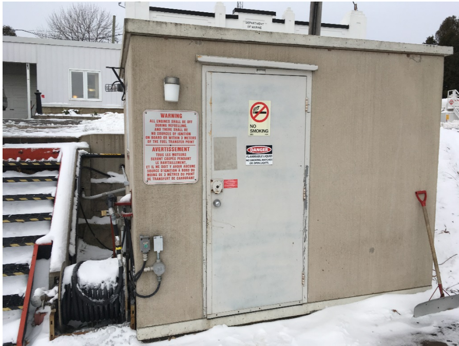
Photograph 13: Fuel dispenser and storage shed #4 located on the western portion of the Site.
