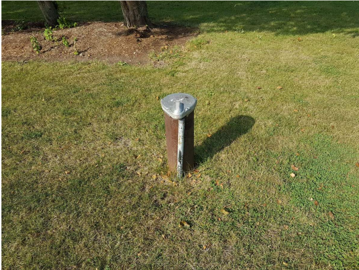
Figure 5-1 On-Site Potable Water Well Location
