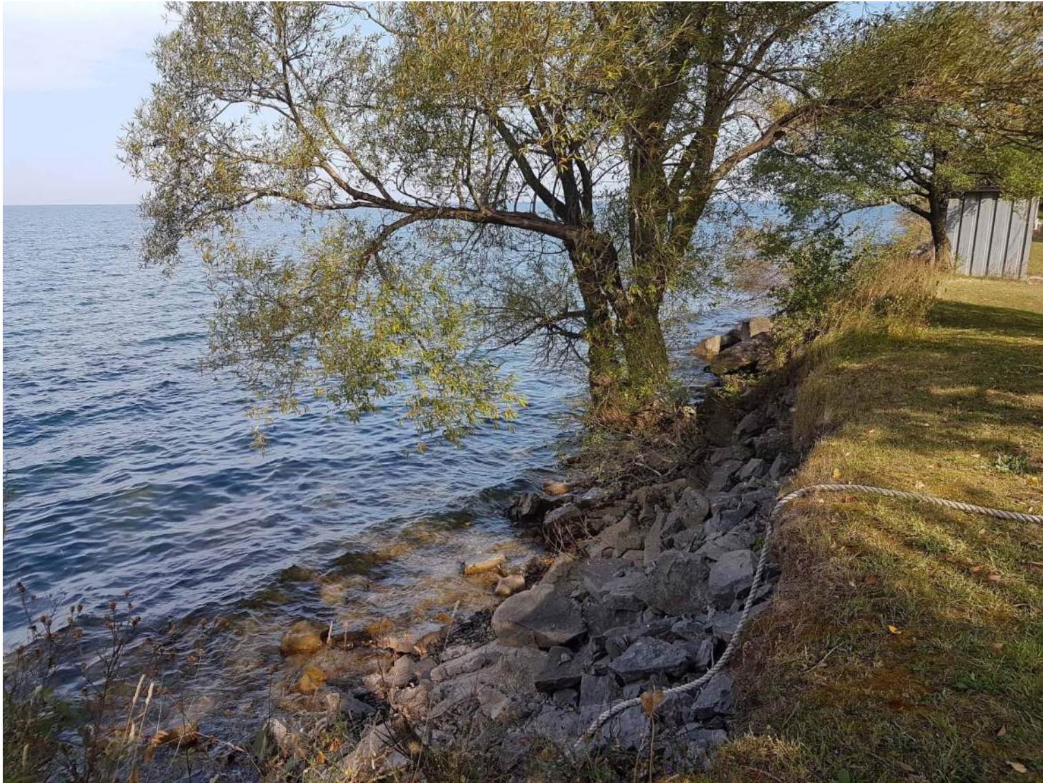
Figure 5-2 Evidence of Erosion
