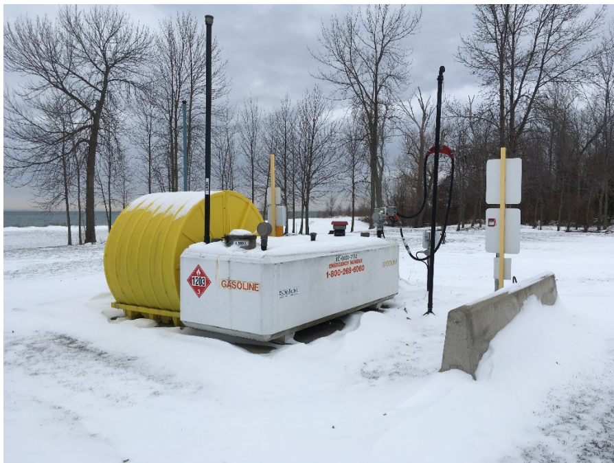
Photograph 8: Gasoline AST (1,900 L), waste oil AST (500 L) and bilge water drums located to the west of storage shed # 1.
