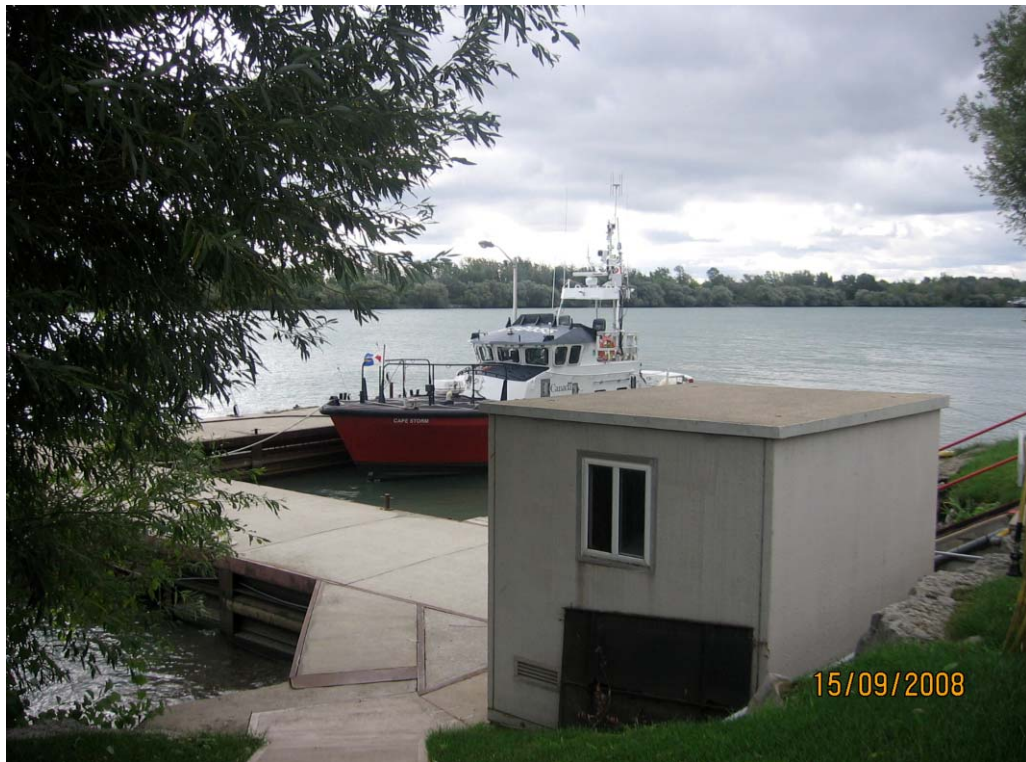
Photograph 4: View of Ready building and dock.
