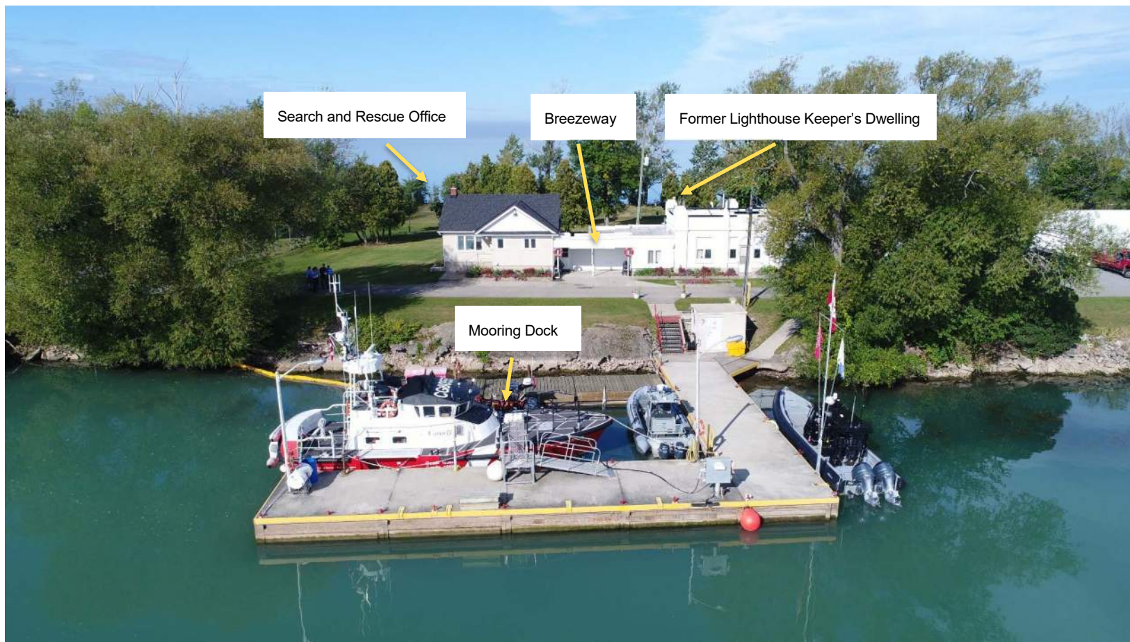
Figure 3-2 Main On-Site Structure and Adjacent Dock
