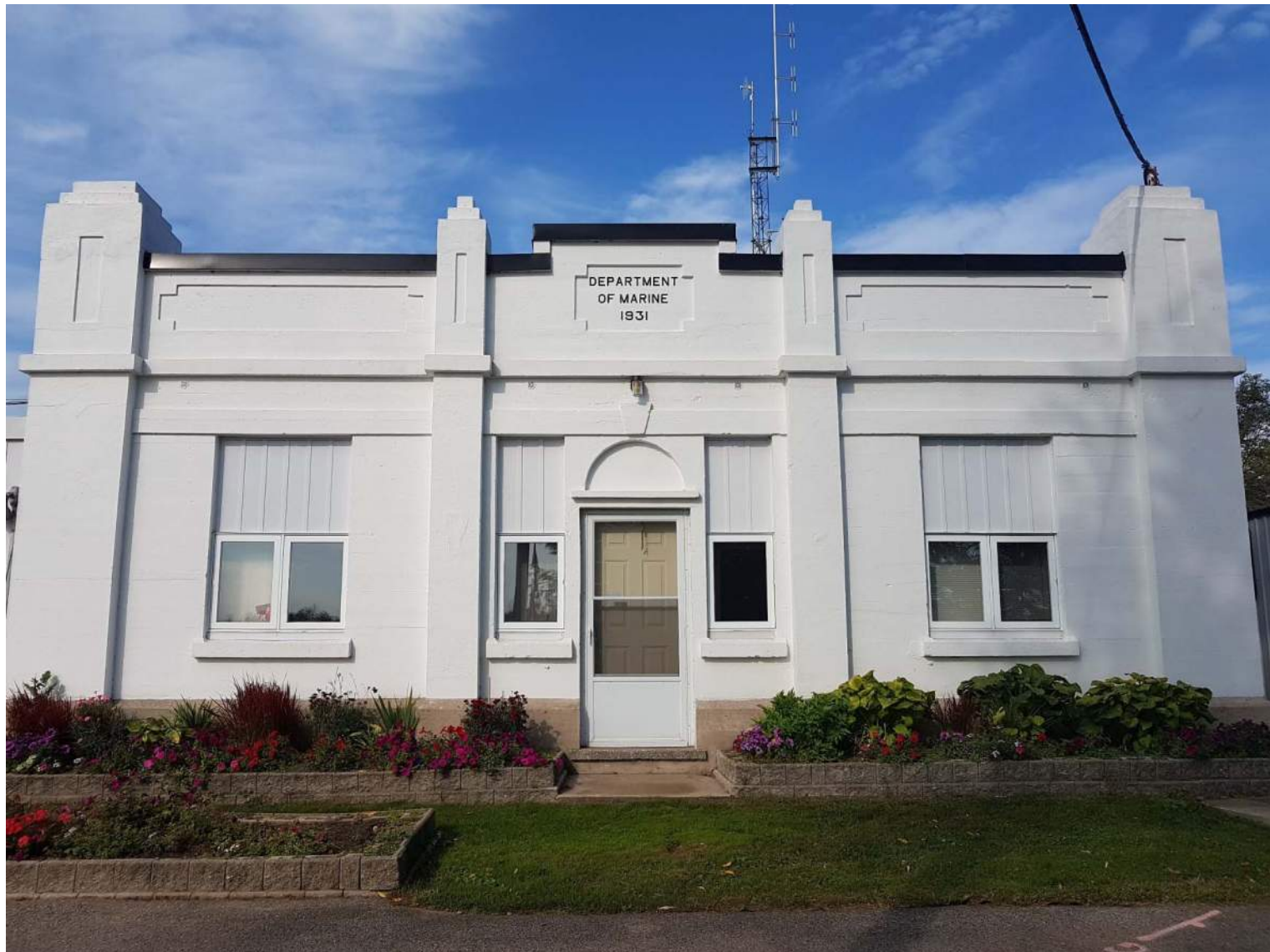
Figure 3-3 Former Lighthouse Keeper's Dwelling
