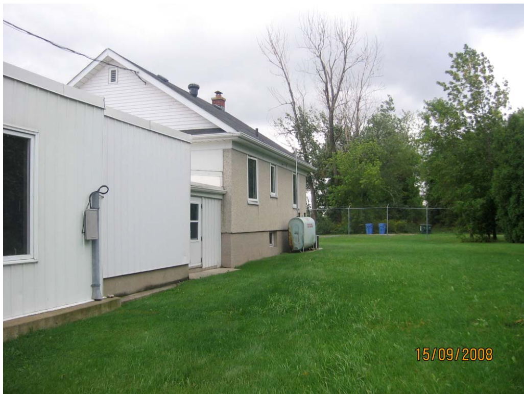
Photograph 10: 1,100-L fuel oil AST on west side of office/residence building.
