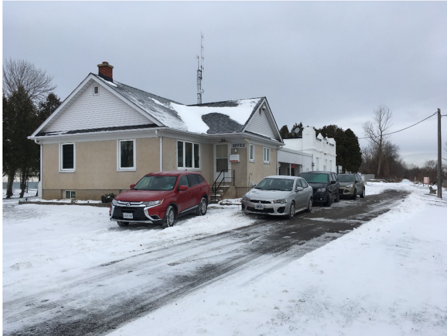
Photograph 1: Main building as viewed from the southwestern portion of the Site.
