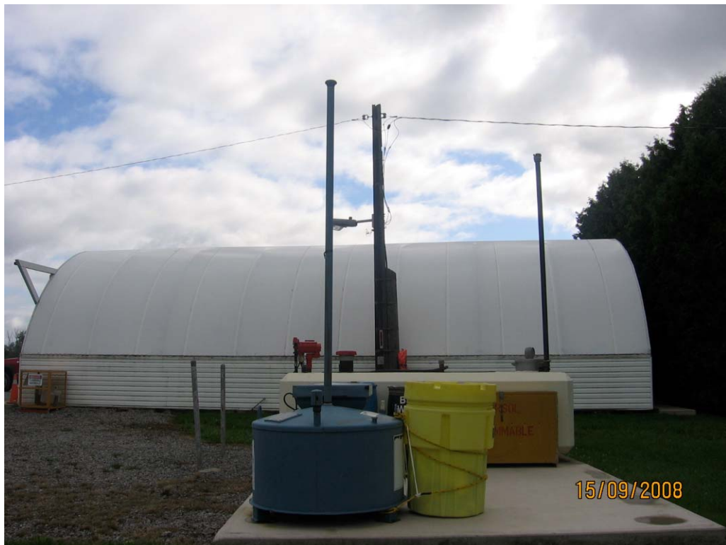
Photograph 13: View of 1,900-L gasoline AST and 500-L waste oil AST.
