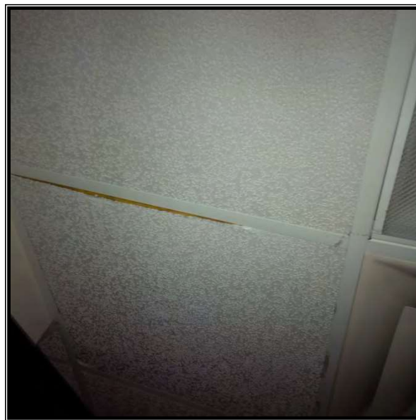
Photo 4 Non-asbestos 24" x 24" lay-in fibreglass ceiling tiles, Exercise Room, Galley House
