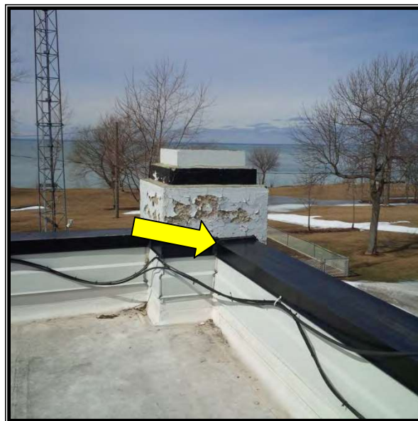
Photo 10 Non-asbestos black caulking at parapets (samples 0008A-C), Roof, Galley House
