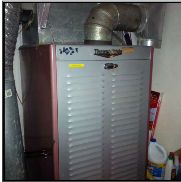
Photo 3 Uninsulated furnace, Furnace Room, Galley House
