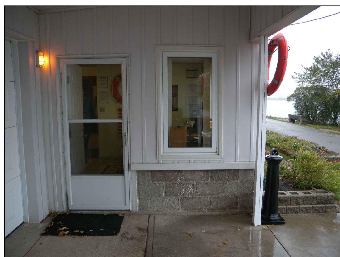
FIG. 11 - EX. ENTRANCE - ENTIRE BUILDING TO BE DEMOLISHED
