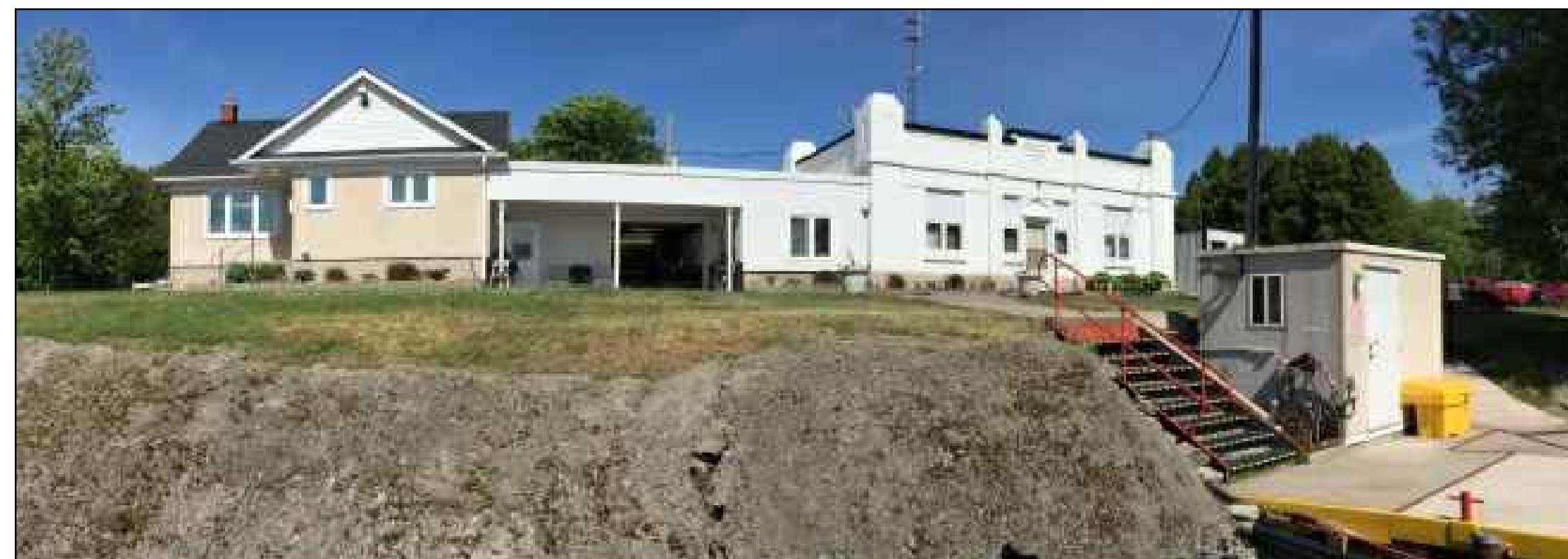
FIG. 2 - EX. BUILDINGS AS SEEN FROM EAST AT DFO DOCK
