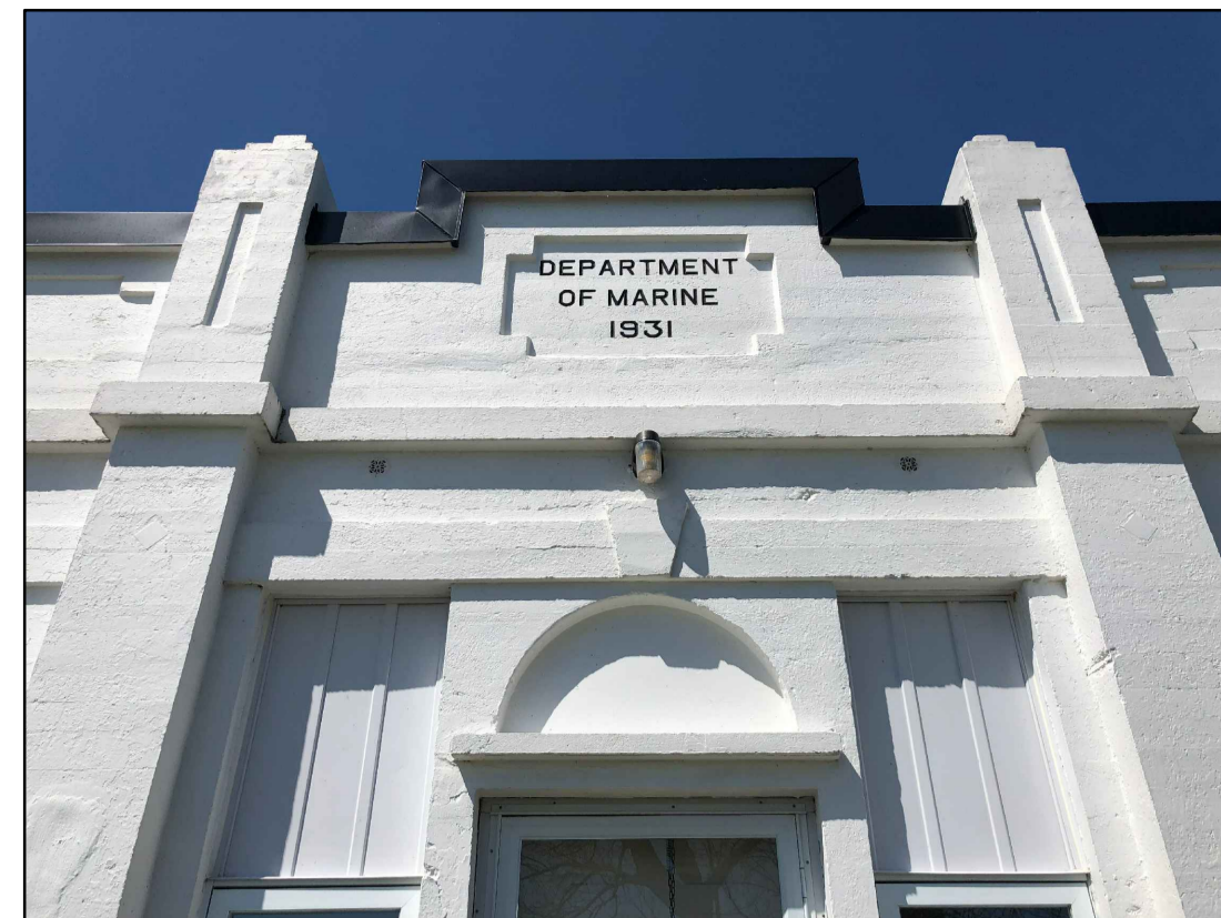
FIG. 2 - HISTORIC BUILDING ENTRANCE DETAIL - EAST ELEVATION
