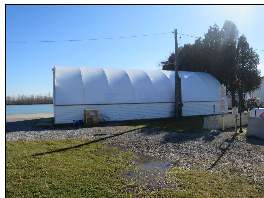
FIG. 9 - EX. EXTERIOR OF HOOP HOUSE - TO REMAIN
