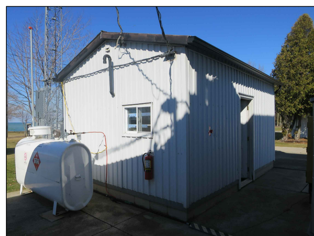
FIG. 13 - EX. EXTERIOR - ENTIRE STRUCTURE TO BE DEMOLISHED
