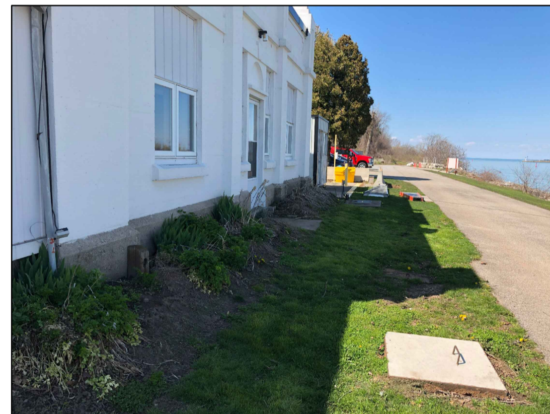
FIG. 9 - EX. SEPTIC TANK IN FRONT OF EAST ELEVATION OF HISTORIC BUILDING - TO BE DECOMMISSIONED, REMOVED AND AREA TO BE RELANDSCAPED WITH SOD
