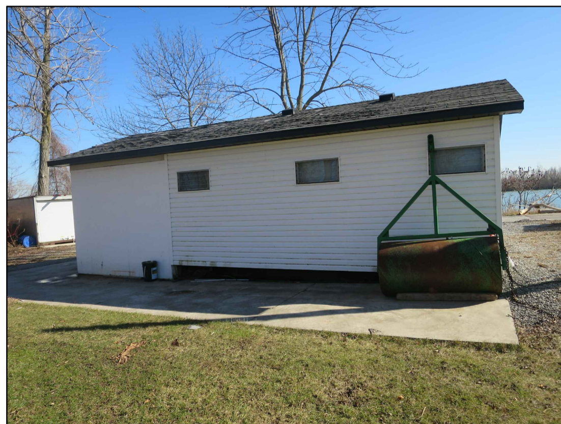
FIG. 13 - EX. EXTERIOR - ENTIRE STRUCTURE TO BE DEMOLISHED
