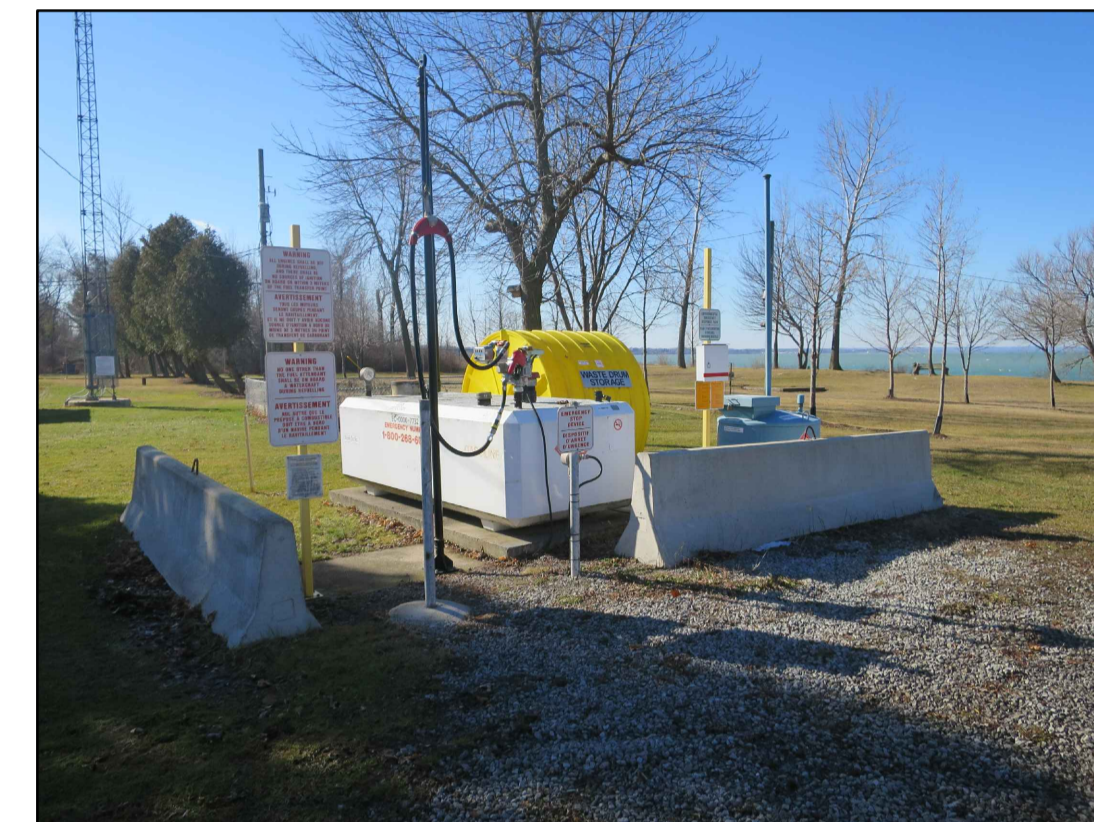
FIG. 6 - EX. DIESEL TANKS. PROTECT IN PLACE AND MAINTAIN ACCESS THROUGHOUT CONSTRUCTION.
