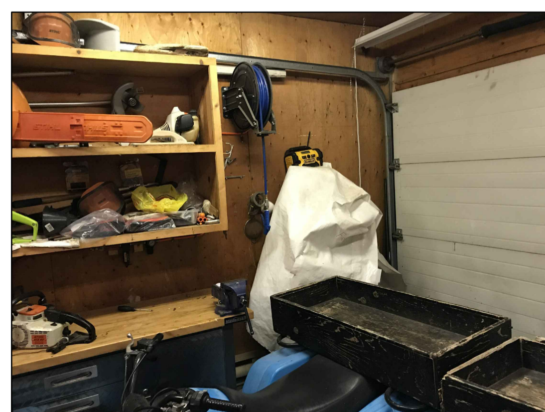
FIG. 14 - EX. INTERIOR - ENTIRE STRUCTURE TO BE DEMOLISHED; CONTENTS WILL BE REMOVED BY OWNER.
