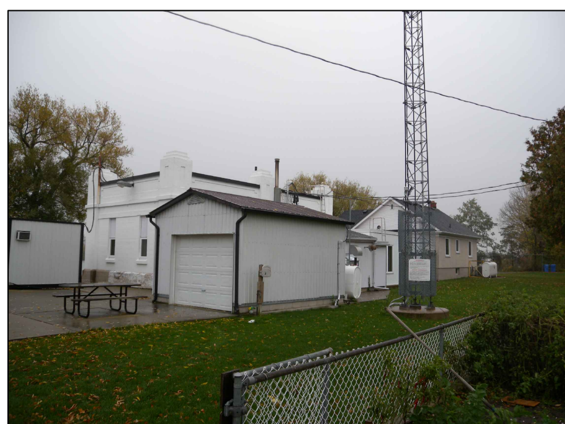
FIG. 12 - EX. EXTERIOR - ENTIRE STRUCTURE TO BE DEMOLISHED
