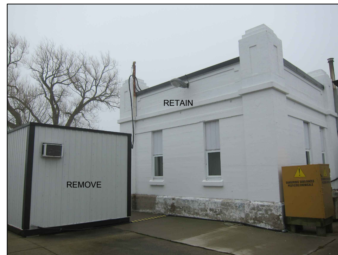
FIG. 3 - HISTORIC BUILDING NORTH ELEVATION
