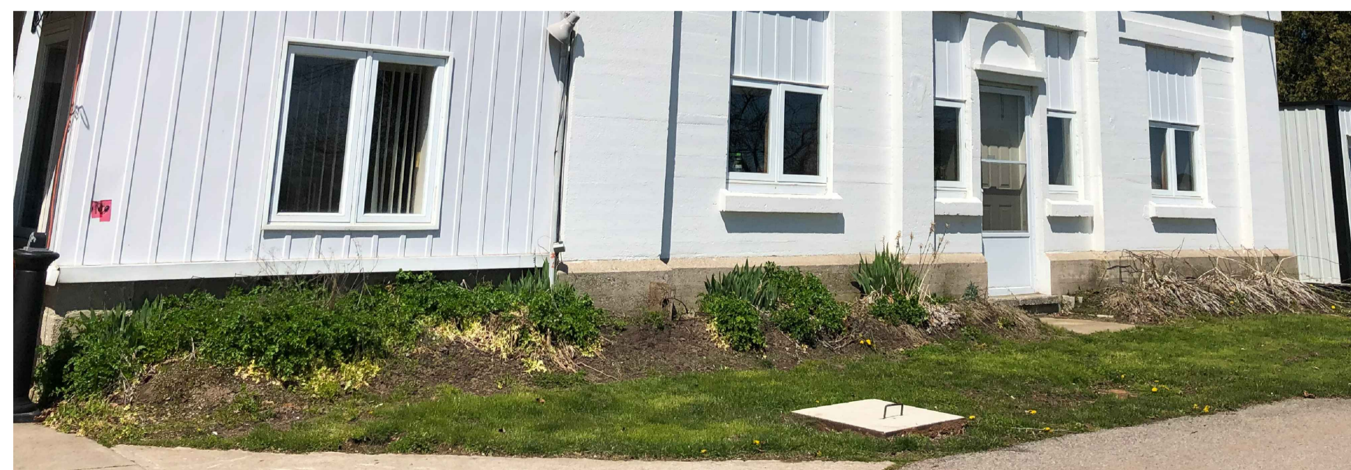
FIG 1 - EX. EAST ELEVATION OF EX. HISTORIC BUILDING (NEW OFFICE)
