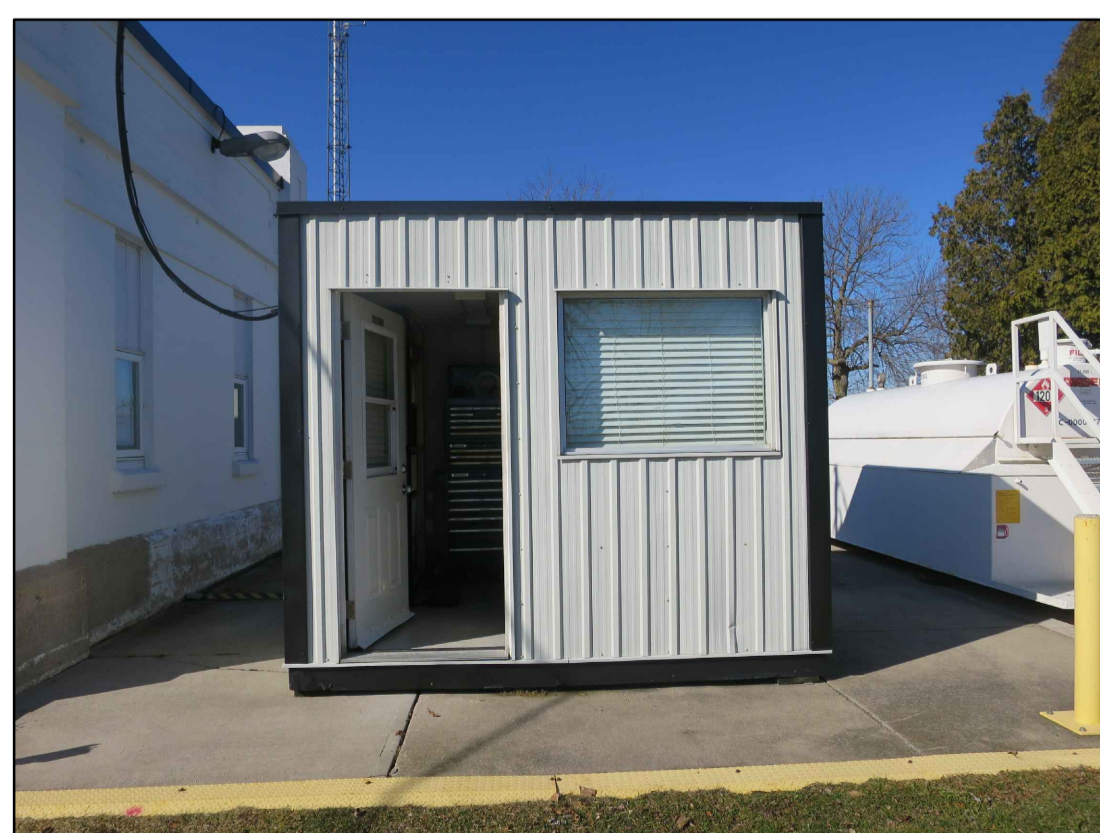
FIG. 15 - EX. EXTERIOR - ENTIRE STRUCTURE TO BE DEMOLISHED
