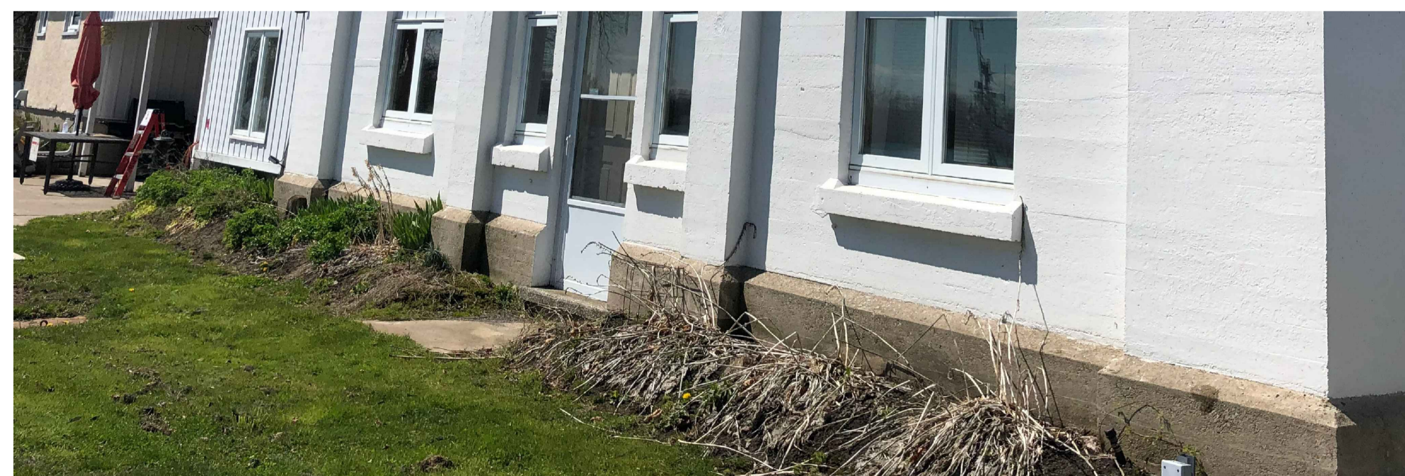
FIG 2 - EX. EAST ELEVATION OF EX. HISTORIC BUILDING (NEW OFFICE)
