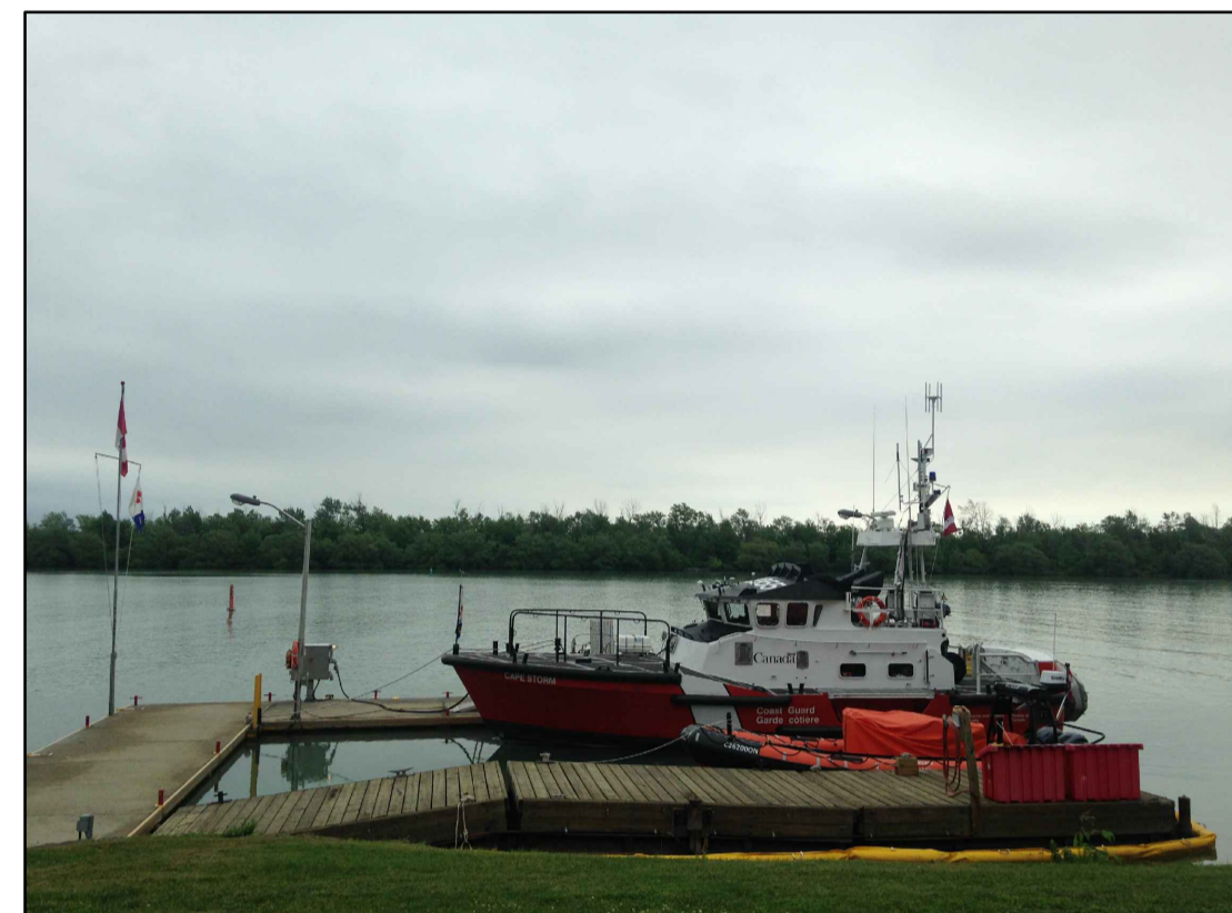
FIG. 3 - EX. DOCK, DEPARTMENT OF FISHERIES & OCEANS DFO. ACCESS TO BE MAINTAINED DURING CONSTRUCTION
