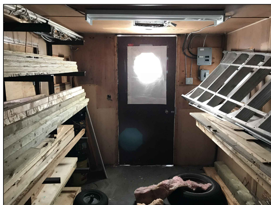
FIG. 14 - EX. INTERIOR - ENTIRE STRUCTURE TO BE DEMOLISHED (OWNER WILL REMOVE MATERIALS).
