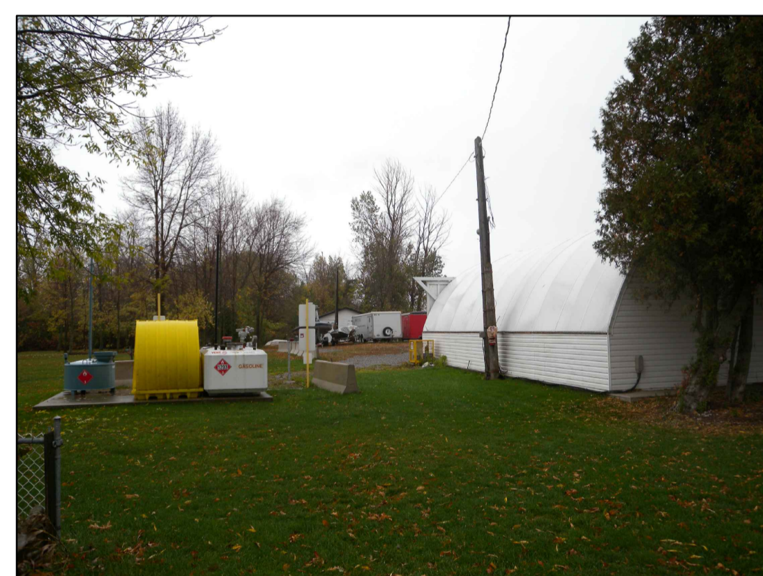
FIG. 10 - EX. EXTERIOR OF HOOP HOUSE - TO REMAIN
