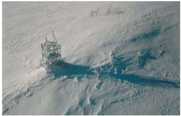
Figure #12: Mount Arthur microwave repeater site (1997)
