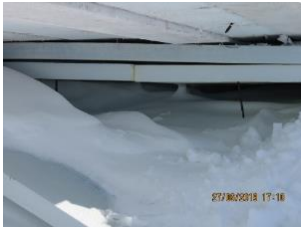
Figure #40: The Styrofoam layers were fastened to the ice layer with 8" spiral steel spikes
