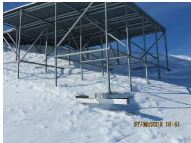
Figure #29: Close up view of South-East section of loading pad
