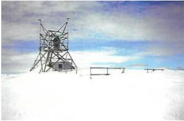
Figure #11: Mount Arthur microwave repeater site with antennas removed (October 1994)
