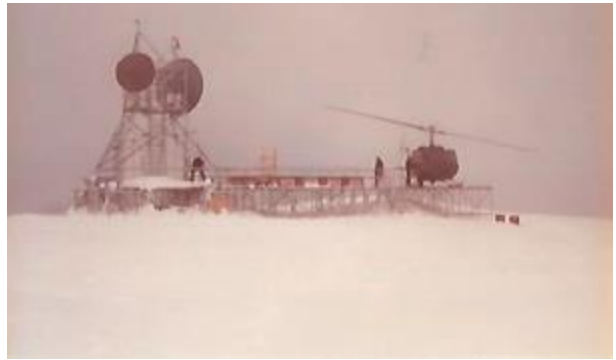
Figure #6: Mount Arthur microwave repeater site (1982)
