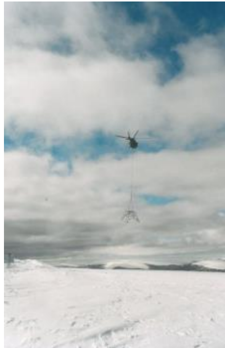
Figure #13: Mount Arthur- antenna tower removed from site (1997)
