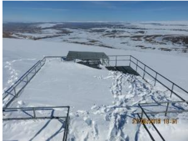
Figure #25: View looking east – battery platform in foreground and loading area in background
