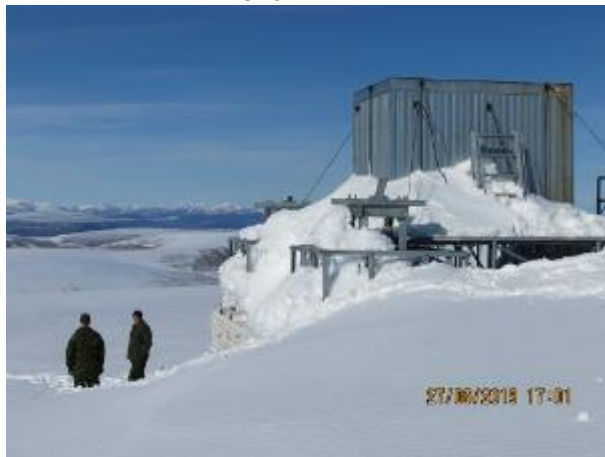
Figure #20: View of equipment shelter area of platform
