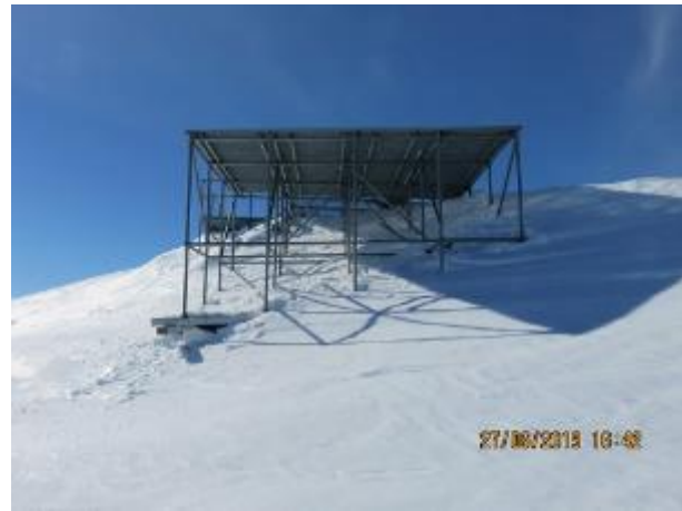
Figure #19: View of platform looking west
