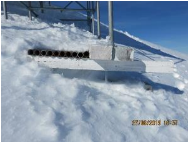
Figure #30: Close up view of South-East section of loading pad
