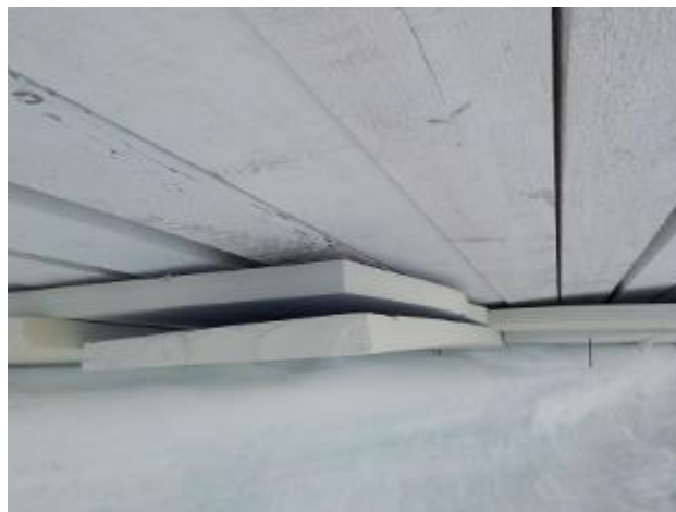
Figure #66: Styrofoam insulation
