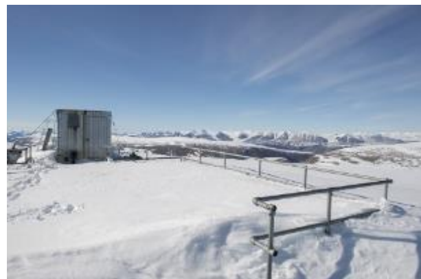
Figure #23: View of abandoned equipment shelter on platform
