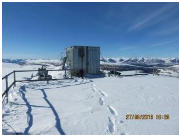
Figure #22: View of abandoned equipment shelter on platform
