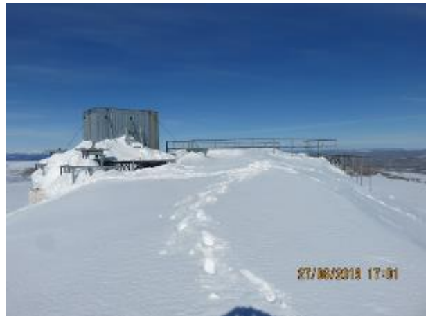
Figure #17: View of existing platform looking north
