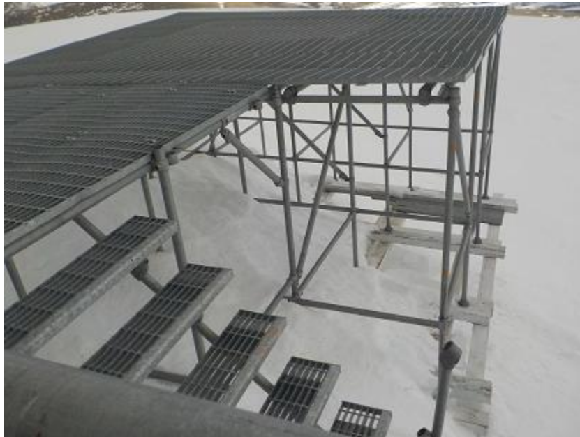
Figure #76: Steel stairs
