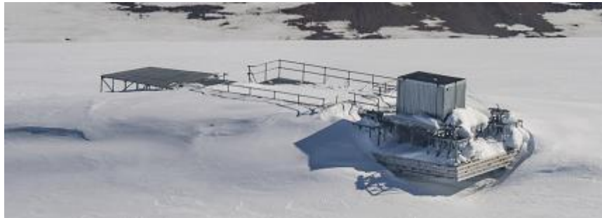
Figure #71: Safety railing
