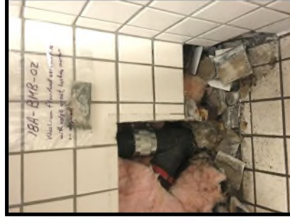
Locker Room Floor & Wall Tiling Materials 3" Ceramic Tile; Edging Grout; and Backing Mortar Sample 18A-BMB-02 layers were 'None Detected' for asbestos.
