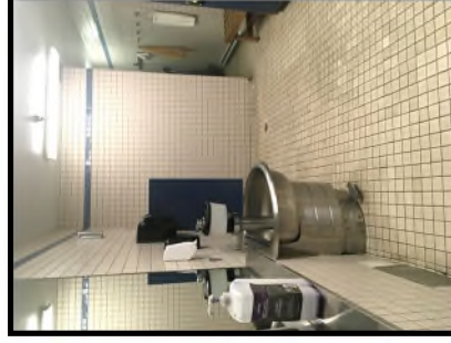
Locker Room Floor & Wall Tiling Materials 3" Ceramic Tile; Edging Grout; and Backing Mortar Sample 18A-BMB-02 layers were 'None Detected' for asbestos.
