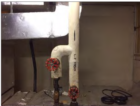
Asbestos containing parging cement pipe fittings (Samples 0004A-C) and non-asbestos fibreglass insulation (Samples 0003A-C) present in Boiler Room 1.
