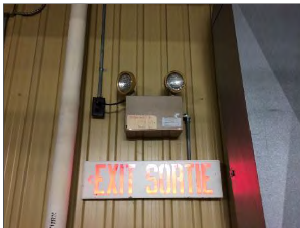
Lead acid battery for emergency lighting.
