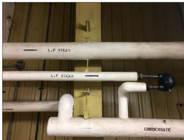
Asbestos containing parging cement pipe fittings (Samples 0002A-C) and non-asbestos fibreglass insulation (Samples 0001A-C) present in Boiler Room 1.
