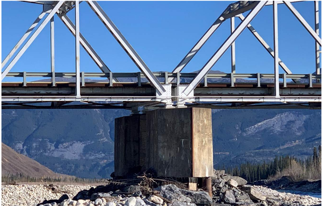
P05 - Existing central pier, looking downstream
