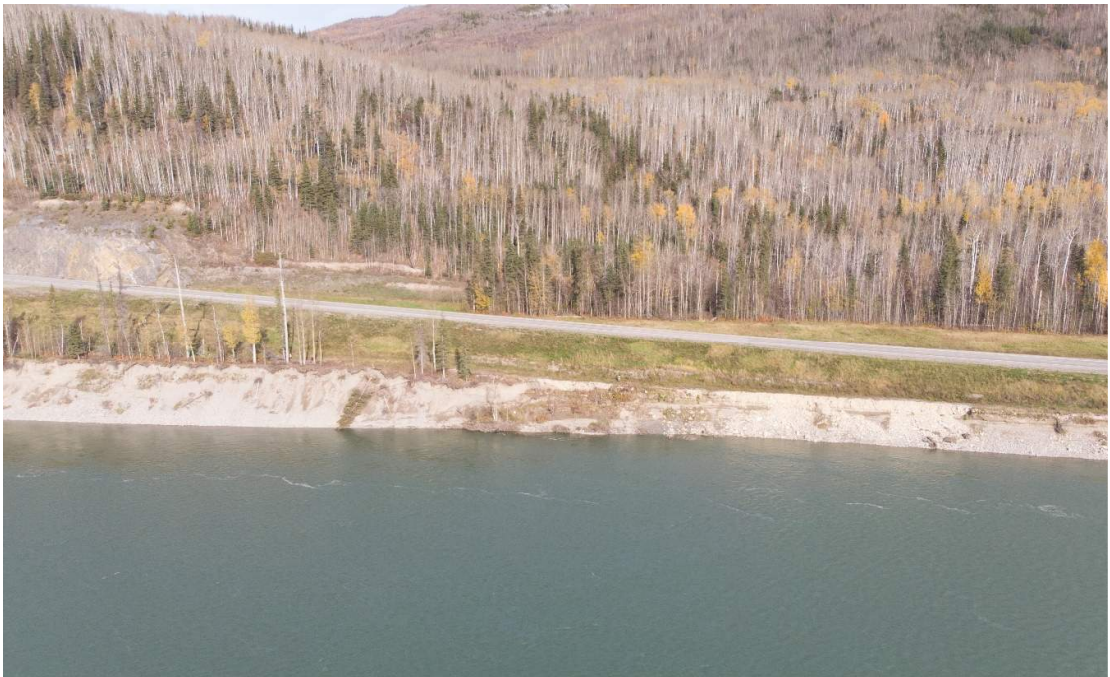
P02 - Zoomed in view of highway embankment 1
