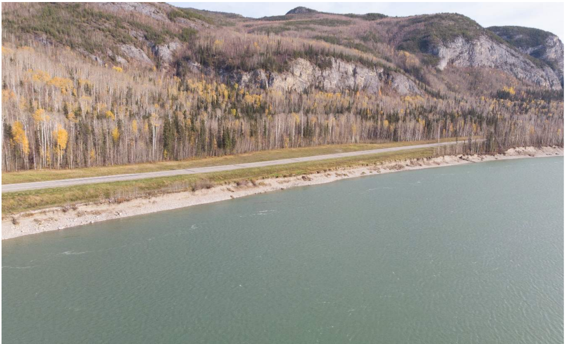
P04 - Zoomed in view of highway embankment 3
