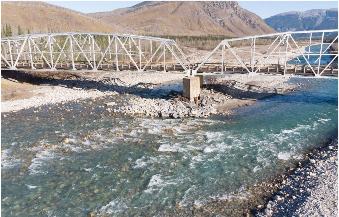
P02 - Looking downstream, square to bridge, taken from air 2
