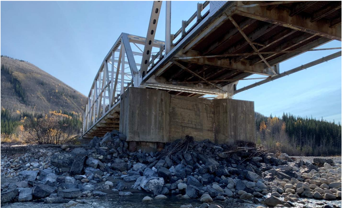
P11 - Side view of existing pier (looking towards Fort Nelson) 3
