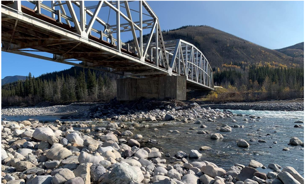
P09 - Side view of existing pier (looking towards Fort Nelson) 1
