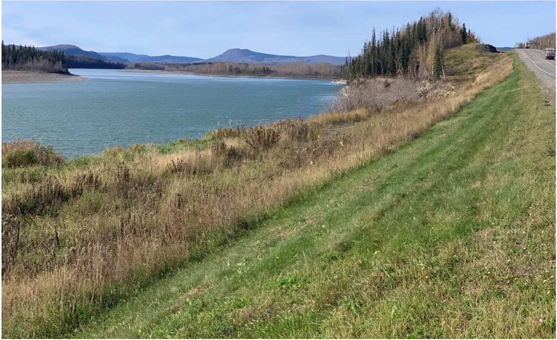
P07 - Existing vegetation on highway embankment, looking upstream
