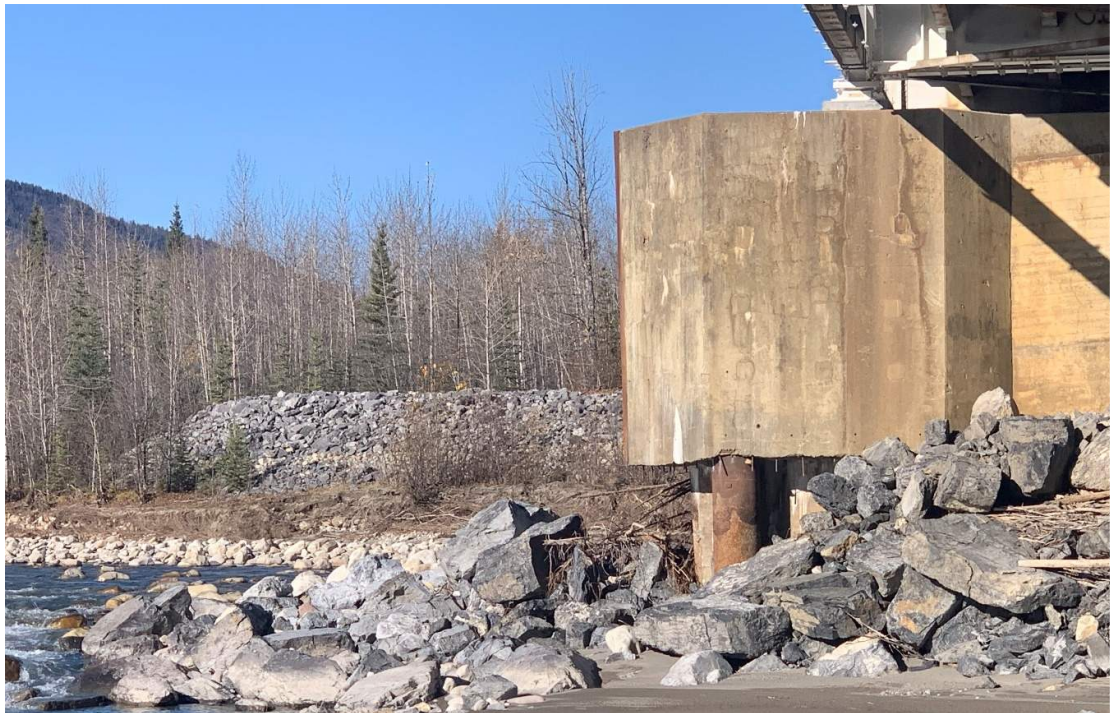
P06 - Side view of existing pier nose (looking towards Watson Lake)
