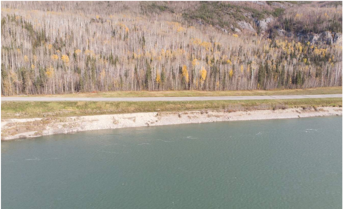
P03 - Zoomed in view of highway embankment 2
