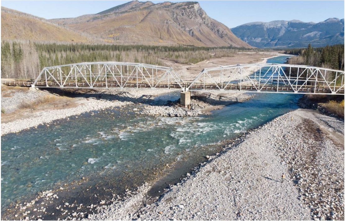
P01 - Looking downstream, square to bridge, taken from air 1
