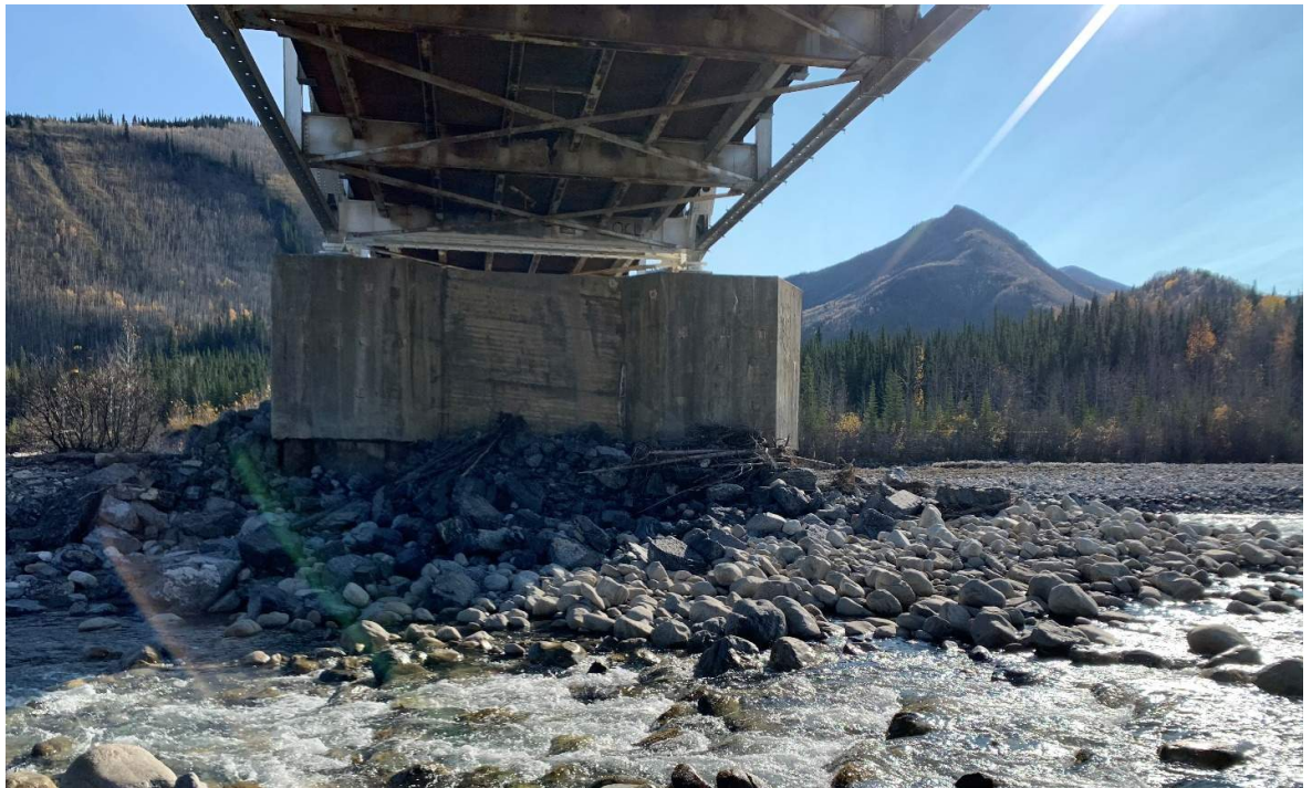
P10 - Side view of existing pier (looking towards Fort Nelson) 2
