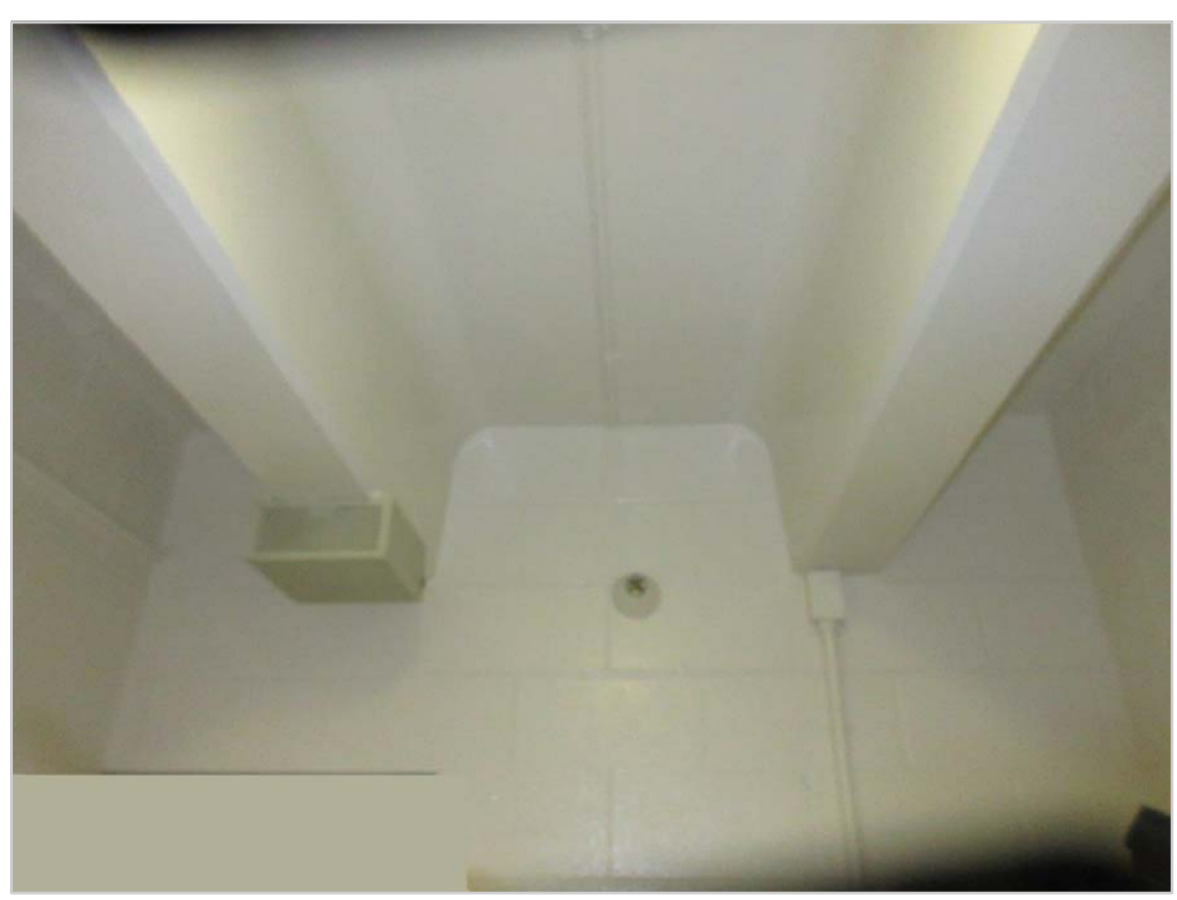
07: TYPICAL CELL CONDITION, ABOVE DOOR
