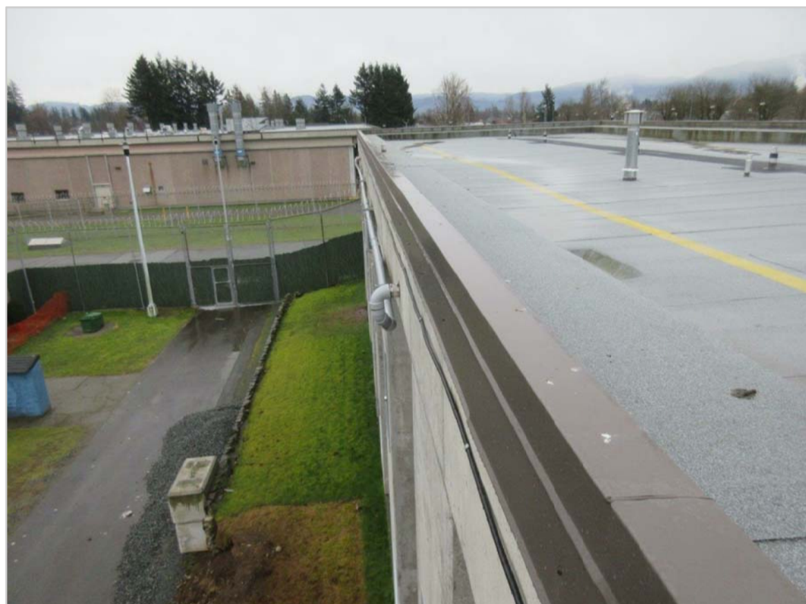
03: NORTH PARAPET AND RAIN WATER LEADER
