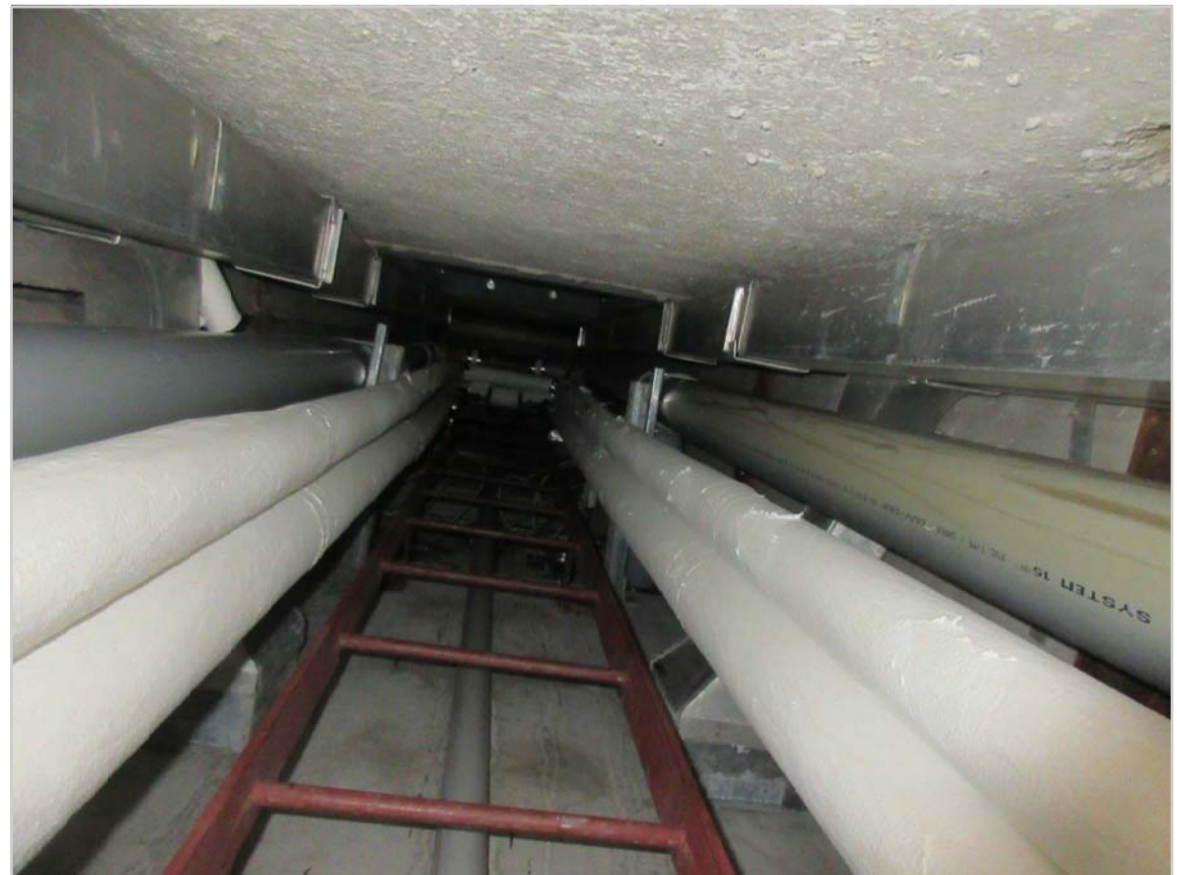
12: TYPICAL CONDITION INSIDE EXTERIOR CHASE, TOWARDS THE TOP
