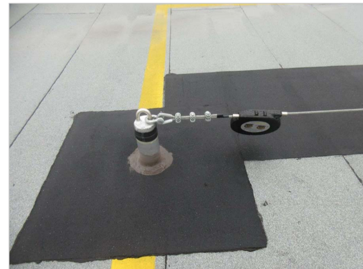
06: END ROOF ANCHOR WITH SHOCK ABSORBER
