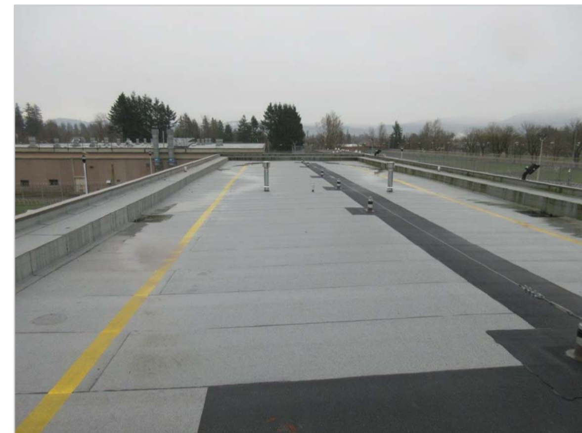
02: ROOF, VIEWED FROM WEST
