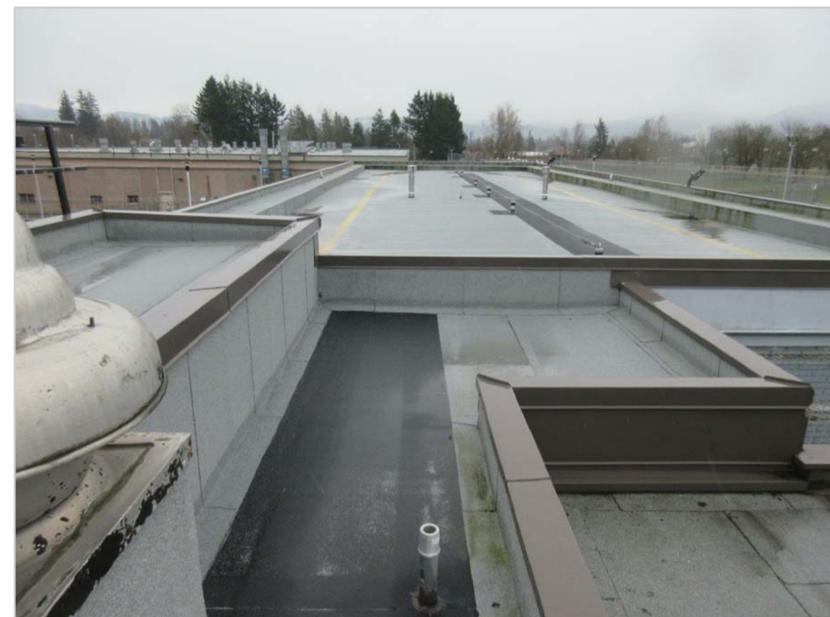
01: VIEW FROM WEST ADJACENT ROOF
