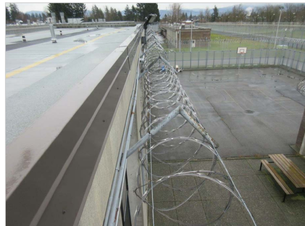
05: SOUTH PARAPET WITH CONCERTINA TAPE
