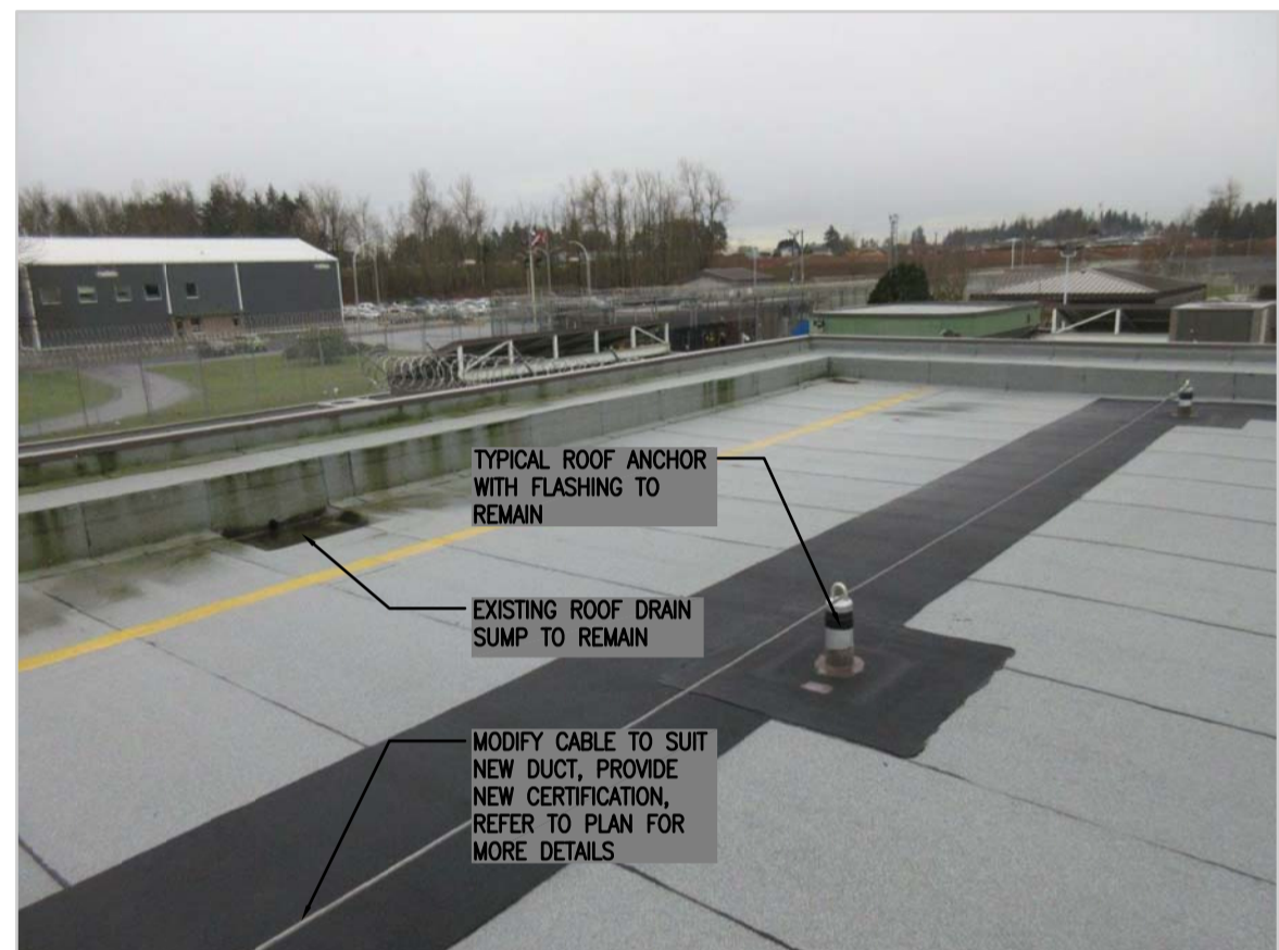
04: ROOF, NORTH EAST CORNER
