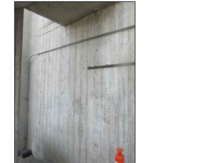
#20 - LU5 - KITCHEN WALL OUTSIDE
