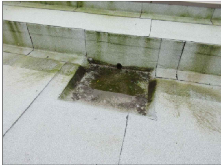
#6 LU5 - ROOF DRAIN
