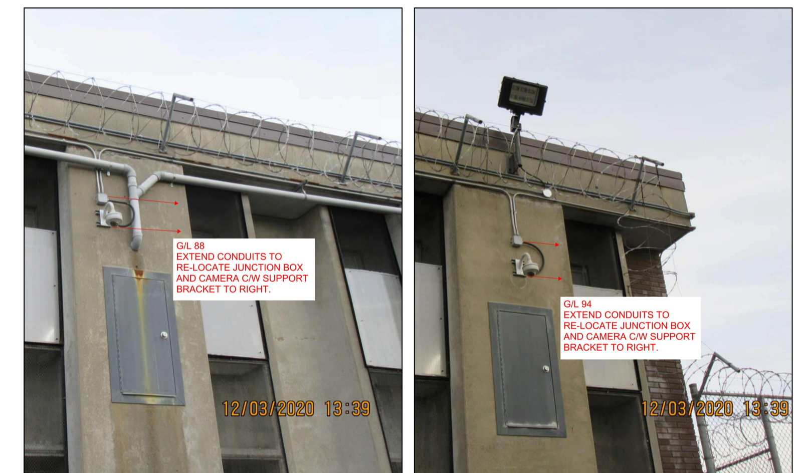
EXTERNAL VIDEO CAMERA RELOCATIONS
