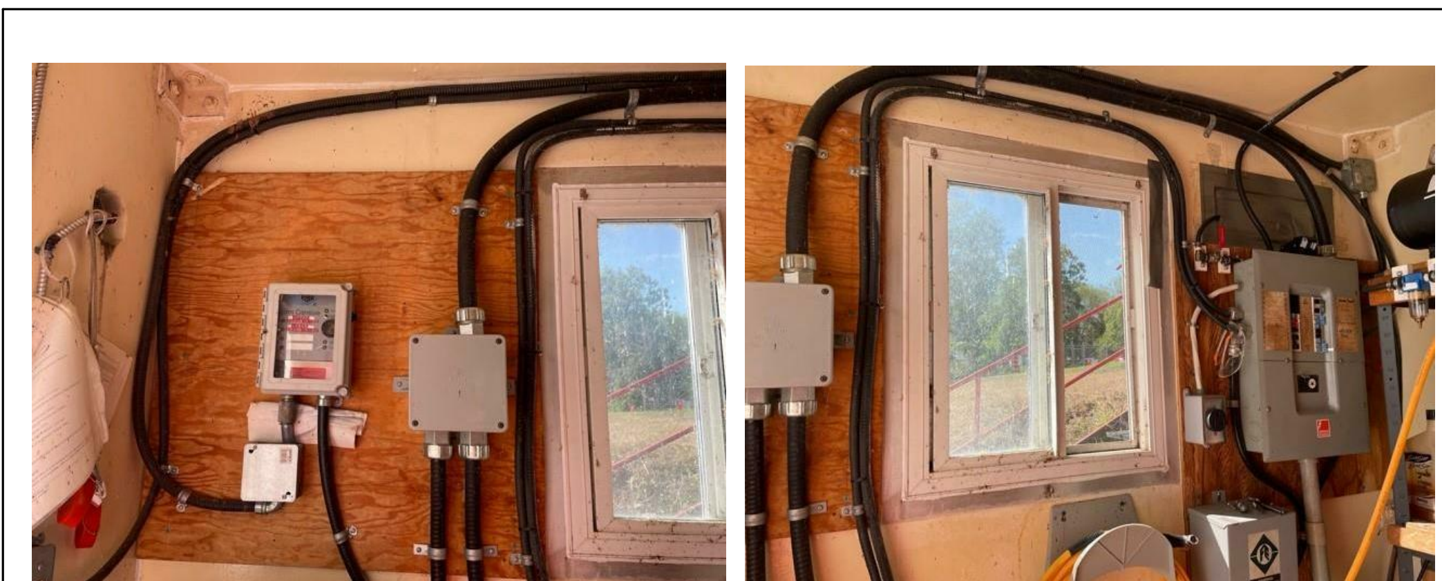
4 NEW LOCAL SHORE POWER DISTRIBUTION "PP-2SP" E901 N.T.S.
