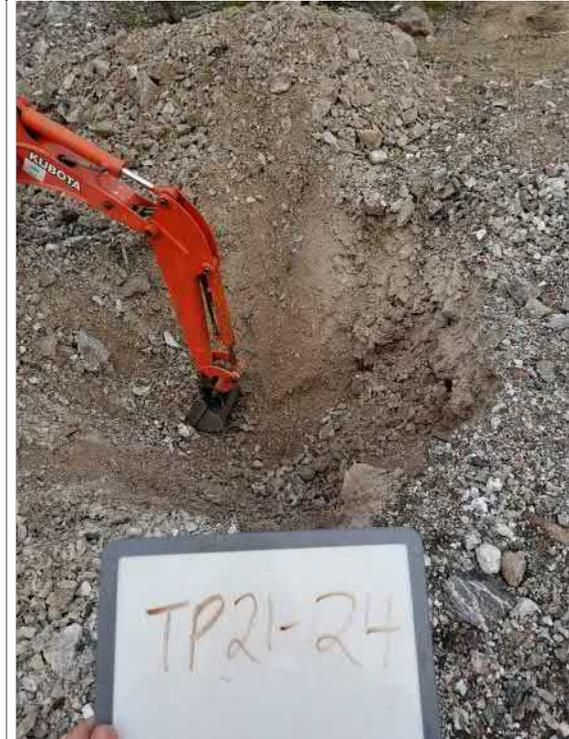
Photo 46: Excavated TP21-24 until contact with rock surface prevented the machine from continuing deeper. 1.05 metres below ground surface (mbgs) was reached.
