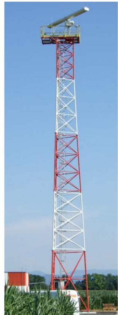
Figure 7.1 Three-legged lattice tower
