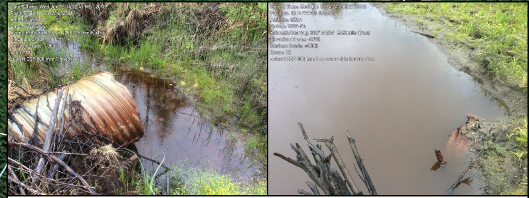
Culvert 13+200: Inlet (left) and Outlet (right)
