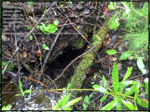
Culvert 22+070: Two views of the culvert
