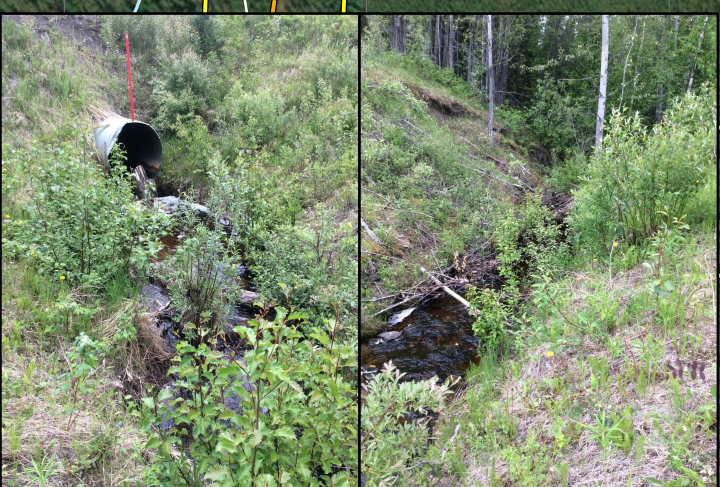
Culvert Ex-10 (SE): 48" Diameter / Downstream side / Boulder and gravel substrate
