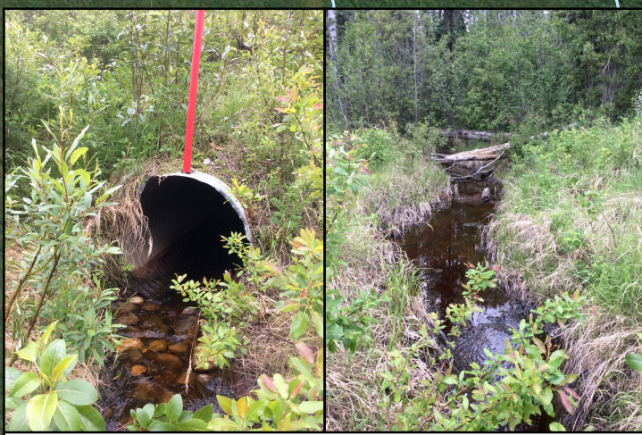
Culvert Ex-11 (NW): 36" Diameter / Upstream side / Gravel substrate
