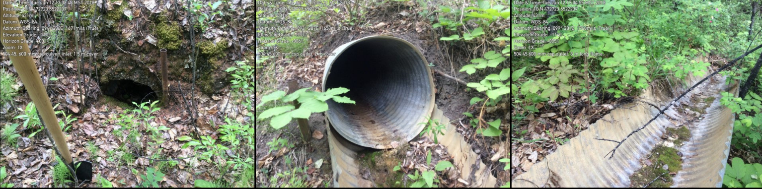
Culvert 22+510: Inlet (left), Outlet (centre) and Flume (right)
