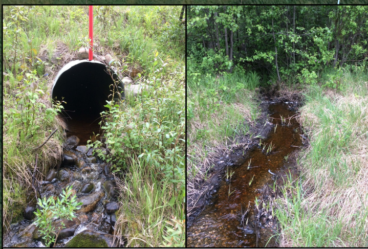
Culvert Ex-11 (SE): 36" Diameter / Downstream side / Gravel substrate
