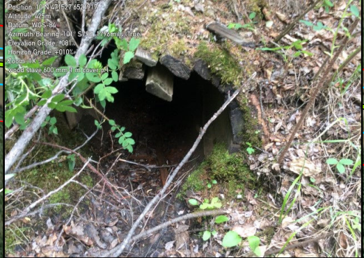
Culvert 23+990: Inlet (top) and Outlet (bottom)
