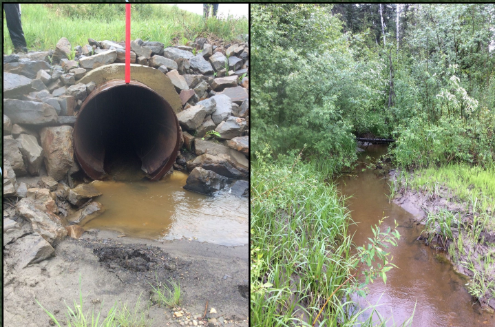
Culvert Ex-4 (NW): 41" Diameter / Upstream side / Gravel, cobble, silt substrate
