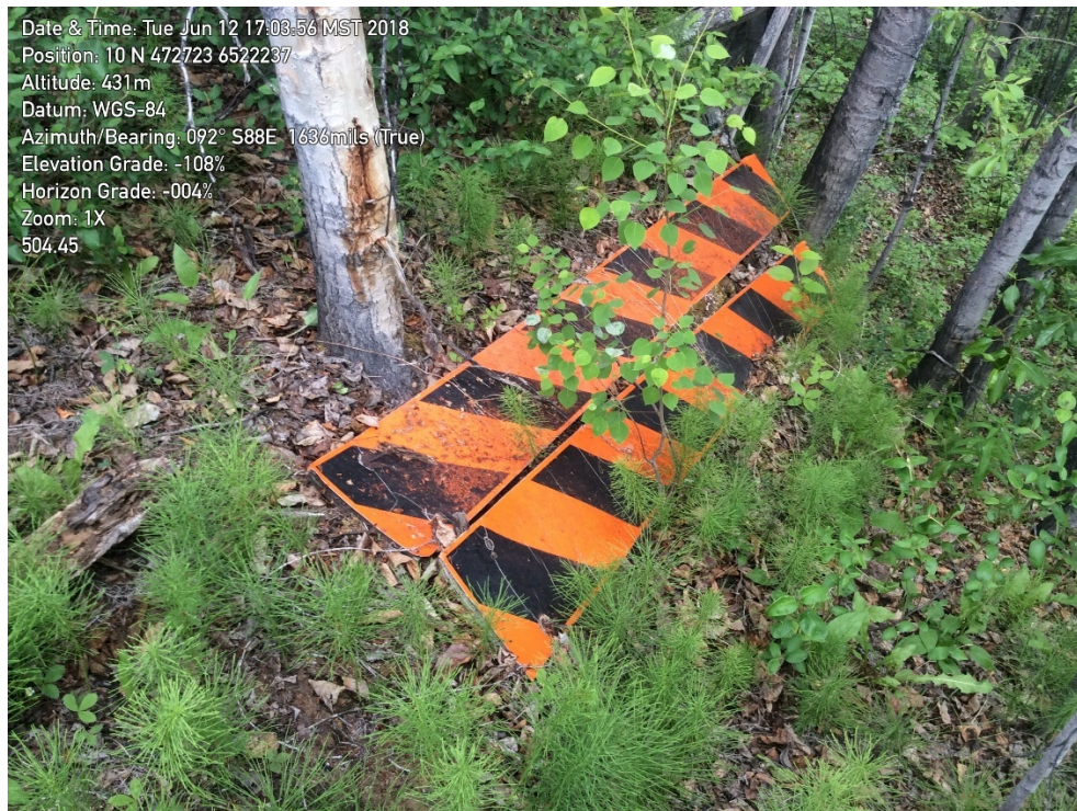
Photo 4: Debris Location C (Approx. Km 22.84) – Photo 1 of 1
