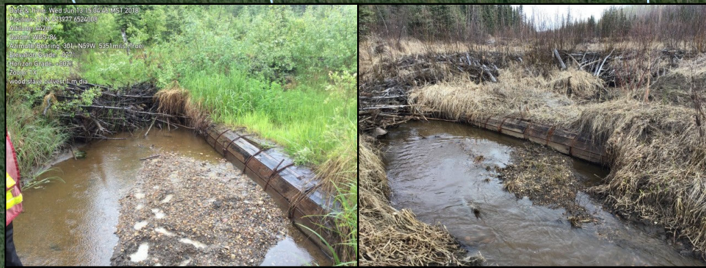
Culvert 14+300: Views of the woodstave
