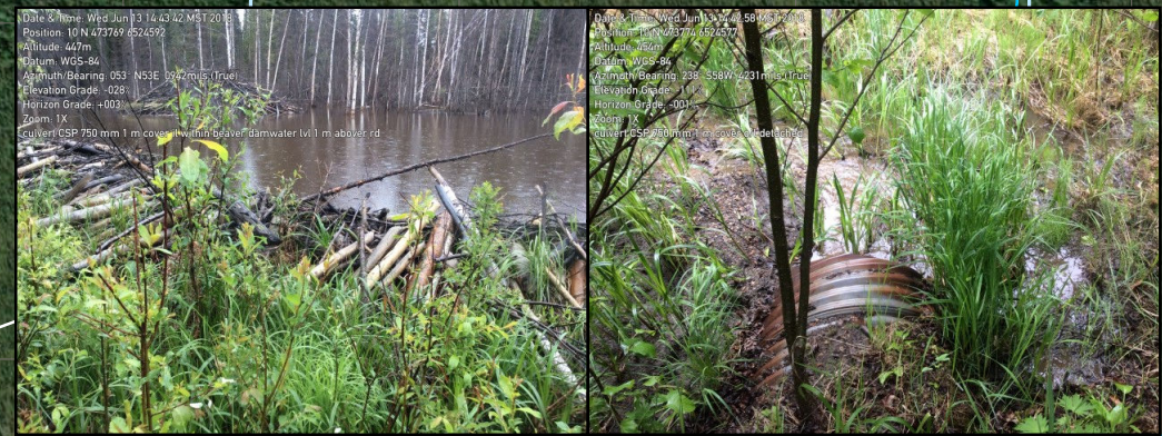
Culvert 13+680: Inlet (left) and Outlet (right)
