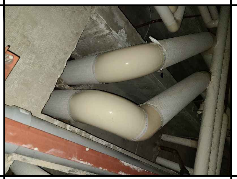
FIGURE A RISERS TO AHU-1
