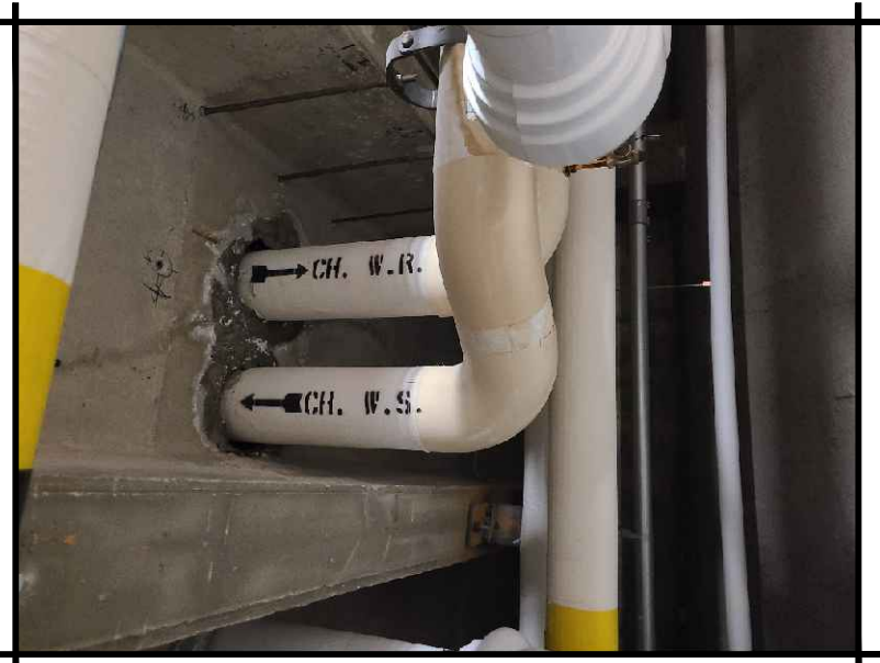
FIGURE C RISERS TO AHU-1
