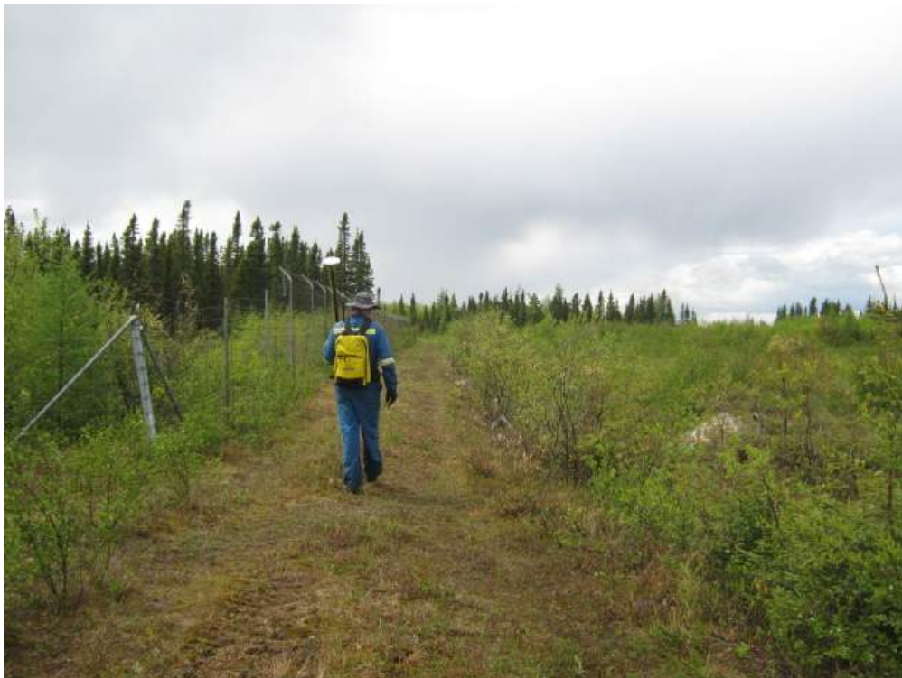
Photo 6 – Perimeter access road along south fence line. Wet/bog areas, light brush and missing BWO (Sta. 3+658).
