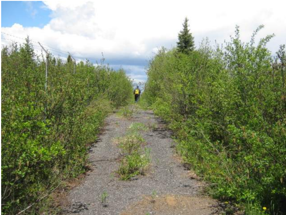
Photo 4 – Heavy brush along northwest perimeter access road (Sta. 0+200).
