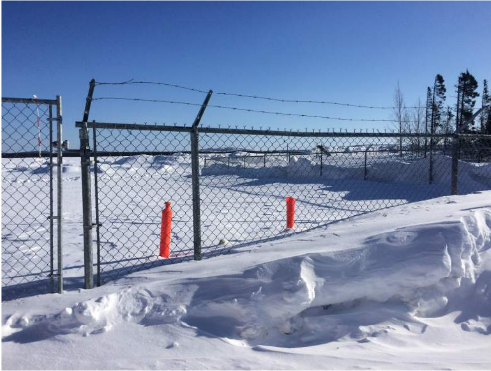
Photo 9 – Chain link fence missing BW strand on south side of Hangar (Sta. 5+400).
