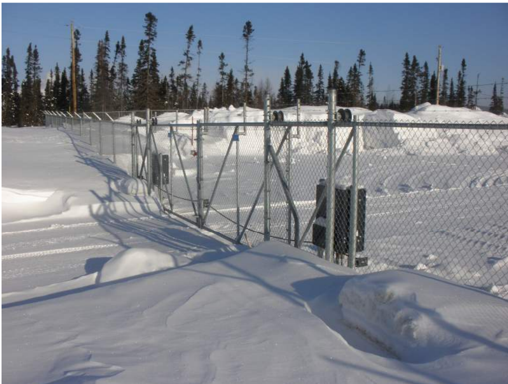
Photo 12 – Automated rolling gate (A2) near the CSB.
