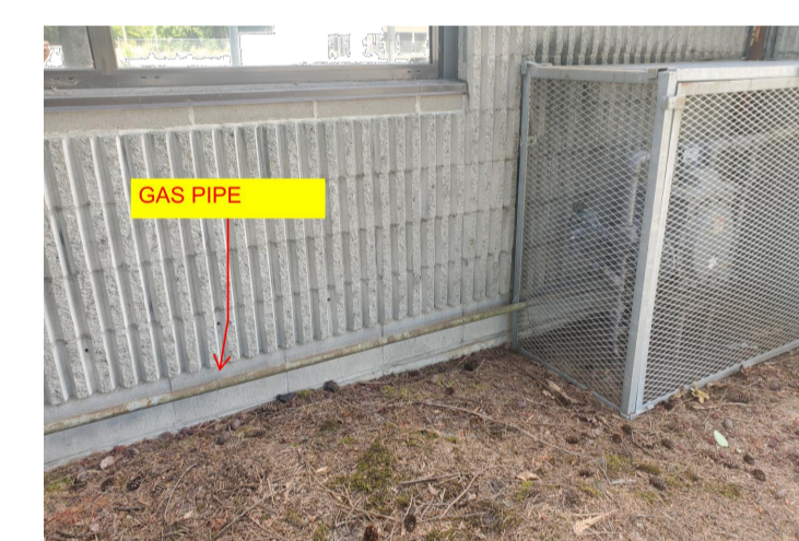
14 EXISTING GENERATOR #2 E2.1 NOT TO SCALE
