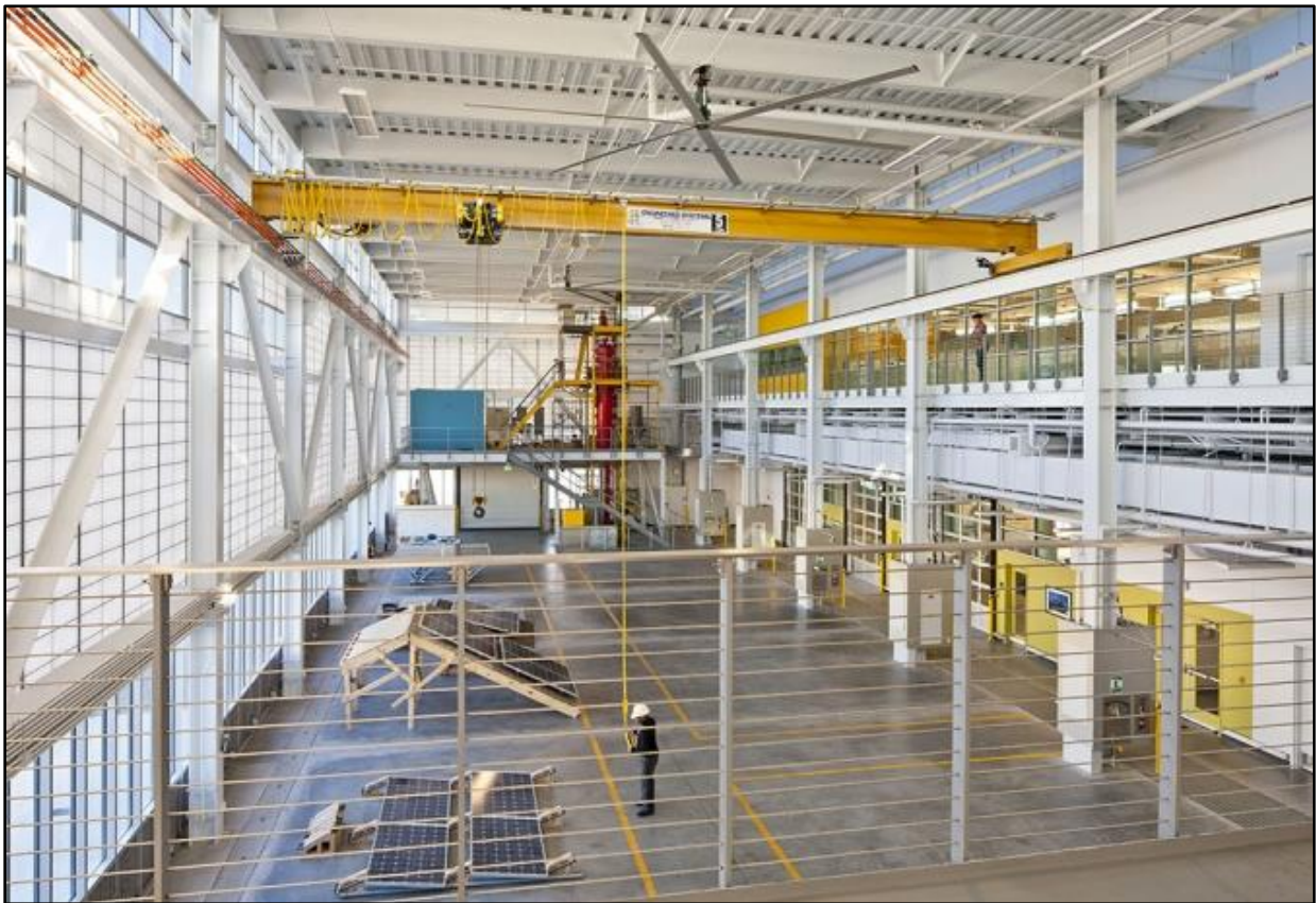
Figure 3.5: Georgia Tech University, Carbon-Neutral Energy Solutions Laboratory (CNES) (Atlanta, GA)
