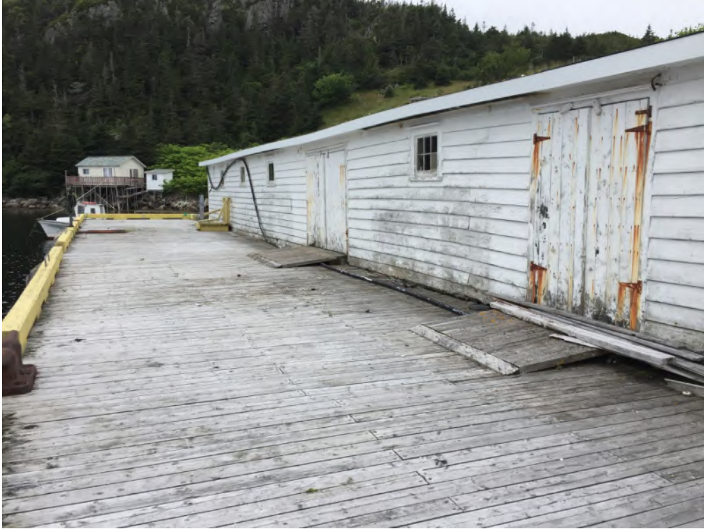
Photo taken prior to September 10, 2021.
