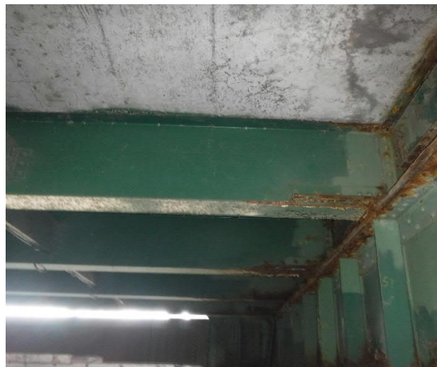
Approach Span at Rear Floor Beam
