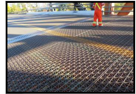
PHOTO - 1 GENERAL VIEW OF GRATING PANEL AT BRIDGE C.L.
