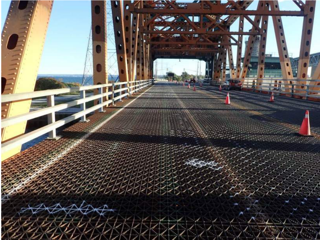
Photo 1: Typical BCLB Grating view with Traffic Control during inspection
