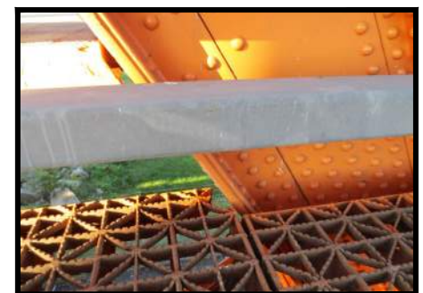
PHOTO - 3 130x50 COPED PANEL CORNER
