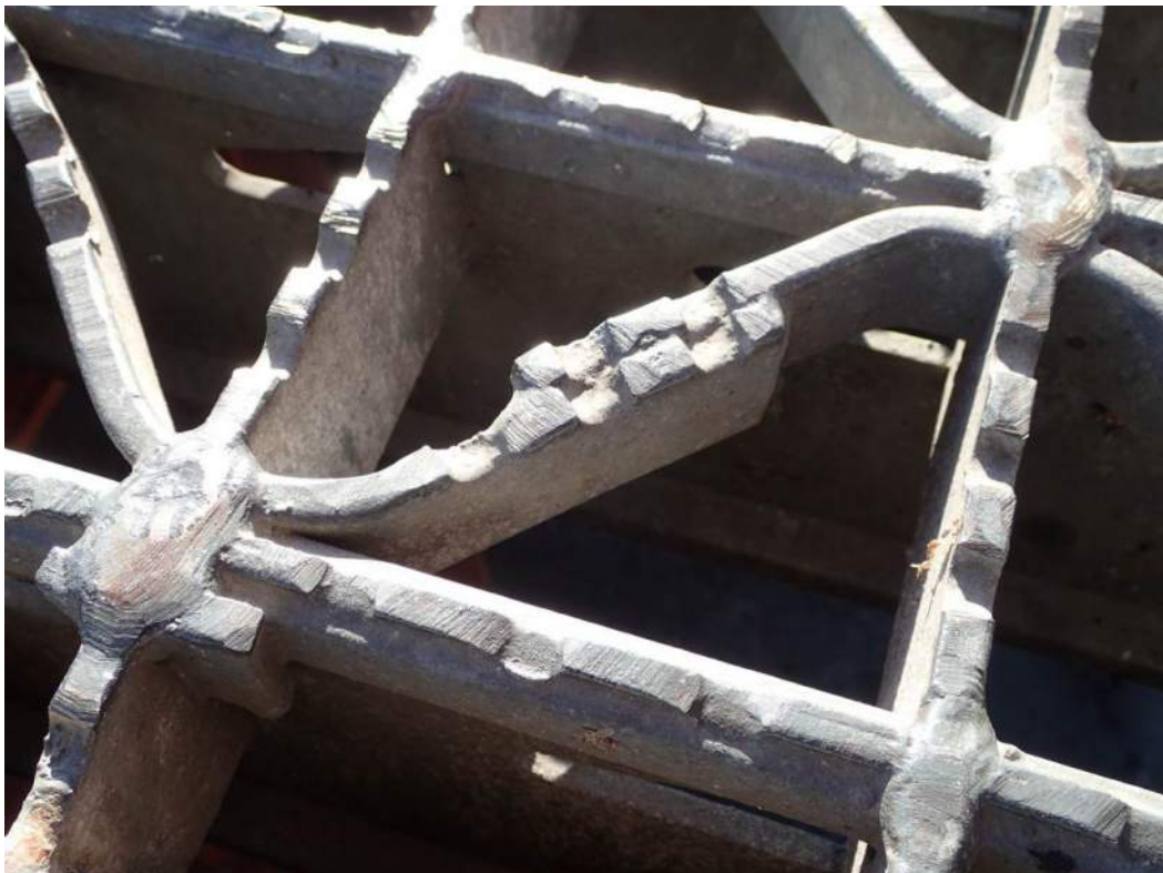
Photo 4: Test Panel detail
