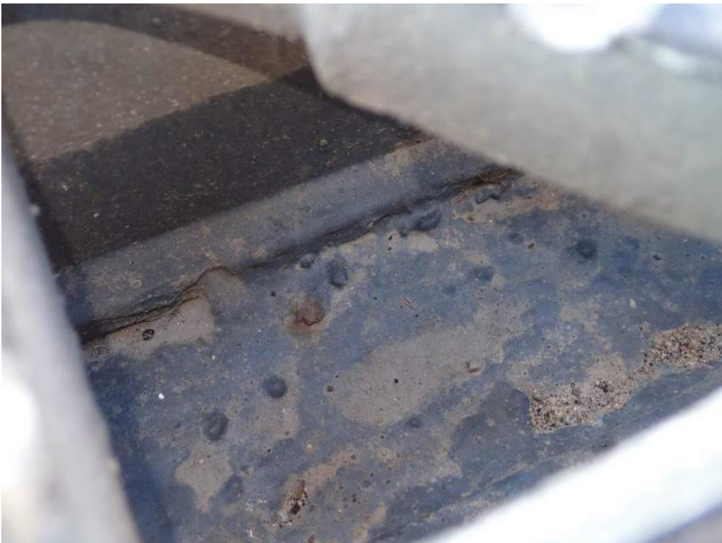
Photo 6: Test Panel – Typical M-beam to stringer connection
