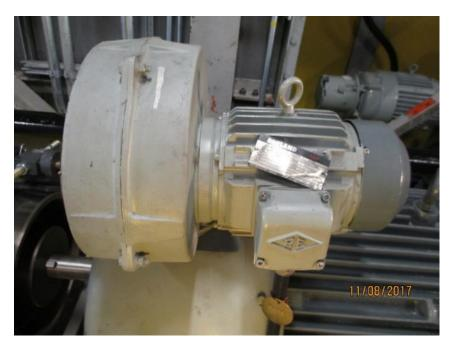
Photo E25 Northeast Motor Blower Nameplate. The blower nameplate was not affixed to the motor at the time of inspection.
