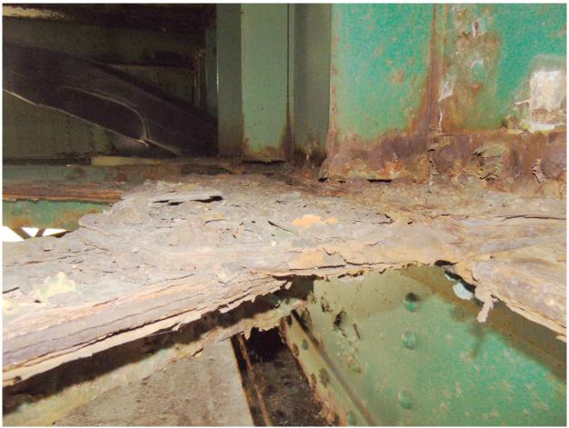
134 Severe Corrosion on Sway Bracing at Rear Floor Beam @ North Tower (TYP)
