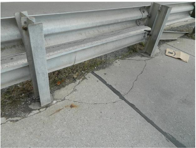
304 Wide Cracks on Sidewalk & Light Impact Damages on Posts @ Southwest Approach Page A2 [152] of A2 [153]
