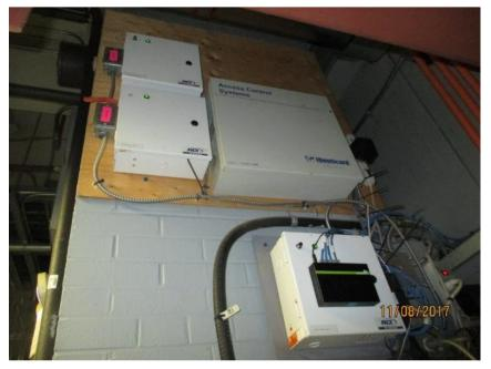
Photo E67 Bridge Access Control System. The bridge is provided with access control system to prevent unauthorized access to the bridge facilities. The access control system was operational at the time of inspection and provides an effective means of ensuring that only authorized personnel can gain access to the facility.
