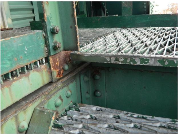
190 Light-Medium Corrosion on Anchor Plate for Catwalk Railing @ South Tower (TYP) Page A2 [95] of A2 [153]
