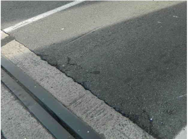
45 Unsealed Cracks & Minor Abrasions on Asphalt near Expansion Joint @ North Approach & North Tower Spans
