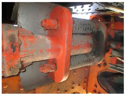
Photo M29 28. The spring and bolts have moderate corrosion.
