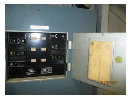
Photo E35 Typical Tower Heater Distribution Panel. This panel is of the existing installation and is in good operating condition.
