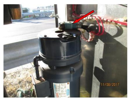
Photo E56 Typical Traffic Gate Motor and Hand Crank Limit Switch. The components are in as-new condition. Note that the gate is provided with a hand crank limit switch (arrow).
