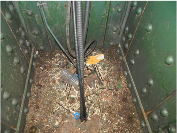
148 Debris on Interior Plate in Northwest Column of North Tower @ Sidewalk Level (TYP) Page A2 [74] of A2 [153]
