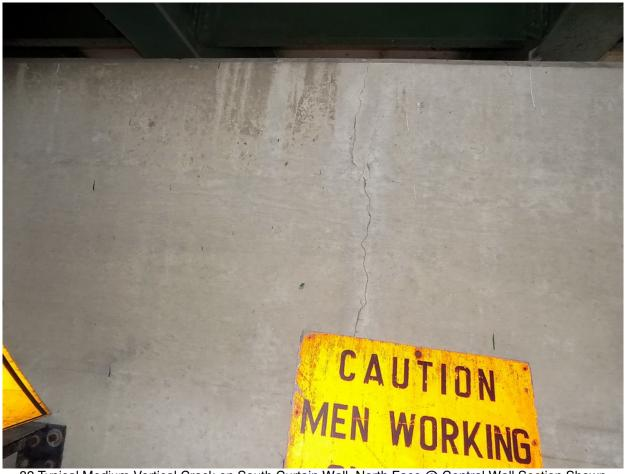
32 Typical Medium Vertical Crack on South Curtain Wall, North Face @ Central Wall Section Shown Page A2 [16] of A2 [153]
