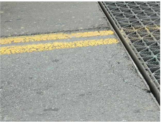
48 Unsealed Crack on Asphalt @ South Tower Span adjacent to Lift Span Grating
