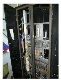
Photo E42 Typical Elevator Control Cabinet. The elevator control is of the original bridge installation. Although still working, it reportedly requires periodic maintenance.
