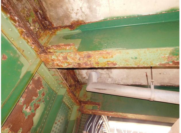
93 Wet Soffit & Heavy Corrosion on Steel below Exp Joint @ North Approach & Tower Spans, looking West
