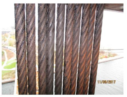
Photo M17 SW-IB Counterweight Ropes. View of the section of the ropes that contact the sheave grooves. Note the corrosion due to inadequate lubricant.
