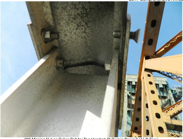
289 Missing Nut on Splice Bolt for Top Handrail @ Post in Panel 7 of Lift Span
