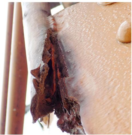
242 Typical Severe Corrosion on Railing Post @ Southeast Lower Guide Bracket
