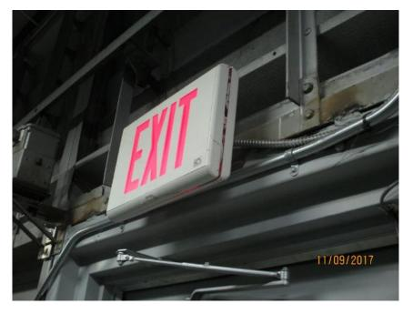
Photo E71 Exit Light. The casing of the Exit light in the generator room was damaged. Otherwise all exit lights are in working order.
