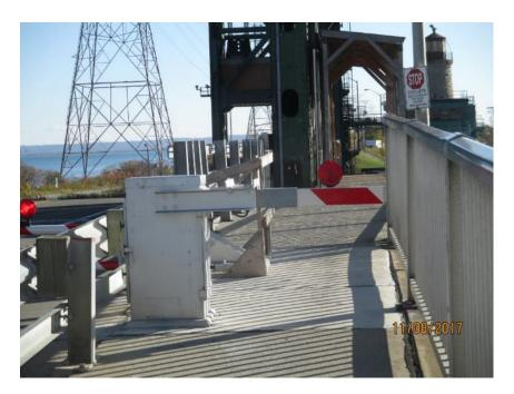
Photo E57 Typical Pedestrian Gate. The pedestrian gate is used to stop pedestrian during the bridge operation. The Pedestrian gates are in as-new condition. Note that the pedestrian gate and signal control are not in the traffic control sequence so that the operator can stop the pedestrian before stopping the traffic.
