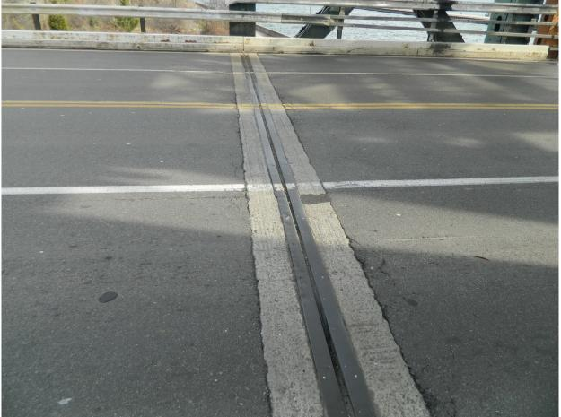
52 Compression Seal Expansion Joint @ North Approach & North Tower Span, looking East Page A2 [26] of A2 [153]
