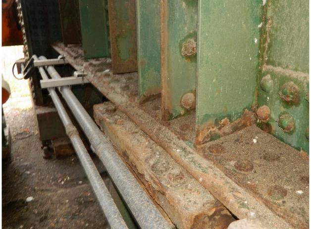
135 Typical Accumulation of Sediment on Front Floor Beam, South Tower Shown
