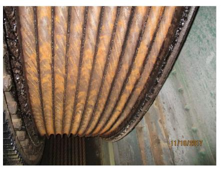
Photo M23 NW-IB Counterweight Sheave. The counterweight grooves are devoid of lubricant and exhibit surface corrosion.
