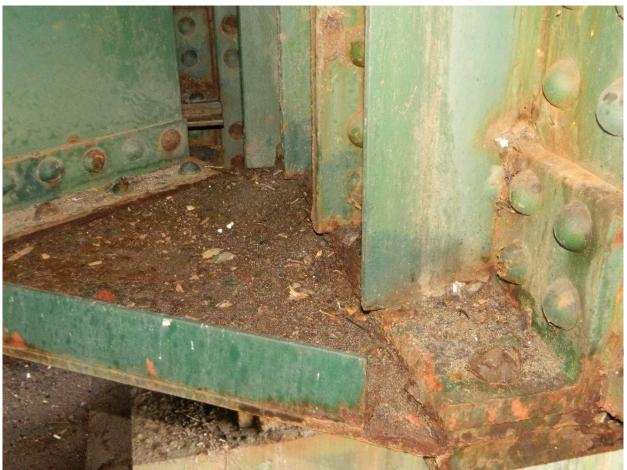
136 Sediment on Gusset Plate behind Front Tower Column, Northeast Column @ South Tower Shown Page A2 [68] of A2 [153]
