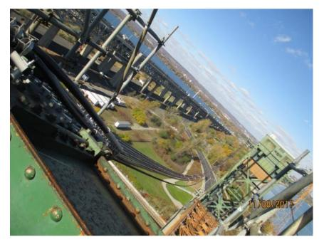
Photo E63 Typical New Aerial Cables Installation (East Shown). The aerial cables were replaced during the recent rehab project. The new aerial cable is the self-supported type and there has been some damage among the cable assemblies due to movement under the wind loads. The aerial cables have been temporary tied together with ropes to mitigate damage. A solution in the form of the installation of aerial cable spacers was underway at the time of the inspection.
