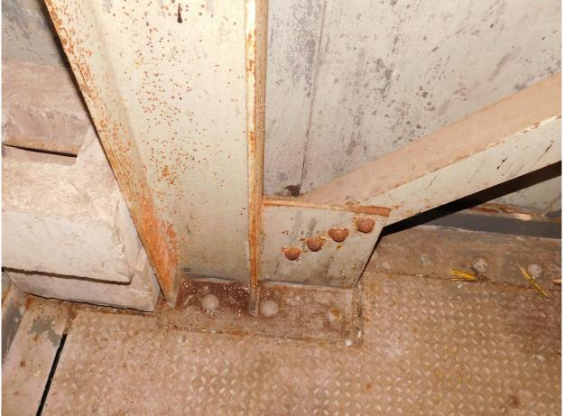
209 Typical Light Corrosion on Steel Frame, Sheave Room in South Tower Shown
