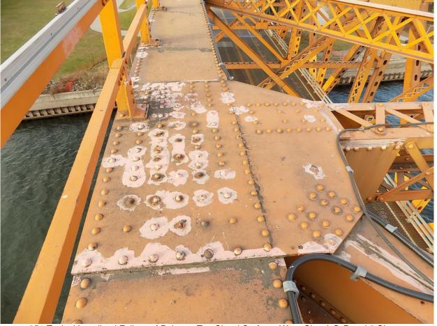
251 Typical Localized Failure of Paint on Top Chord Surface, West Chord @ Panel 3 Shown
