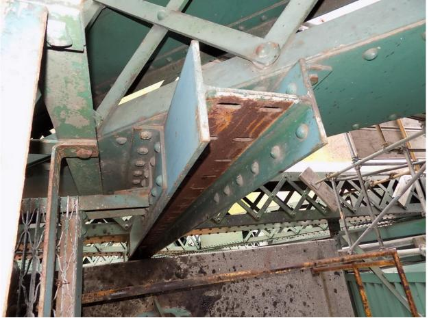
171 Missing Guide-Bar Angles @ top Section of West Guiderail for Counter Weight in North Tower
