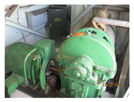
Photo E41 Typical Elevator Motor. The elevator motor is of the original installation.
