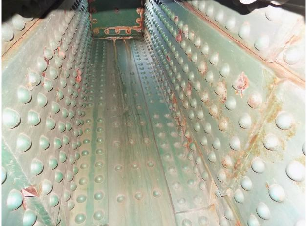
147 Typical Local Peeled Paint & Light Rust on Column Interior, Northeast Column of South Tower Shown
