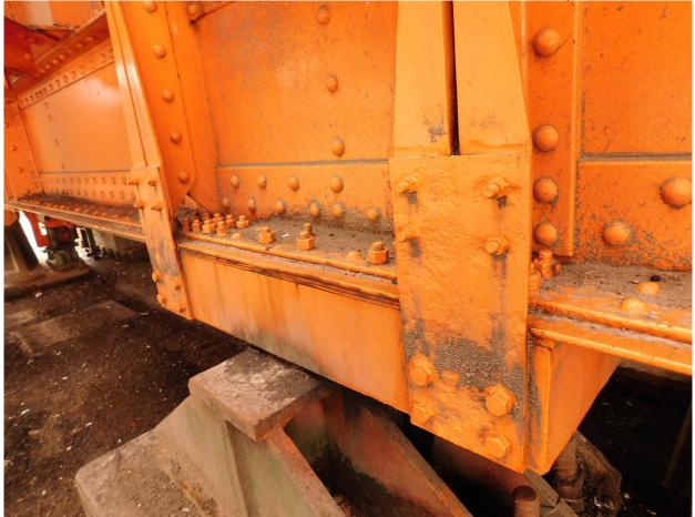
237 Typical Painted-Over Pitted Connecting Plate Surface on End Floor for Centering Shoe, North End Shown
