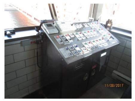
Photo E15 Traffic Control Panel. The new traffic control console top was recently installed. The layout and function of the console top is similar to the old console.
