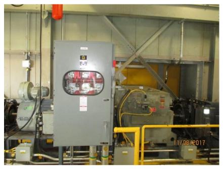
Photo E23 Typical Drive Motor Disconnect Switches. The drive motor disconnect switch is of the original installation and been reused to serve the new motor.
