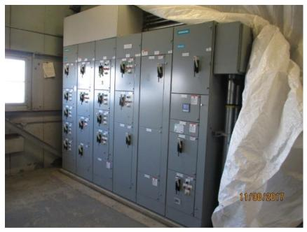
Photo E20 Typical New Motor Control Centre. Note that the white plastic that covers the MCC is the indication of the roof leak.
