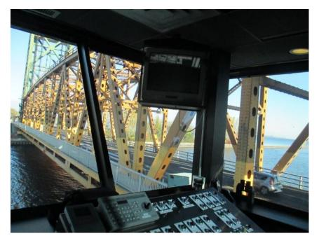
Photo E17 CCTV and Intercom Interface. The CCTV and intercom interface units are mounted on the upright corner of the traffic control console. Note that both CCTV and intercom system are original and are functional. Also note that the CCTV monitor is CRT display and is outdated.
