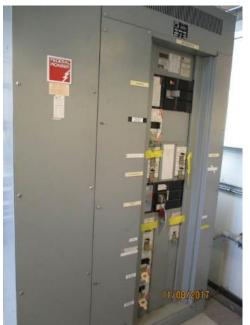
Photo E10 Main Switchboard No.2. This is the main distribution switchboard for the bridge electrical system. Note some change has been made to this switchboard since the 2016 inspection due to the recently completed rehab. project. The changes include new breakers, new labels and disabling of the old drive system feeder breaker with a padlock.
