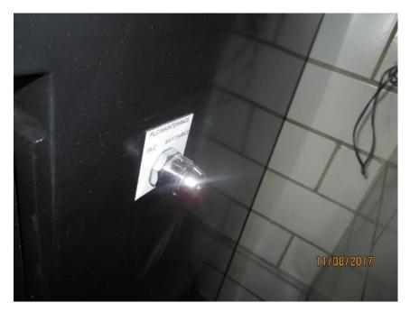
Photo E16 Traffic Control Bypass. A keyed selector switch for PLC and Maintenance select has been installed on the side of the console cabinet as part of the new control system function. Note that the relay mode of the traffic control does not have any interlocks per new logic.
