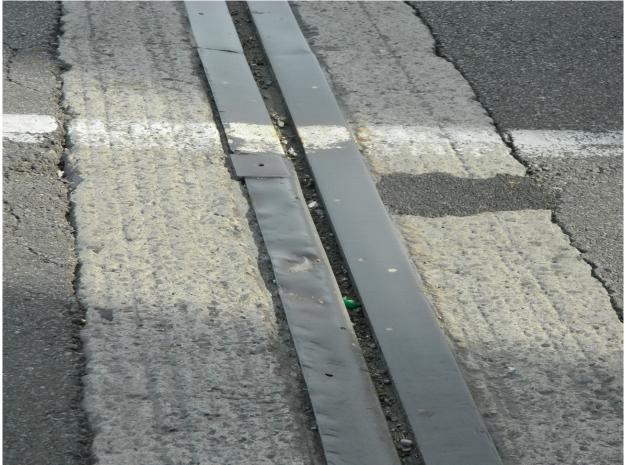
57 Deformed & Abrasion Marks on Joint Steel Angle @ Expansion Joint @ North Approach & North Tower Span
