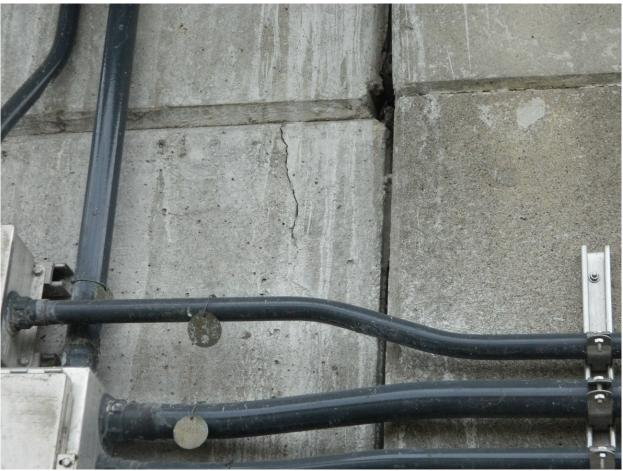
40 Medium Vertical Crack on Upper Mid Section of Northeast Retaining Wall
