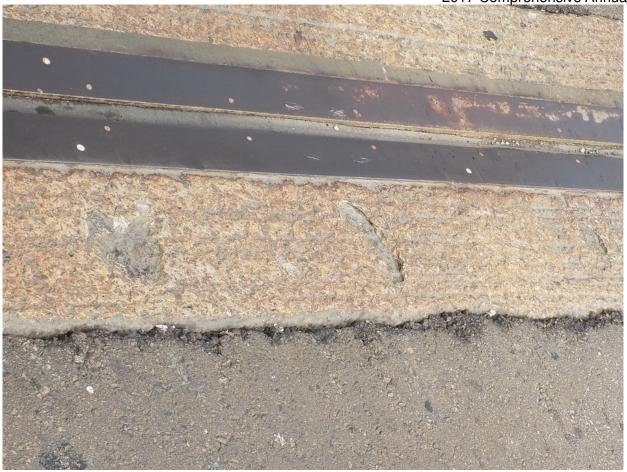
61 Typical Shallow Spalls on End-Dam @ Exp Joint, Joint between South Approach & Tower Spans Shown
