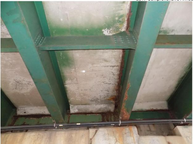
89 North Approach Span, Large Wet Areas on Soffit @ Central Interior Areas of Span
