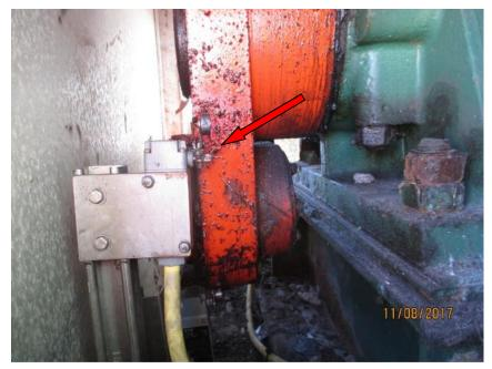
Photo E46 Typical Span Lock Limit Switches at the Center of Lock Machinery. A set of limit switches have been installed at the center of the span lock rotation machinery. These limit switches were installed as part of the recent replacement and upgrade project and are used in place of the original rotary cam limit switch.
