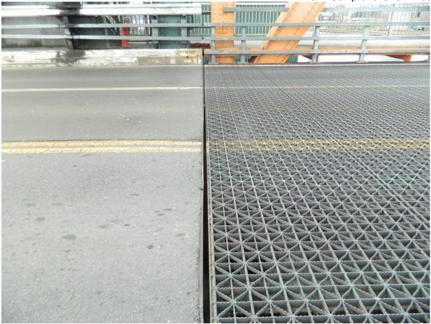
55 Open Gap Expansion Joint @ South Tower & Lift Span Decks, looking West
