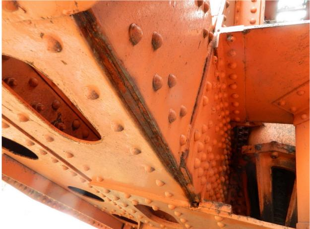
233 Typical Localized Corrosion on Truss Bottom Chord
