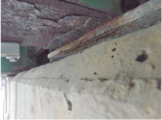
111 North Approach Span, Severe Corrosion on Bottom of Stringer 6 @ North Abutment
