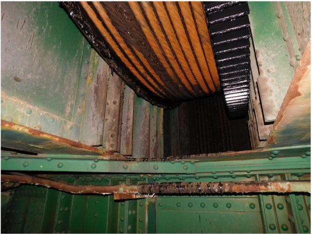
160 Typical Light Corrosion on Bottom of Sheave Girders, South Tower Shown
