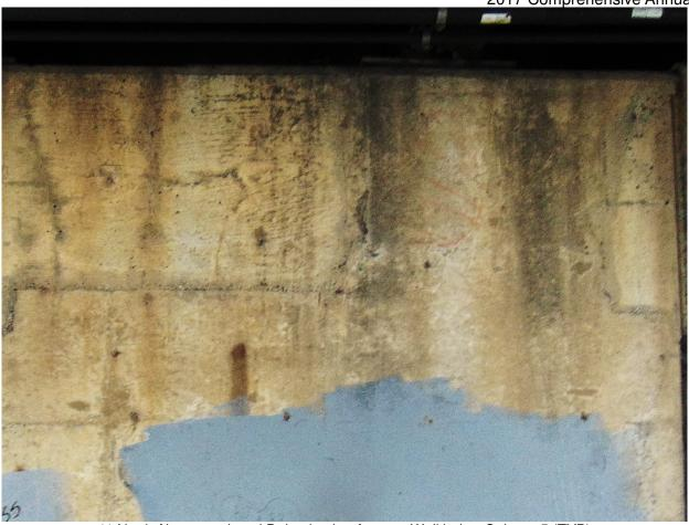
11 North Abutment, Local Delamination Area on Wall below Stringer 5 (TYP)
