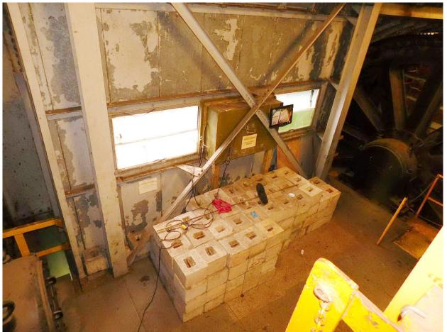
202 Stabilizing Weight Concrete Blocks @ South Central Area of Sheave Room in North Tower (TYP) Page A2 [101] of A2 [153]
