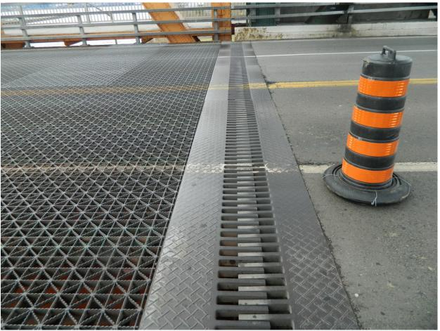
54 Open Gap Finger Plate Expansion Joint @ South Tower & Lift Span Decks, looking West Page A2 [27] of A2 [153]
