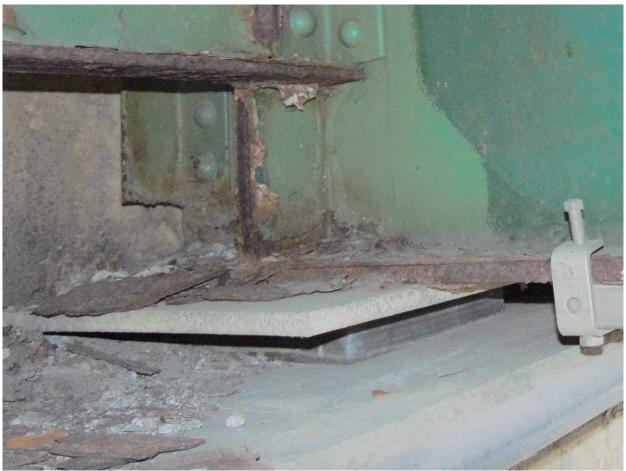
24 Typical Laminated Bearing & Oversized Shoe Plate at North Abutment, Stringer 6 Bearing Shown Page A2 [12] of A2 [153]
