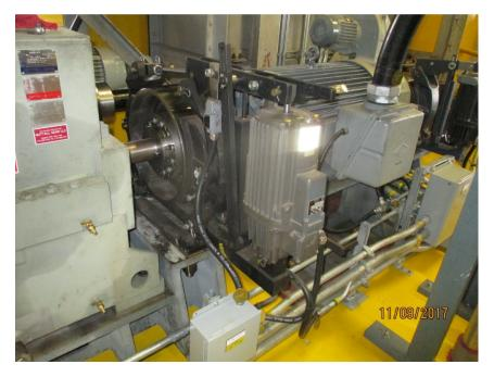
Photo M1 Machinery Brake - SE and Brake Wheel Coupling C3-SE. General view of the machinery brake assembly. Note the unpainted brake wheel coupling bolts.
