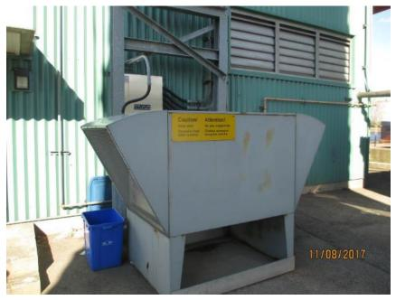
Photo E8 Main Standby Generator Load Bank. This load bank is located outside of the control house and is appropriately sized to exercise the main (600kW) standby generator under load. Note the excellent condition of the load bank enclosure with louver and protective screen.
