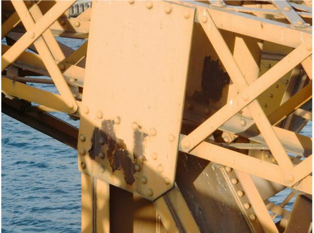
257 Peeled Paint & Light Corrosion on Gusset Plate @ South Portal Bracing
