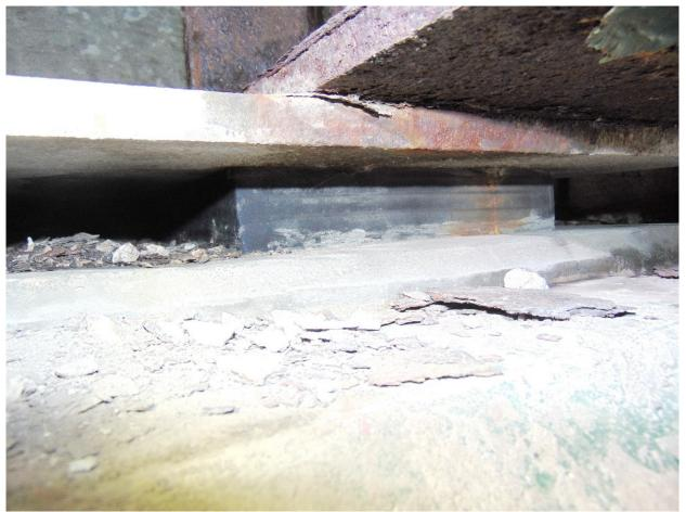
22 Typical Laminated Bearing @ South Abutment, Stringer 2 Bearing Shown
