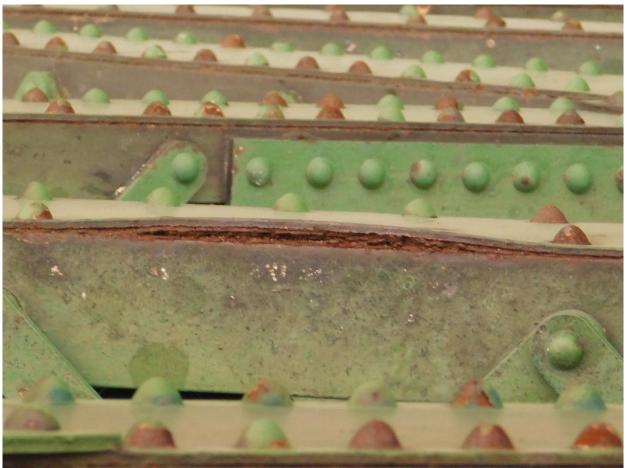
152 Severe Rust Jacking @ Missing Rivets on Horizontal Member 4 of South Tower (TYP) Page A2 [76] of A2 [153]
