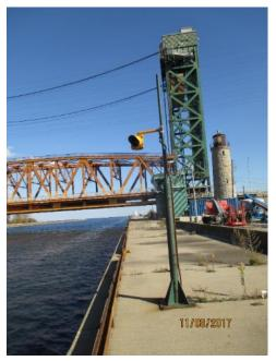
Photo E50 Small Craft Navigation Light. The small craft navigation lights are installed one on each side of the canal. Note the corrosion on its mounting post.
