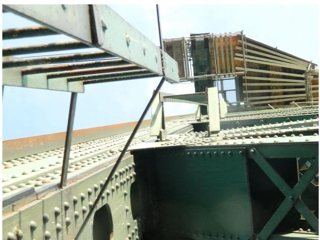
186 Typical Disconnected Lower Section of Disused Exterior Ladder, South Tower near Northwest Column Shown Page A2 [93] of A2 [153]
