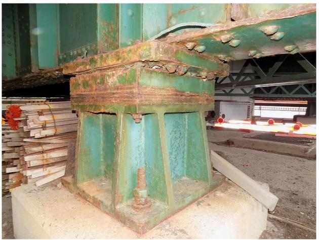
124 South Tower Base, Interior Steel Pedestal Bearing under South Floor Beam
