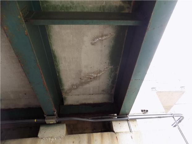
91 North Approach Span, Stained Diagonal Cracks @ Northeast Section
