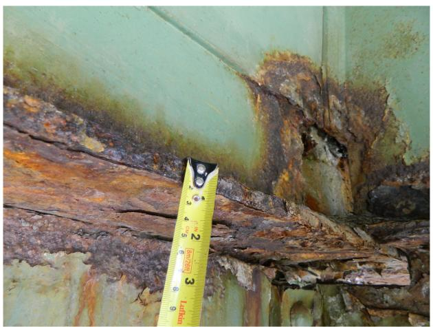
114 Severe Corrosion on Top Flange of Stringer 8 @ North Approach Span
