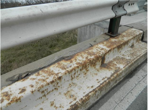
297 Typical Light with Local Medium Corrosion on Steel Curb Plate
