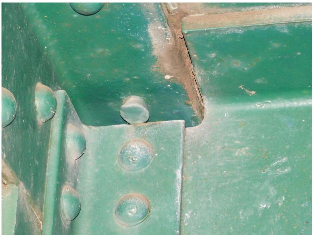
162 Un-Fitted Rivet @Top of 6th Sheave Girder from West above Floor Beam, North Tower Page A2 [81] of A2 [153]
