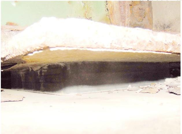
21 Typical Laminated Bearing @ North Abutment, Stringer 5 Bearing Shown
