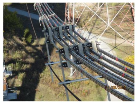
Photo E64 Typical Aerial Cable Spacer Installation (West Shown). The contractor is in the process of installing the aerial cable spacers.
