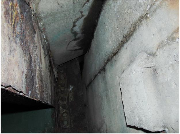
85 Typical Soffit Sloping Towards Structural Steel @ South Abutment, Stringers 3&4 Shown
