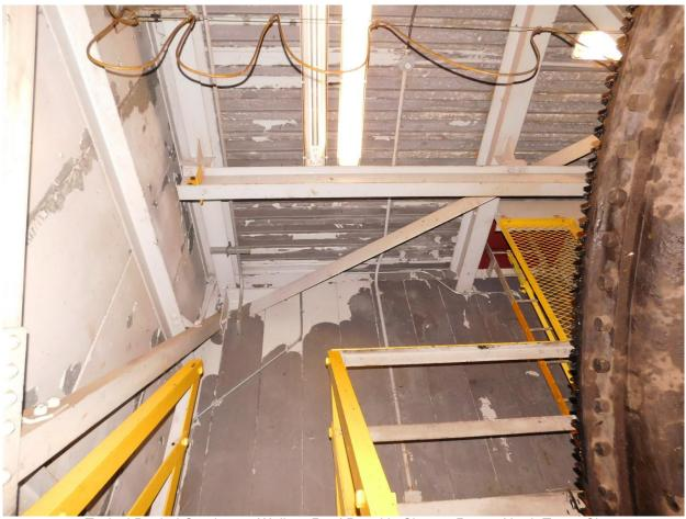
206 Typical Peeled Coating on Walls & Roof Panel in Sheave Room, North Tower Shown Page A2 [103] of A2 [153]
