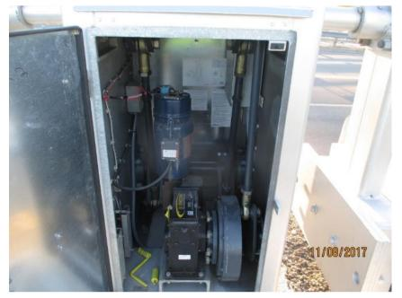
Photo E61 Typical Barrier Gate Enclosure. The barrier gate is in as-new condition. Note that the hand crank handles and drill adapter are laying on the bottom of the enclosure.
