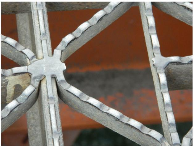
220 Broken Bearing Bar on Grating Panel in Central Section of Northbound Traffic Lane Page A2 [110] of A2 [153]
