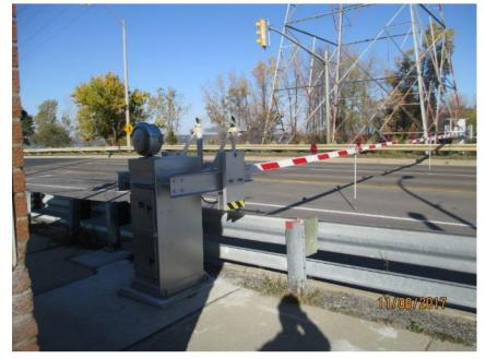
Photo E53 Typical Traffic Gate with Gong. The traffic gates of the new construction and function as expected. Note that the gong on NE traffic gate did not work at time of the inspection.
