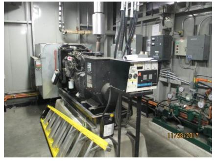
Photo E5 Auxiliary Standby Generator. Note auxiliary standby generator only provide powers the bridge facility and auxiliaries in the event of a utility electric failure but is not used or rated to operate the bridge.
