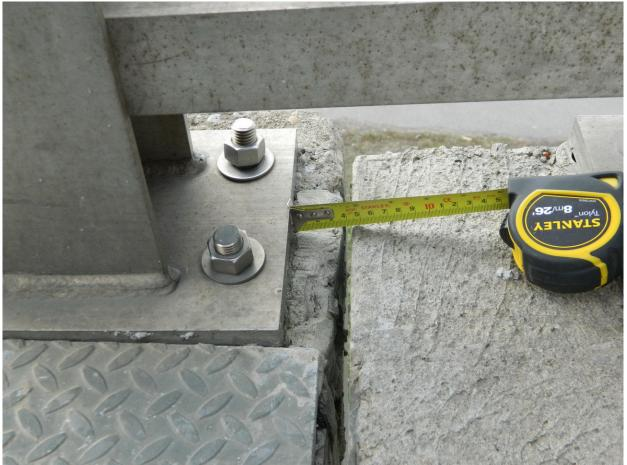
290 Typical Loose Anchor Bolt on West Railing Post adjacent to Abutment Joint, South Abutment Joint Shown Page A2 [145] of A2 [153]
