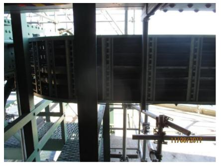
Photo E66 Typical Aerial Suspension Cables on Cable Tray. The aerial cables are well supported and spaced inside the cable tray.
