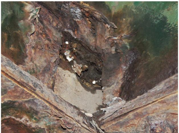
298 Local Severe Corrosion with Perforation Hole on Bent Curb Plate, South Approach Span Shown Page A2 [149] of A2 [153]
