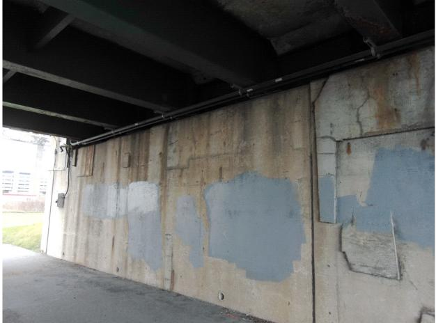
09 North Abutment, Large Patches on Upper West Section of Wall, looking West
