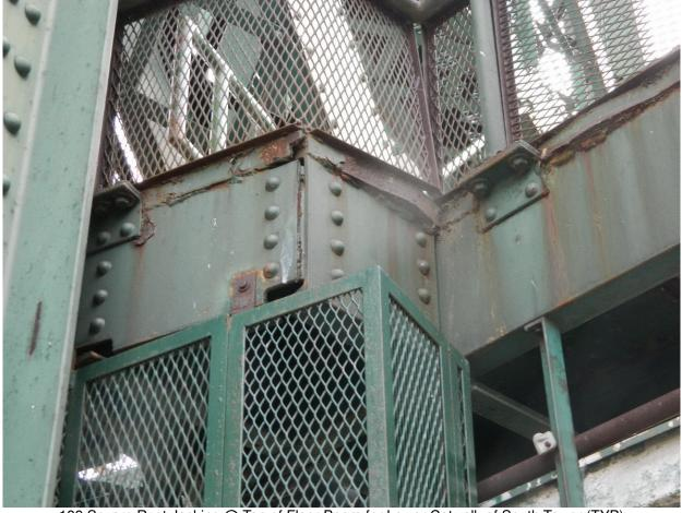
189 Severe Rust Jacking @ Top of Floor Beam for Lower Catwalk of South Tower (TYP)
