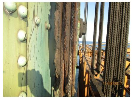
Photo M20 NW Auxiliary Counterweight Ropes. The auxiliary ropes and sheave have built up old lubricant.
