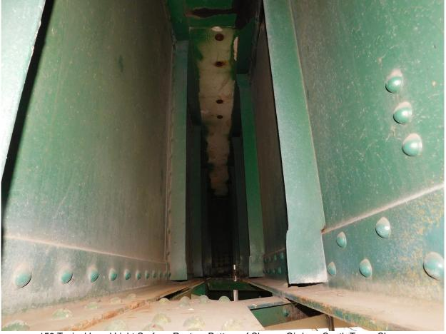
159 Typical Local Light Surface Rust on Bottom of Sheave Girders, South Tower Shown
