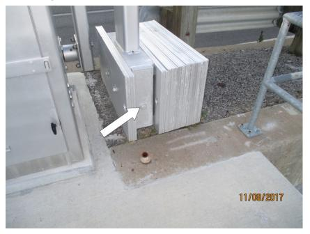
Photo M30 North Barrier Gate. The gate arm counterweight has a bolt that is not fully seated at the east side of the counterweight.
