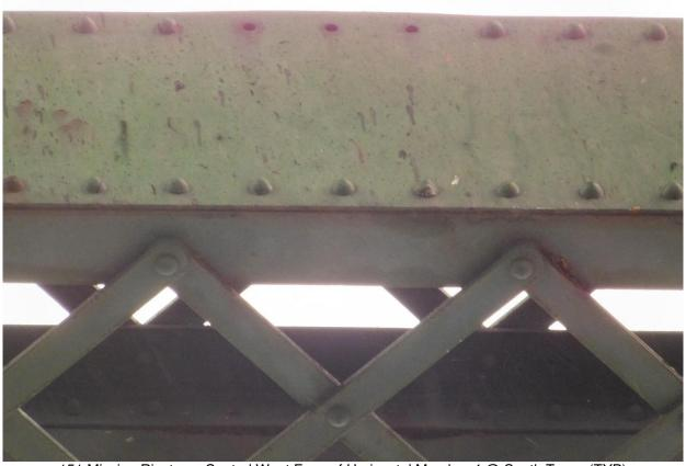
151 Missing Rivets on Central West Face of Horizontal Member 4 @ South Tower (TYP)
