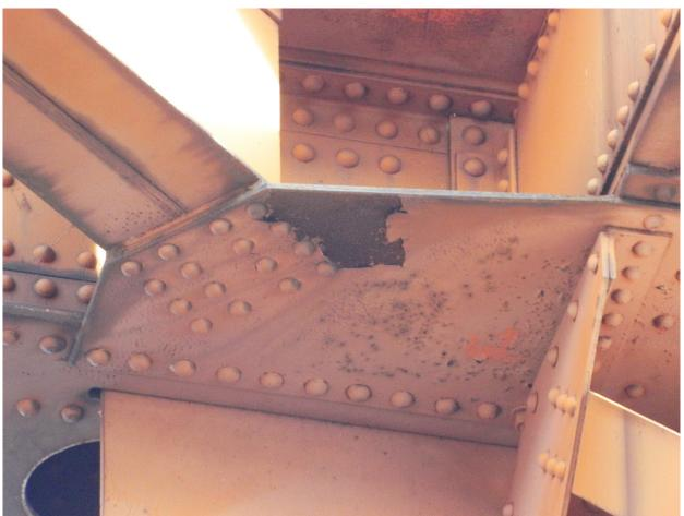
258 Localized Peeled Paint & Light Corrosion on Gusset Plate at Top East Chord near Mid Span Section Page A2 [129] of A2 [153]
