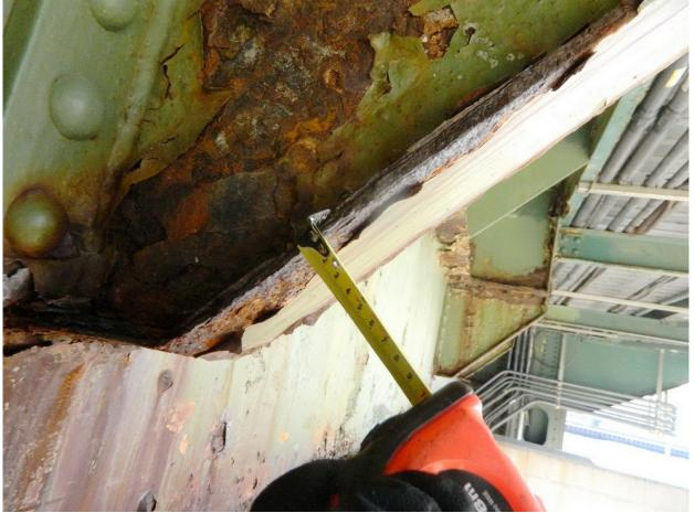
115 Local Severe Corrosion on Bracket for Cantilevered West Sidewalk @ North Approach Span
