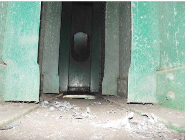
140 Bird Feather & Debris on Bottom interior of East Jacking Girder @ South Tower (TYP) Page A2 [70] of A2 [153]
