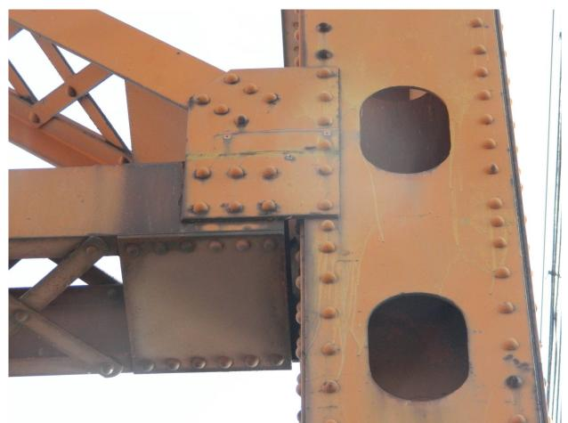
254 Rust Stain & Light Corrosion on Lower Sway Bracing @ Vertical Chord of Truss (TYP) Page A2 [127] of A2 [153]
