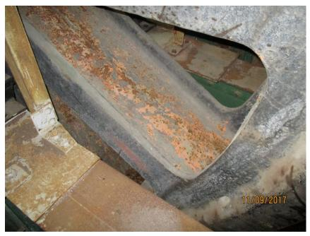
Photo M22 SW-OB Counterweight Sheave. There was paint deterioration and light corrosion on the sheave casting.
