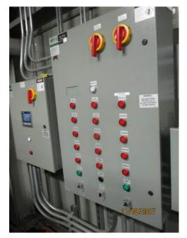
Photo E7 Generator Fuel Pump System. This pump system allows automatic refuelling of the day tank from the main tank located within the control house compounded area. It was previously reported that the main tank status monitoring system has not been properly installed and is currently not operational.
