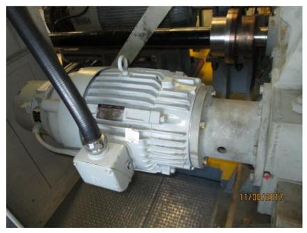
Photo E26 Typical Auxiliary Drive Motor. The new auxiliary motor with integral brake was installed during the recent rehab. Note that the original chain drive aux. has been changed to the direct coupling to the reducer.
