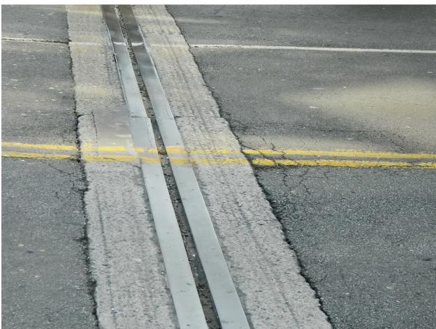
46 Pattern Unsealed Cracks adjacent to Exp Joint End-Dams between North Approach & North Tower Spans Page A2 [23] of A2 [153]
