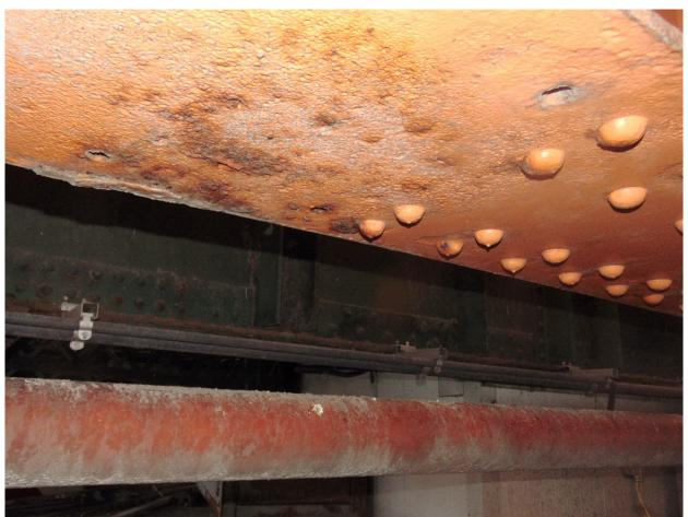
240 Light Rust Stains Bottom Flange & Rivet Holes @ Removed Shoe Plate for Rail Support(TYP) Page A2 [120] of A2 [153]
