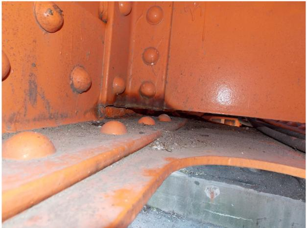
234 Local Light-Medium Corrosion on Internal Stiffener Plate near South End of East Deck Truss Page A2 [117] of A2 [153]
