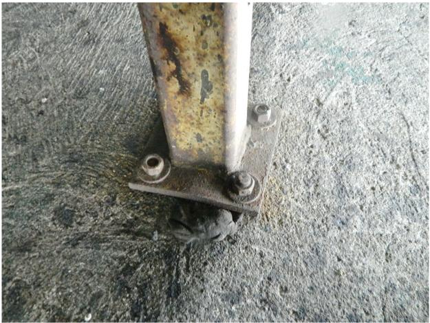
174 Loose Anchor Bolt on Central Post of Safety Rail atop South Counter Weight
