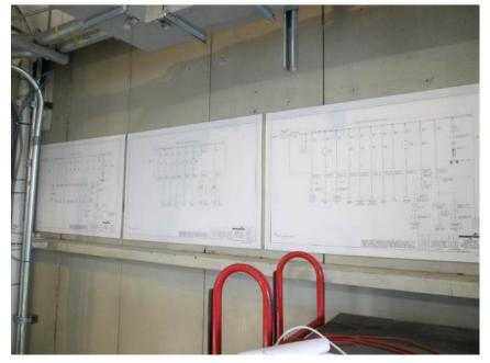
Photo E1 One Line Diagrams in Electrical Room. Note that the "As Built" one-line diagrams of the recently completed rehabilitation project are poster printed.
