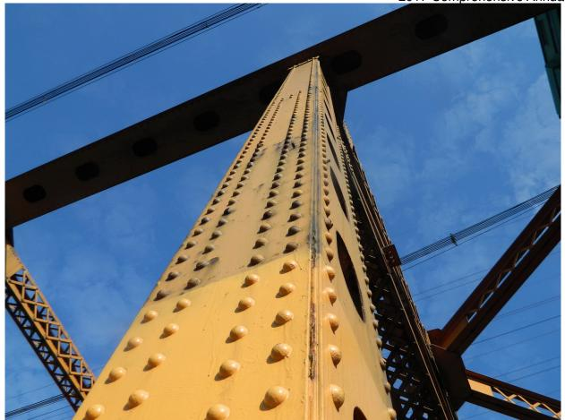
253 Typical Faded Coating & Light Surface Rust on Truss, Vertical Member near SW Corner of Lift Span Shown
