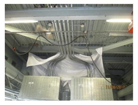
Photo E73 General Lighting and Smoke Detectors (South Tower Shown). The space lighting and fire system equipment is the original installation. They are adequately installed to provide safe work place. Note the cover over the top of the south drive/resistors is the indication of the roof leak. Immediate action should be taken to repair the roof leak in order to keep bridge operating reliably.
