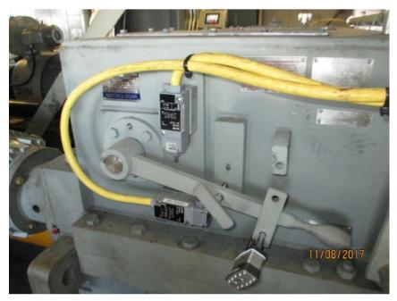
Photo E27 Lever Handle and Limit Switches on the Gear Reducer. Two handles are provided, one on each side the reducer for AUX drive operation and transverse skew adjustment. Many limit switches have been installed on the reducer box for the lever position indication and interlock.
