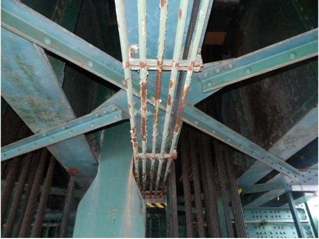
199 Light Surface Rust on Conduits under Sheave Girder in North Tower (TYP)
