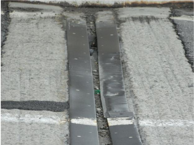
58 Loose Joint Steel Angle @ West Section of Expansion Joint between North Approach & North Tower Span Page A2 [29] of A2 [153]
