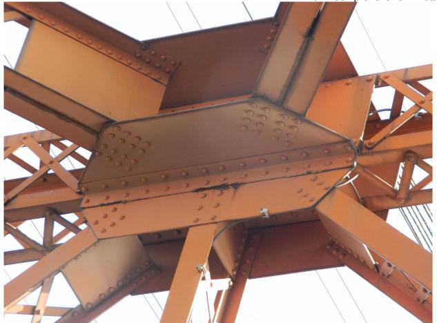
261 Light-Medium Rust Jacking on Gusset Plat @ Mid Section of Upper Horizontal of Sway Bracing @ Panel 5
