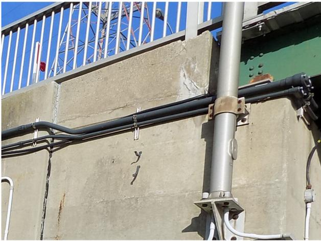
38 Stained Cracks @ top South Corner of Northwest Retaining Wall
