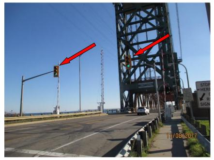
Photo E51 Traffic Signals. Note the good condition of the signals. The light bulbs are LED which extend the life of the bulbs.
