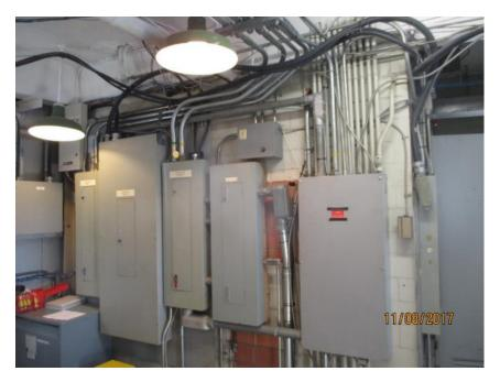
Photo E13 Electrical Room Panelboards. The transformer and the panelboards are of the existing installation. All panels are in good condition with additional circuits been added as part of the recent rehab.
