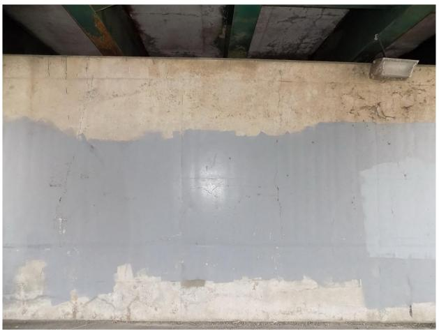
30 North Curtain Wall, Medium Vertical Cracks on East Section of Wall (TYP)
