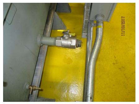
Photo M14 North Span Drive Reducer. There is evidence of a small oil leak at the drain valve.
