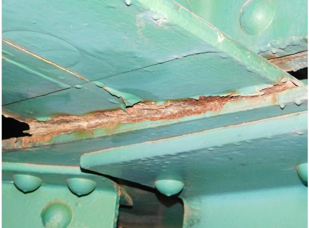
161 Severe Rust Jacking on Bottom North End of 3rd Sheave Girder from West in South Tower
