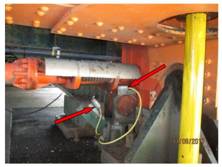
Photo E45 Typical Span Lock Limit Switches at the Lock Bar. These limit switches were installed as part of the recent rehab.
