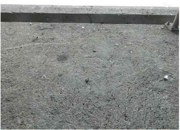
168 Typical Medium Crack on Top Surface of Concrete Counter Weight, North Tower Shown Page A2 [84] of A2 [153]
