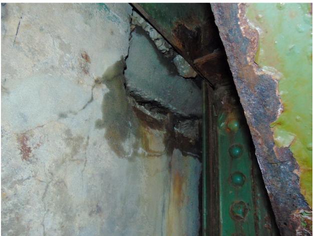
14 Seepage through Spalled at Pathed Area on Upper Section of North Ballast Wall behind Stringer 8 Page A2 [7] of A2 [153]
