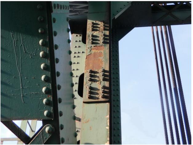
172 Blistered & Peeled Paint on Guiderail for Counter Weight on West Side of South Tower @ Panel 2 Page A2 [86] of A2 [153]
