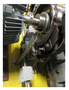
Photo E34 Typical Speed Switch Sensor. The speed switch sensor and pulse wrap are installed between the motor and machinery brake for overspeed protection. The units are well installed.
