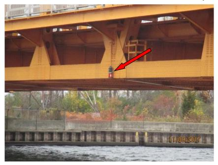
Photo E48 Typical Span Navigation Light. The bridge is provided with two span navigation lights, one facing each approaching navigable channel. These lights were found to be operational at the time of inspection and in good serviceable condition.
