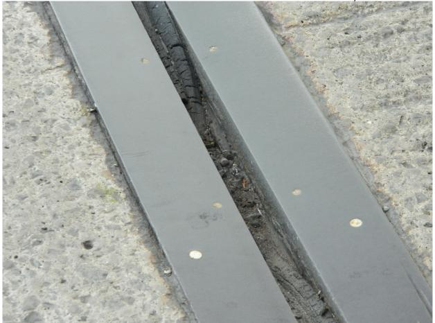
59 Loose Compression Seal in West Section of Expansion Joint between North Approach & North Tower Span
