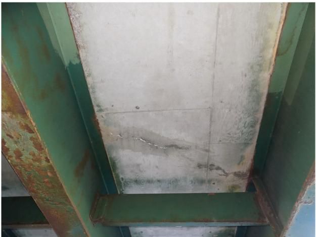
92 North Approach Span, Diagonal Stained Crack with Wet Area on East Soffit near Mid Section of Span Page A2 [46] of A2 [153]
