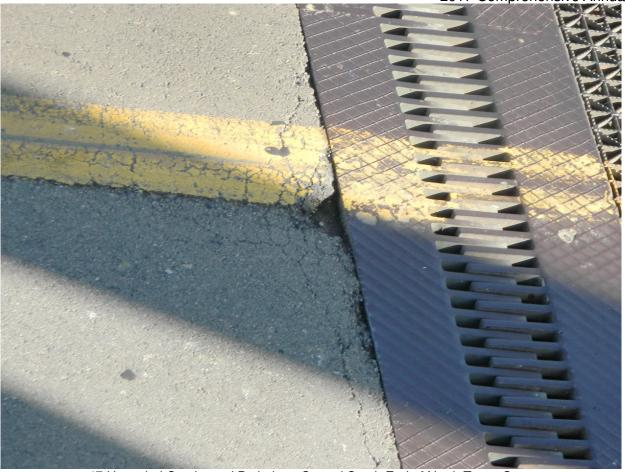
47 Unsealed Cracks and Pothole at Central South End of North Tower Span
