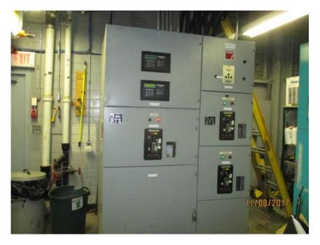
Photo E3 Switchboard #1. The switchboard is the original installation and is in good condition. Note that the utility and generator power main breakers are electrically operated and interlocked. There is no mechanical interlock for this manual transfer means.
