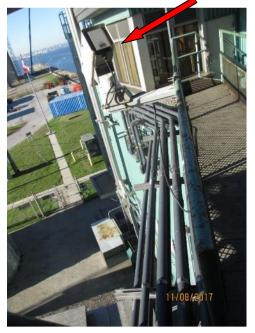
Photo E68 CCTV System. The CCTV cameras are strategically located throughout the bridge to monitor the roadway approaches, waterway approaches and main access areas to the bridge. The operation can monitor all these location from the operator's room via a CCTV monitor. The camera installation was found to provide good visual information and had been well installed.
