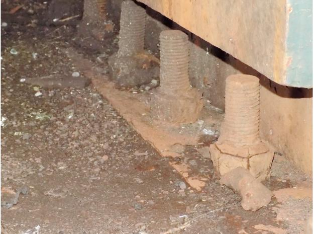
127 Severe Corrosion on Anchor Bolts for Anchorage Assembly for Front Tower Column, NW Column @ South Tower
