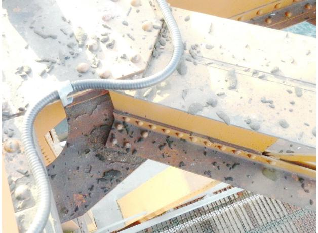
259 Light-Medium Corrosion on top of Portal Bracing Gusset Plate @ West Corner of South Lifting Girder
