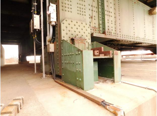
123 Typical Anchorage Assembly on Rear Tower Column, Northwest Column @ North Tower Shown
