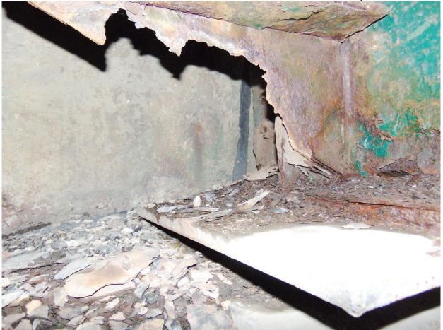
113 Severe Corrosion on Stringer 8 & Perforated Stiffener for Diaphragm @ South Abutment
