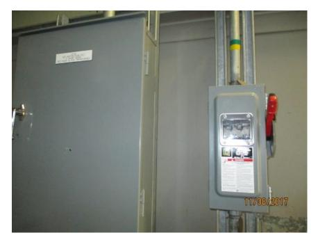
Photo E36 Typical New Lighting and Disconnect. A transformer, a disconnect switch and a lighting panel are of part of the new installation during the recent bridge rehabilitation. These components are in an as-new condition.
