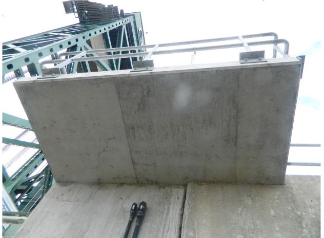
37 New Cantilever Slab for Swing Gate Support on Northeast & Southeast Retaining Walls, Northeast Wall Shown
