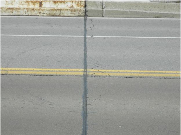
56 South Expansion Joint, Pattern Unsealed Cracks @ East Section of Paved-over South Exp Joint Page A2 [28] of A2 [153]
