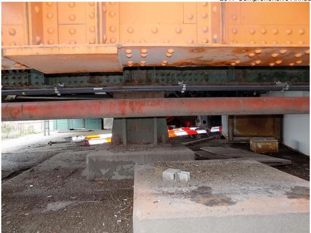
239 Removed Shoe Plate from Bottom Flange Railway Live Load Support @ South Pier (TYP)
