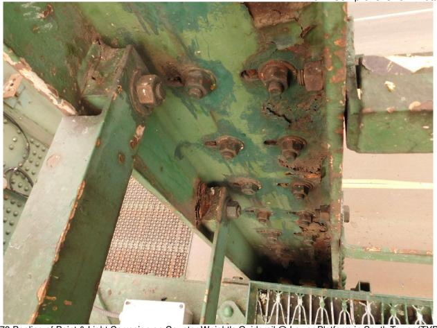
173 Peeling of Paint & Light Corrosion on Counter Weight's Guiderail @ Lower Platform in South Tower (TYP)
