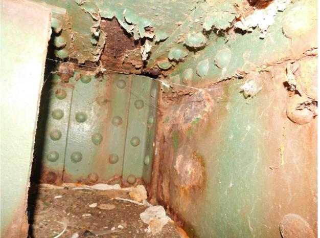
125 Local Severe Corrosion on Anchor Assembly for NW Rear Column @ North Tower
