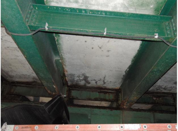
95 North Tower Span, Wet Areas on Soffit @ Northwest Section of Span
