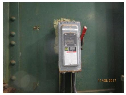
Photo E44 Typical Span Lock Motor Disconnect Switch (North Disconnect Switch Shown). The disconnect switch is rated NEMA 3R and exhibits excessive corrosion.
