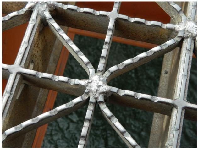
218 Typical Weld Repaired on Original Deck Grating
