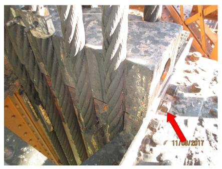
Photo M19 NW-OB Main Lift Girder Splay Casting. The middle nut is not fully seated at this location (arrow). Also note the light fretting at the rope/splay interface.
