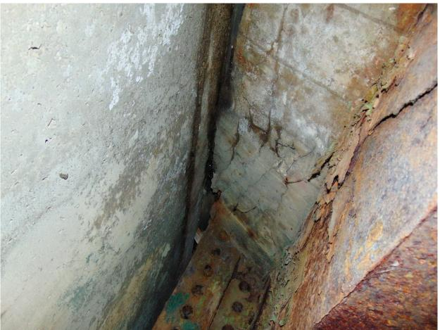
86 Typical Wet Soffit & Severe Corrosion on Steel below Abutment Joints, South End @ Stringers 5&6 Shown Page A2 [43] of A2 [153]
