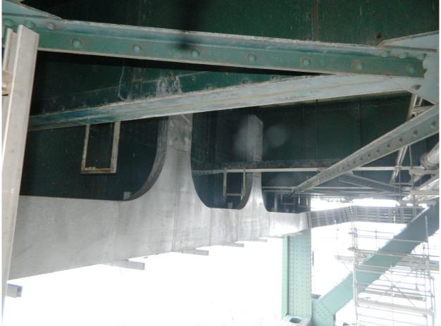
197 New Cable Tray behind Rear Transverse Sheave Girder @ North Tower (TYP)
