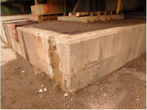
121 Cracks & Local Severe Scaling on Concrete Base @ North Tower's Southwest Leg
