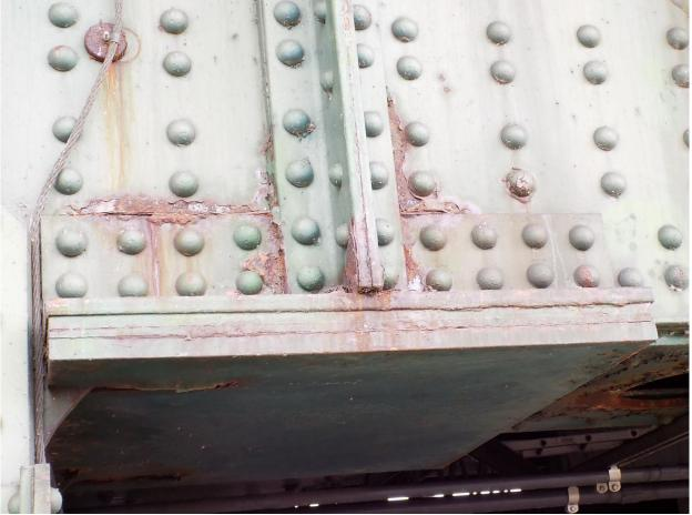
139 Local Medium Rust Jacking on Bottom North Section of West Jacking Girder @ North Tower (TYP)
