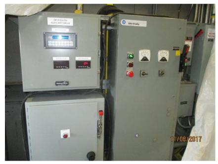
Photo E28 South Auxiliary Drive Controller and Span Height Indication Panel. The auxiliary drive was relocated along with the MTS and emergency power panelboard. They are all in good serviceable condition. Note the white plastic sheet cover over the units is the indication of the roof leak in the area. The span height indication is recently installed.
