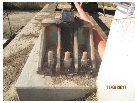
Photo M26 North Centering Device. There is minor debris accumulation on the support. The anchor bolts have paint deterioration and section loss.
