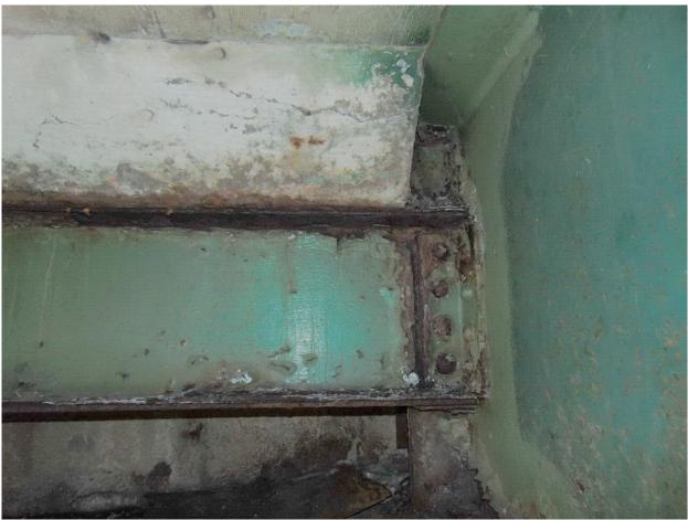
90 North Approach Span, Local Delam on Soffit atop North End Diaphragm @ Stringer 6 Page A2 [45] of A2 [153]
