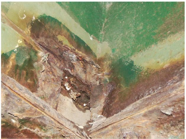
116 South Approach Span, Perforated Curb Plate @ South Expansion Joint End
