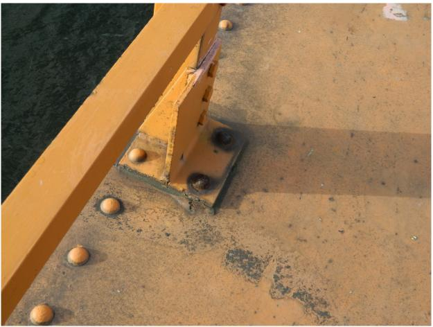
252 Typical Light Corrosion Spots on Post Base atop of Truss's Top Chord
