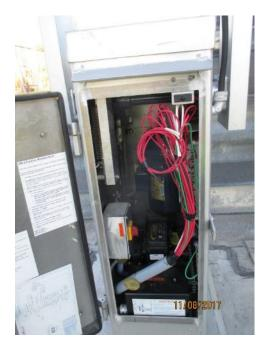
Photo E58 Typical Pedestrian Gate Enclosure. Note that the length of wires inside the gate is excessive in such a small enclosure. Otherwise the gate is in as-new condition.
