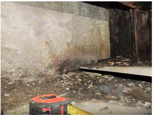
20 South Abutment, Large Delamination on South Ballast Wall near Stringer 7
