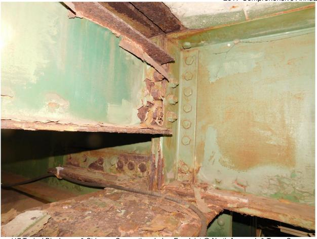
117 Typical Diaphragm & Stringers Connections below Exp Joint @ North Approach & Tower Spans
