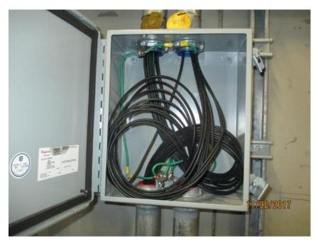
Photo E70 Typical Bonding. The raceway system bonding is well installed and conform to the CSA standard.
