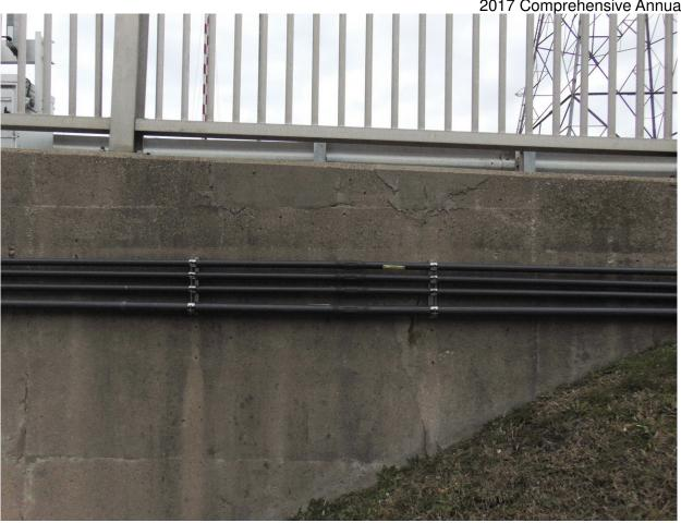
39 Isolated Vertical Crack & Local Patched Areas on Southwest Retaining Wall (TYP)
