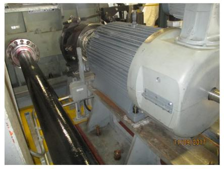
Photo M5 Motor-SW. The motor mounting bolts and support anchor bolts are unpainted with light corrosion forming. The shims and the top of the support are also unpainted.
