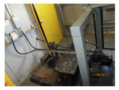
Photo E31 Span Resolvers. One single turn resolver and one multi-turn resolver have been attached to the existing gearbox after removing the old control devices.
