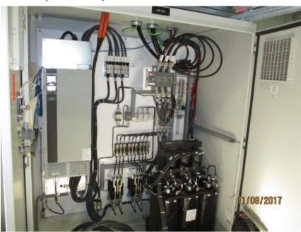
Photo E22 Typical VFD Drive System. The 200HP Danfoss VFD drive, 18 poles transformer and rectifier are well installed inside the drive enclosure.
