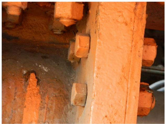
276 Loose Bolts on front West Side of Southeast Saddle Shoe of Lift Span
