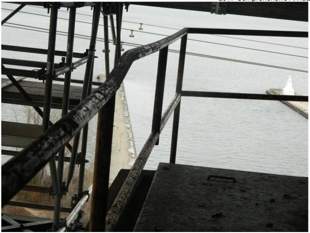
175 Bent Pipe Rail near Northeast Corner of North Counter Weight, looking East
