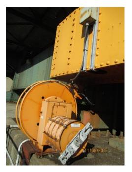
Photo E62 Typical Cable Reel (North Shown). Provides power and control for electrical equipment on the movable span. Note the corrosion throughout the cable reel body.
