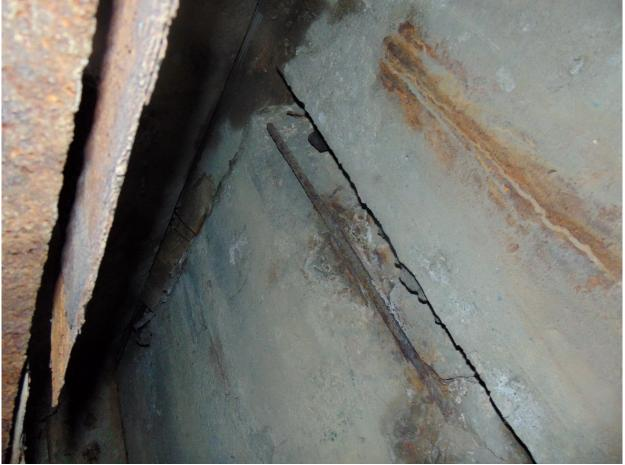
13 North Abutment, Exposed Bar in Spalls @ Central Construction Joint in North Ballast Wall
