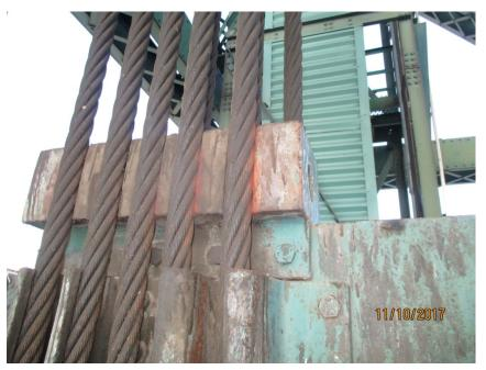
Photo M16 NW-OB Counterweight Rope Connections. There was fretting where the counterweight ropes rub against the counterweight splay casting. There was also light corrosion in spots due to inadequate lubricant.
