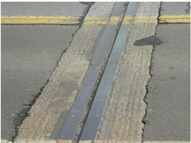
60 Concrete & Asphalt Patches and Minor Spalls on End-Dams between South Approach & Tower Spans Page A2 [30] of A2 [153]
