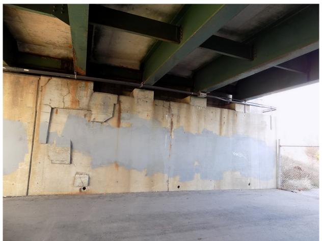
08 North Abutment, Large Patches & Isolated Medium-Wide Vertical Cracks on Central & East Section of Wall Page A2 [4] of A2 [153]
