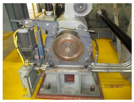
Photo M2 Motor Brake-SE. General view of a typical motor brake assembly. The brake assembly, including the brake wheel hubs and fasteners are unpainted.
