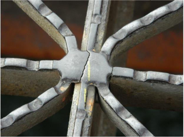
219 Typical Cracked Grating Panel, Central Section of Northbound Lane Shown
