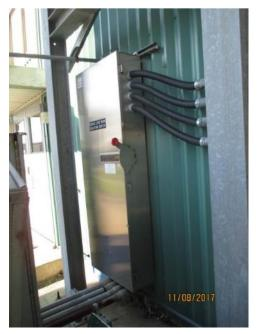
Photo E9 Load Bank Disconnect Switch. The disconnect switch is wall mounted outside the generator room facing the load bank. Note the as-new condition of the disconnect switch.
