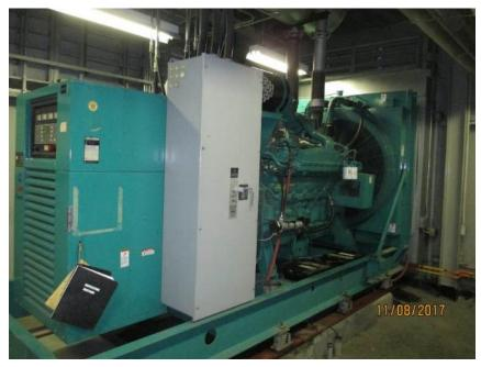
Photo E4 Main 600kW Standby Generator. Generator is used as an alternative source of power to operate the bridge. The standby generator is well maintained and been tested monthly.
