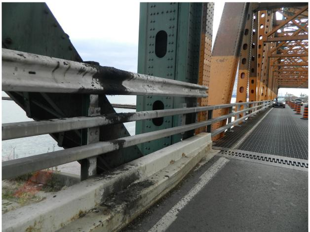
282 Typical Grease on Railings below Counterweight Guiderail @ Tower Span, East Railing @ North Tower Shown Page A2 [141] of A2 [153]
