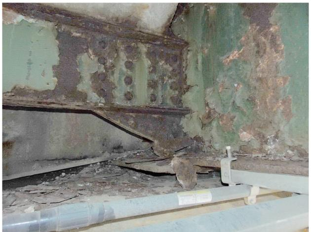
112 Typical Heavy Corrosion on Steel Diaphragm-Gusset Plate & Stringer at North Abutment, Stringer 3 Shown Page A2 [56] of A2 [153]
