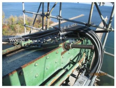
Photo E65 Typical Aerial Suspension Cables Routing. Sufficient bending radius has been created for the aerial cable before routing into the cable tray.
