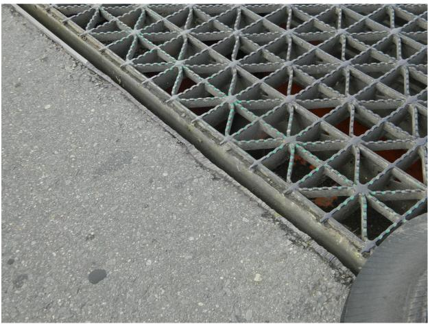
62 Severe Abrasions on Top East Section of End Plate for Open Gap Expansion Joint @ South Tower & Lift Span Page A2 [31] of A2 [153]
