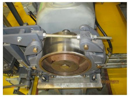
Photo M3 Motor Brake-SE. Areas of paint were found on the friction surface of the brake wheel.
