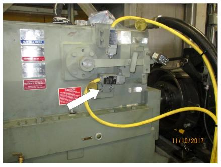
Photo M15 North Span Drive Reducer. There is evidence of a small oil leak at the north index spline lower limit switch plate bolts (arrow).
