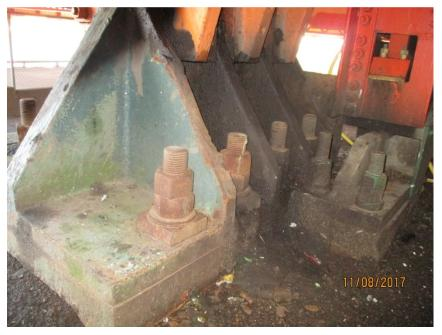
Photo M25 SW Live Load Support. The anchor bolts were corroded.
