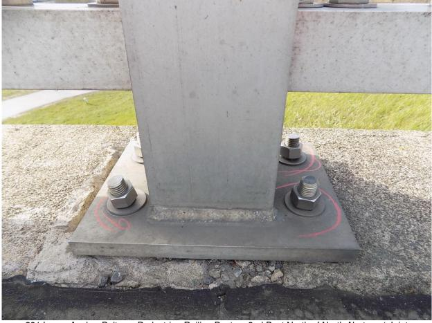
291 Loose Anchor Bolts on Pedestrian Railing Post on 2nd Post North of North Abutment Joint
