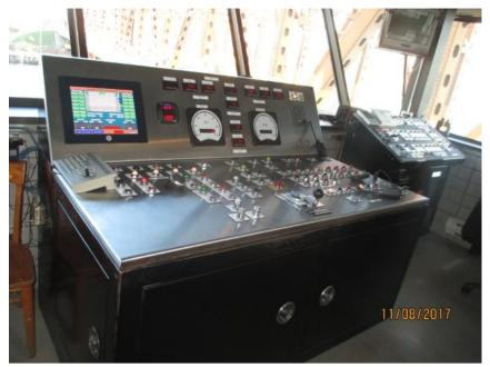
Photo E14 Main Control Desk. New upgraded console top is provided during the recent rehabilitation project. The console is in excellent condition.
