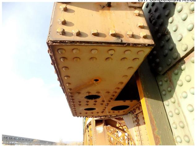
263 Light-Medium Rust Jacking on Bottom Corners of Southwest Guide Roller Assembly
