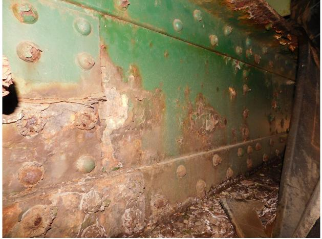
133 North Tower, Severe Corrosion on Lower South Face Section of Rear Floor Beam near NW Column
