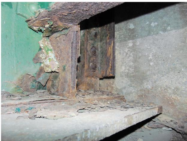
110 Typical Severe Corrosion on Stringers & Diaphragms at Abutment End, Stringer 6 @ South Abutment Shown Page A2 [55] of A2 [153]
