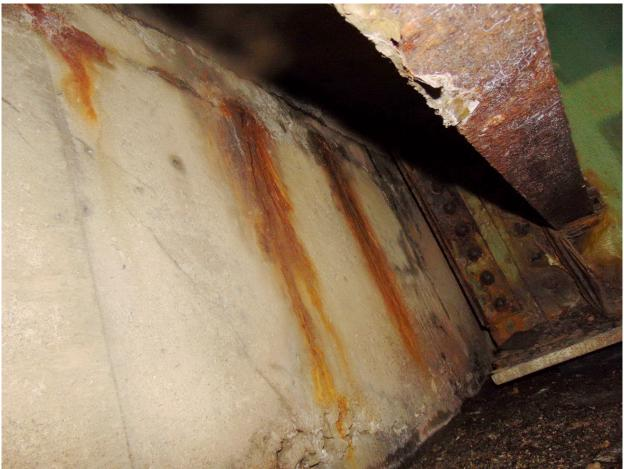
12 North Abutment, Cracks-Rust Stains-local Spalls on West Section of North Ballast Wall (YP) Page A2 [6] of A2 [153]
