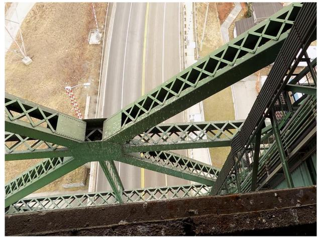
146 Typical Bird Dropping on Tower Steel, South Tower Shown
