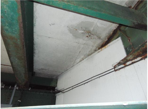
97 North Tower Span, Stained Crack with Wet Area on Interior Soffit near Mid-Span @ Stringer 4
