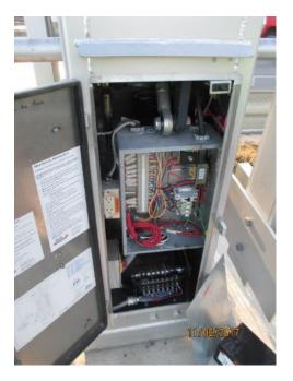
Photo E55 Typical Traffic Gate Enclosure. The equipment inside the gate enclosure is in asnew condition.
