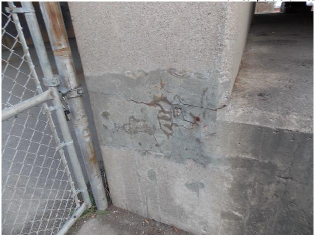
31 North Curtain Wall, Crack @ Horizontal Construction Joint on Bottom West Face of Wall
