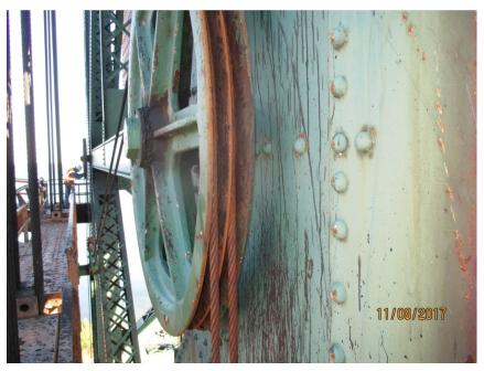
Photo M21 SW Auxiliary Counterweight Ropes. The counterweight ropes and sheave are devoid of lubricant.
