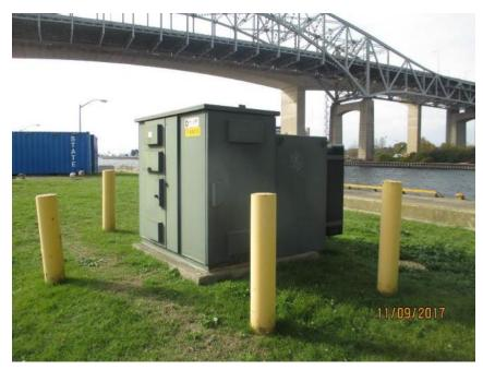
Photo E2 1,000KVA Outdoor Pad Mounted Incoming Service Transformer/Unit Substation. Note the primary service to the transformer is 13.8kV from the local utility overhead supply and secondary of the transformer serves the bridge at 575volt, 3-phase, 60 Hz.
