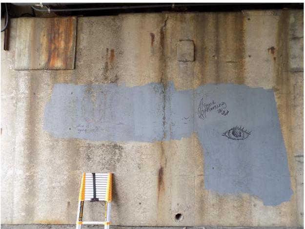
10 North Abutment, Typical Stained Vertical Crack on North Abutment Wall, West Section of Wall Shown Page A2 [5] of A2 [153]
