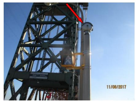
Photo E52 Typical Pedestrian Light and Pedestrian Bell. The pedestrian light is LED type Walk and Halt light. All pedestrian lights functioned properly. The North pedestrian bell (arrow) was out of service and should be fixed.
