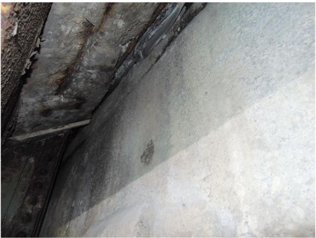
88 Wet Area & Spalls on South End Soffit between Stringers 6&7
