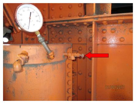
Photo M27 NW Span Air Buffer. The exhaust valve handle (arrow) is broken.
