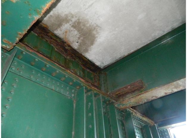
105 Wet Soffit @ Stringers 2&3 adjacent to Exp Joint @ North End of South Approach Span
