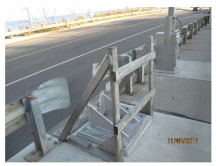
Photo E60 Barrier Gate Receiver. Note the wooden fencing around the receivers for temporary protection. Note that due to the independent of the pedestrian gate operation, the pedestrian can possibly come close to this receiver while the barrier gate is lowering. The wooden fencing was created after the barrier gate installation during the rehab but permanent railing should be provided to keep the pedestrian away from the receiver pocket.
