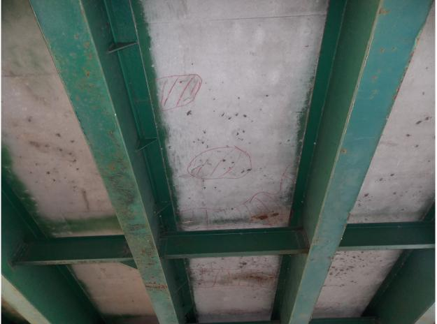
103 South Approach Span, Delam on Central Interior Soffit
