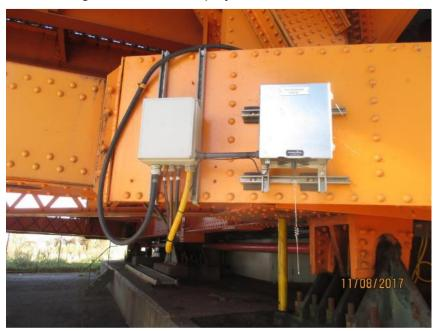
Photo E39 Span Inclinometer Enclosure. Per the rehab design, the span inclinometer was originally installed in the enclosure and communicated wirelessly with the transmitter located inside the CP-2 enclosure. The inclinometer was to be used for the span skew control but does not function.
