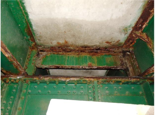
107 Wet Soffit @ Stringers 3&4 below Expansion Joint between South Approach & Tower Spans
