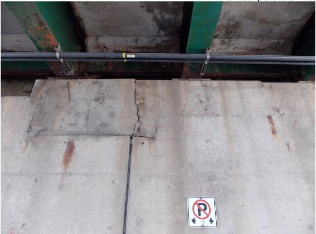
15 South Abutment, Large Concrete Patch with Wide Vertical Crack & Delamination below Stringers 4&5
