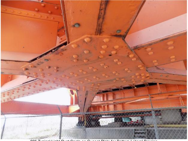
235 Typical Light Rust Spots on Gusset Plate for Bottom Lateral Bracing
