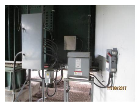
Photo E47 Lighting Panel on North Pier (LP-4). The disconnect switch, transformer, lighting panel and the lighting contactor are of the original installation. The lighting contactor has been modified to work with the current control system.
