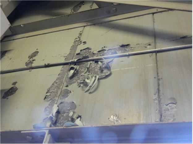
207 Severe Peeling of Paint Coating on East Wall of North Equipment Room
