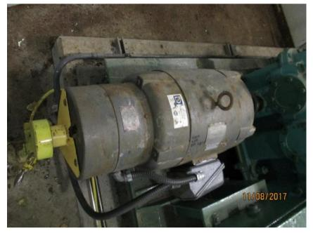
Photo E43 Typical Span Lock Motor. Note the lock motor is of original installation. A limit switch has been installed as part of the hand crank installation and used to prevent electrical operation of the lock motor when the hand crank cover is removed. The hand crank limit switch has been replaced during the recent rehab.
