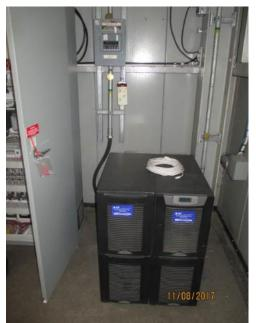
Photo E12 New UPS and UPS Distribution Panel. The UPS and its distribution panel is located next to the CP-2 and is in as new condition. Note the different type of laminated
