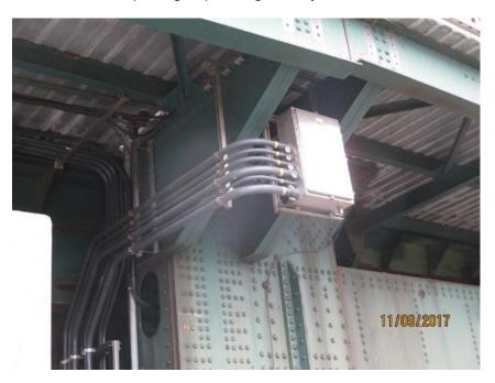
Photo E74 Typical Outdoor Raceway Installation. The newly installed conduit and stainless steel pull boxes are in as-new condition.
