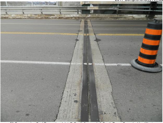
53 Compression Seal Expansion Joint @ South Approach & South Tower Span, looking West
