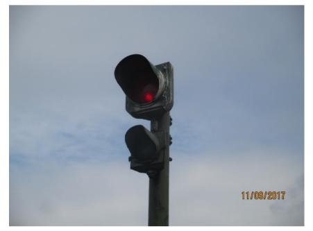
Photo E49 Typical Marine Traffic Navigation Light. The marine traffic lights are located at the tip end of the pier for signaling approaching vessels. The lights are operational but lights and poles exhibit minor signs of corrosion.
