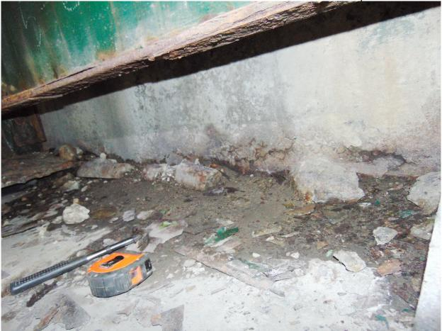
19 South Abutment, Typical Concrete Debris on Bearing Seat
