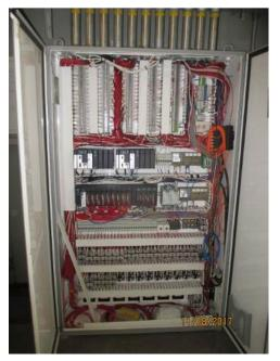
Photo E11 New CP-2 Control Panel. New free standing control panel was installed as part of the recent bridge rehabilitation work. The redundant PLC system and control devices are properly installed inside the panel. Note that the wireway cover cannot be mounted due to over saturated wires in the wireway in some area. The new control system has been updated to the newest GE PLC with improved functions and performance.
