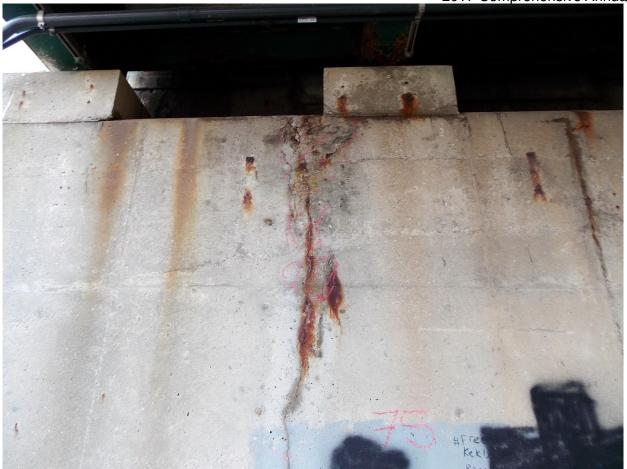
17 South Abutment, Wide Vertical Crack with Rust & Delamination on Wall between Stringers 1 &2
