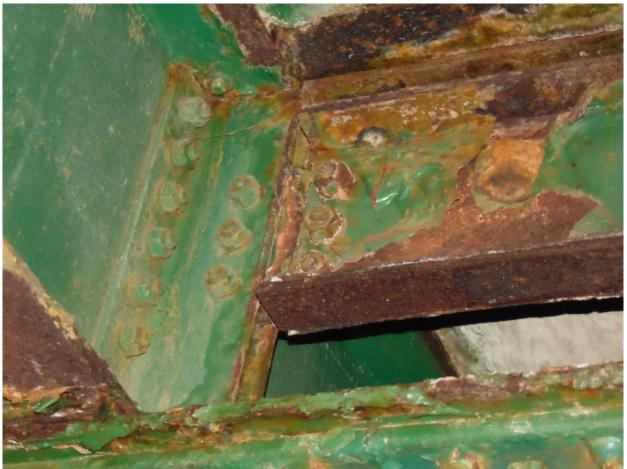
118 Typical Stringers & Diaphragm Connections below Exp Joint between South Approach & Tower Spans Page A2 [59] of A2 [153]
