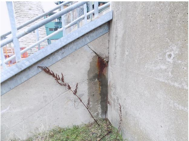
306 Wide Crack with Leakage on Lower Southwest Staircase Section near Retaining Wall Page A2 [153] of A2 [153]
