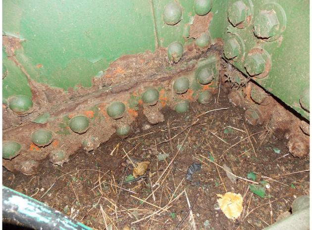
129 Sediment Accumulation @ Interior Bottom Plate of Tower Column, Northeast Column @ North Tower Shown
