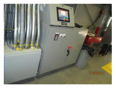
Photo E29 Typical Pull Box and Control Cabinet (CP-3) in South Tower. The control cabinet with PLC display was installed as part of recent rehab. They are in as-new condition.
