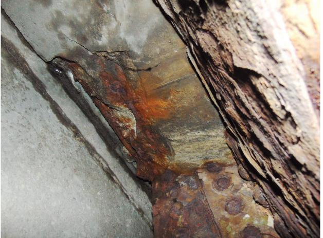
87 Heavy Wet Area with Large Delamination & Spalls at South Deck End, East of Stringer 5
