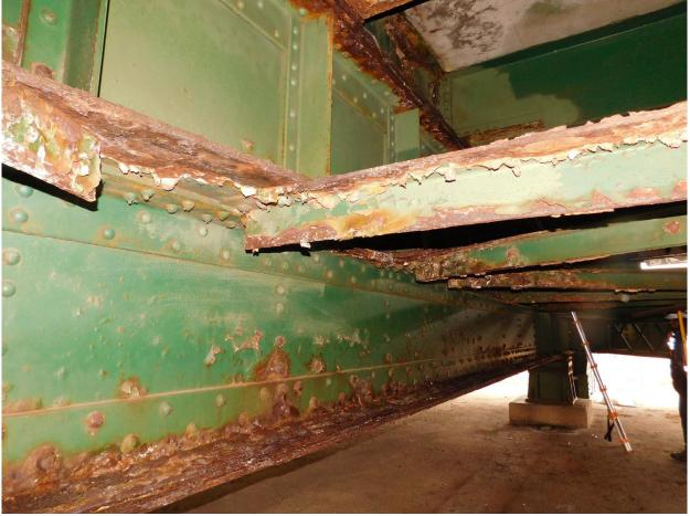
131 North Tower, Medium-Severe Corrosion on South Face of Rear Floor Beam, looking East
