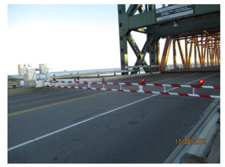
Photo E59 Typical Barrier Gate. Note the newly installed barrier gate, including arm light flasher and gong. The gate is in as-new condition.
