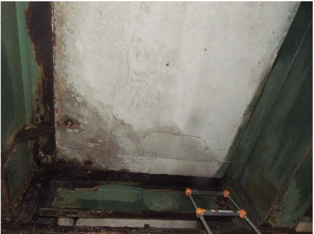
96 Wet Area & Delamination on Soffit between Stringers 3&4 near Exp Jt @ North End of North Tower Span Page A2 [48] of A2 [153]
