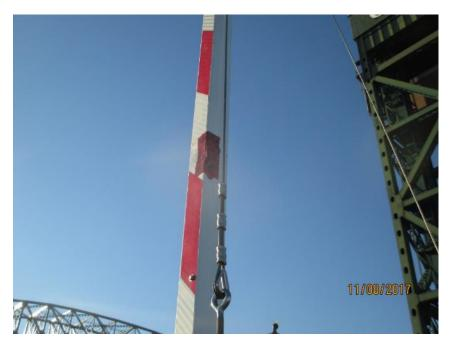
Photo E54 Damaged SE Traffic Gate Arm. Note the dent on the gate arm with a red tape is the result of the impact by a vehicle.
