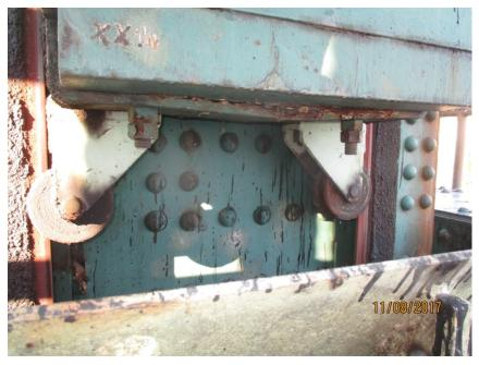
Photo M24 NE Auxiliary Counterweight. There are areas of light corrosion and paint deterioration on the counterweight blocks and frames.
