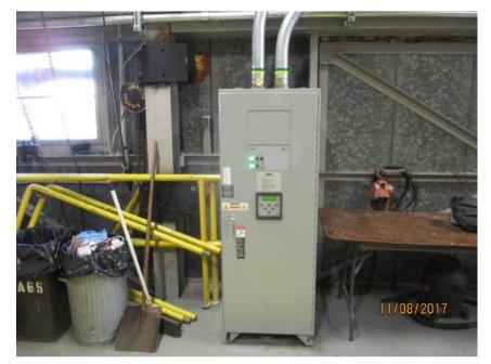
Photo E33 New Aerial Cable ATS in North Tower. The ATS was installed during the recent rehab project. It is used to automatically switch the aerial cable power feed between the east and west. The ATS is well installed.
