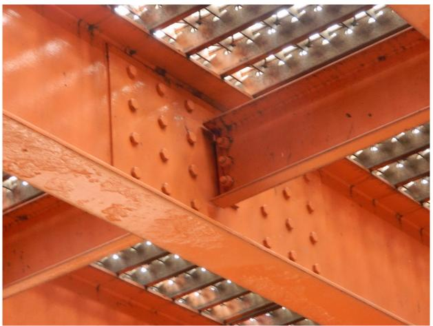
232 Typical Painted-Over Pitted Stringer Surface @ Lift Span
