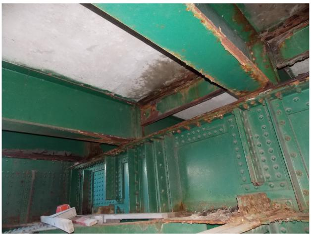
106 Wet Soffit & Heavy Corrosion on Steel below Expansion Joint @ South Approach & Tower Spans, looking SE Page A2 [53] of A2 [153]
