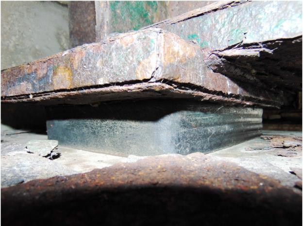
23 Minor Bulging of South Abutment Bearing under Stringer 2 (TYP)
