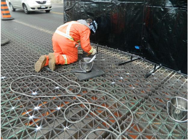
221 Emergency Welding Repairs of Severe Cracks & Broken Deck Grating (TYP)
