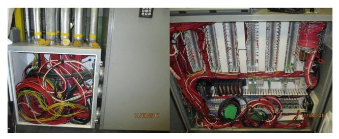
Photo E30 Inside of Pull Box and CP-3 Cabinet. Although the pull box was installed in addition to the control cabinet, both enclosures are over-congested.
