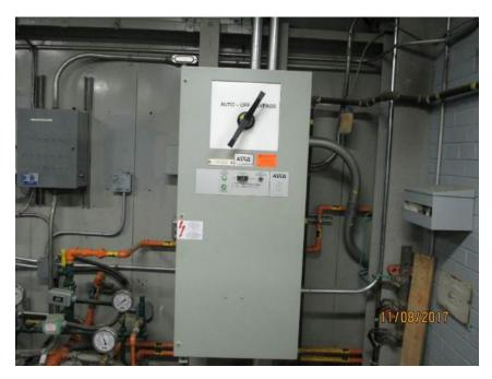
Photo E6 Automatic Transfer Switch (ATS). This ATS is used to automatically start the auxiliary generator to power the bridge facilities in the event of a power failure.
