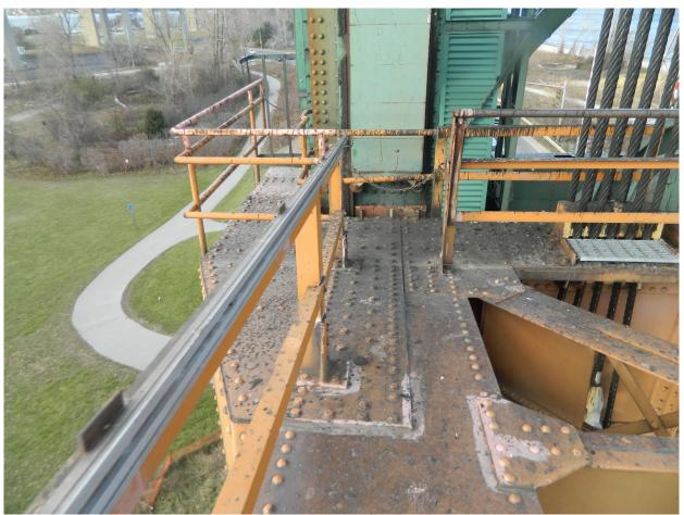
264 Typical Grease Stains on Top Corner of Truss, Northwest Corner Shown
