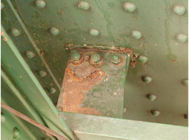
191 Typical Light-Medium Corrosion on Stand-off Bracket for Lower Platform, North Tower Shown
