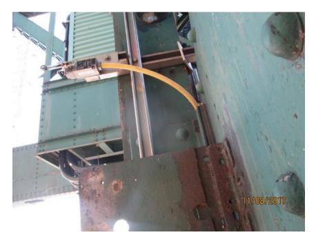
Photo E37 Typical Span Position Limit Switch. 3 span position limit switches have been installed on the south side along the counter weight traveling path: near seated, near open and full open limit. Note that these switches were configured in series with the programmable limit switch interfacing the span height resolver to create redundant/fail safe operation. However, the bridge operation is not fail safe without the positive indication from the north side of the span.
