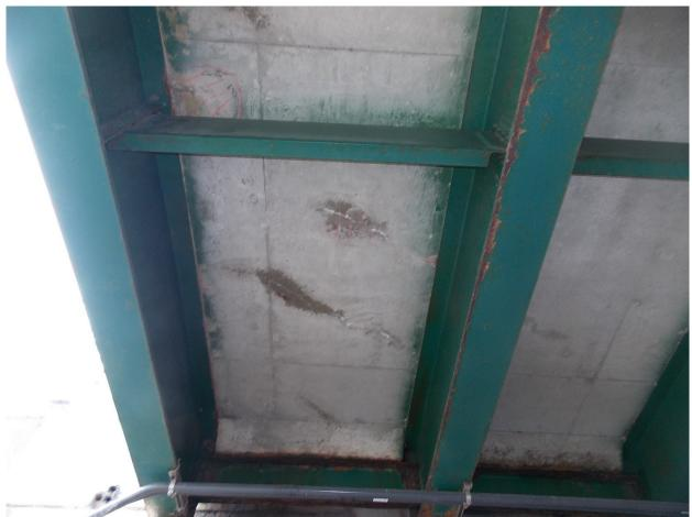
100 South Approach Span, Diagonal Stained Cracks with Delamination on Soffit @ Southeast Corner Area Page A2 [50] of A2 [153]
