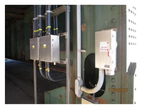
Photo E72 Existing Mobile Generator Disconnect and New Junction Boxes. Note the mobile generator disconnect with receptacle was the original installation. The disconnect switch and generator receptacle have never been used.
