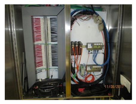
Photo E32 South Tower Aerial Cable Control Termination Box. The network switches and fiber patch boxes are also installed inside the box. Note the looped cables are the spare conductors and communication cables. All wires are well trained and installed.
