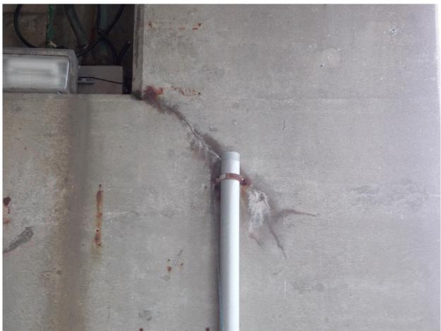
18 South Abutment, Wide Diagonal Crack with Wet & Efflorescence @ Top West Corner Area of Wall Page A2 [9] of A2 [153]
