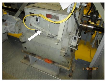
Photo M12 South Span Drive Reducer. The reducer auxiliary drive engagement lever is secured in position with a threaded position bolt (arrow). This bolt could not be rotated to test the south auxiliary drive engagement. Also, note that the reducer mounting bolts and support anchor bolts are unpainted.
