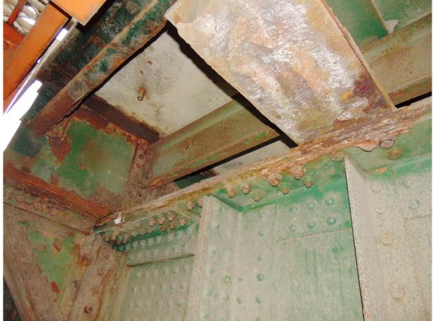
109 Wet Soffit & Heavy Corrosion on East Stringers below Open Gap Exp Joint @ NE corner of South Tower Span
