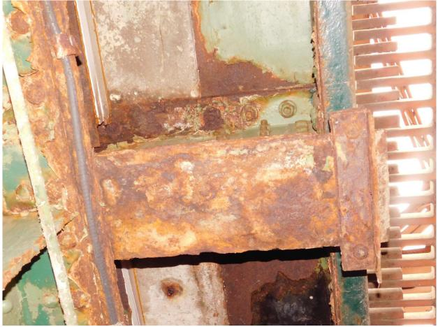
99 Wet Soffit & Heavy Corrosion on Stringer 4 below North Finger Plate Expansion Joint
