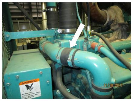
Photo M31 Main Generator. A coolant hose (arrow) exhibits dry rot and was starting to crack.
