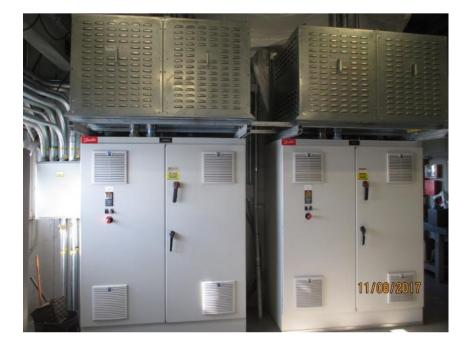
Photo E21 Typical VFD Drives Enclosure with Braking Resistors. Two new drives with resistors are installed in each tower. Both drives are in as new condition. Note two drives are providing redundancy for the main drive operation. Operator can select drives automatically or manually.
