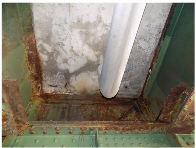
94 Large Wet Area with Spalls on Soffit @ SW Corner of North Approach Span
