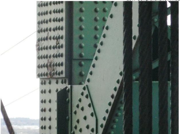
149 Typical Light Corrosion on Tower Column @ Coating Failure Spots, Southwest Column @ North Tower Shown
