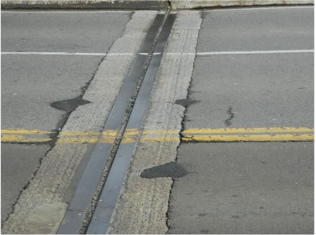
49 Cracks & Asphalt Patches at Exp Joint between South Approach & Tower Span, looking West
