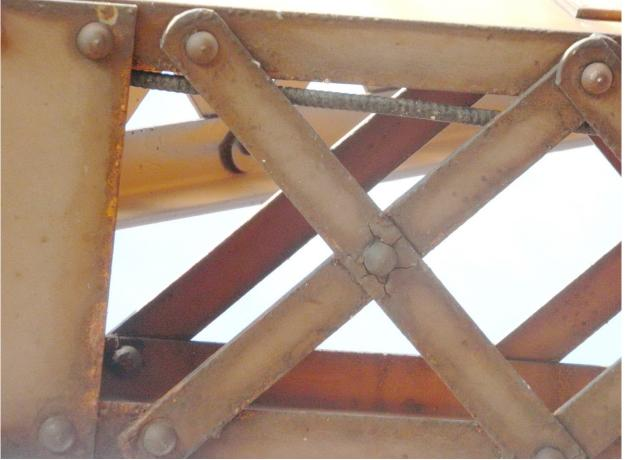
255 Typical Localized Paint Failure @ Lattice on Sway Frame Built-up Member
