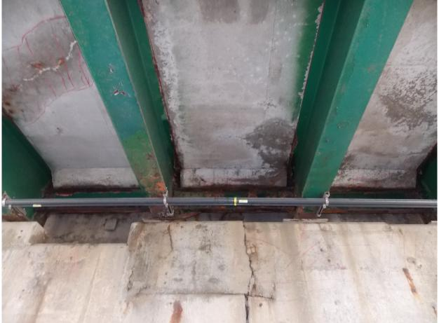
101 South Approach Span, Large Wet & Delam on Interior Soffit @ South Abutment
