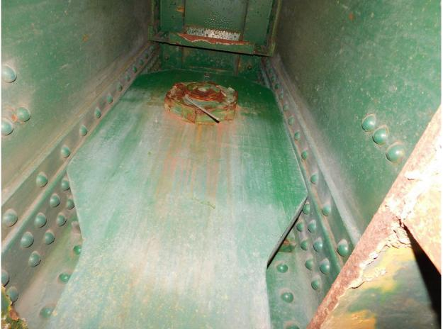
169 Light Surface Rust on Pin for Counter Weight Hanger Plates @ South Tower (TYP)
