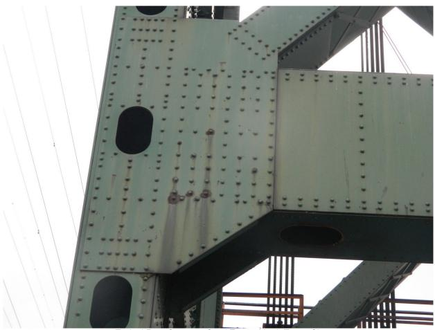
150 Typical Rust Spots on Steel Tower, North Tower Shown
