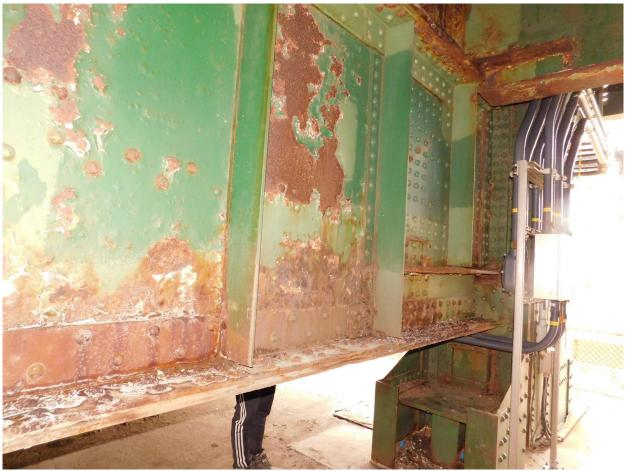
130 North Tower, Heavy Corrosion on North Face of Rear Floor Beam near NW Column Page A2 [65] of A2 [153]
