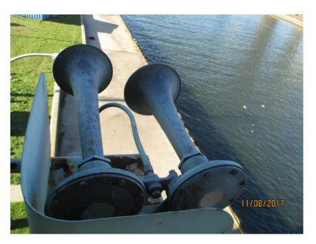
Photo E69 Typical Air Horn. The air horn is operational and is in serviceable condition. Note the corrosion on the air horn housing.
