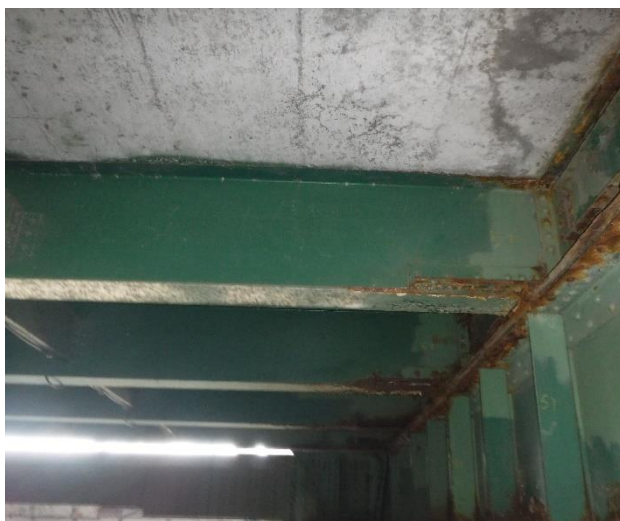
Stringers adjacent to Approach Span
