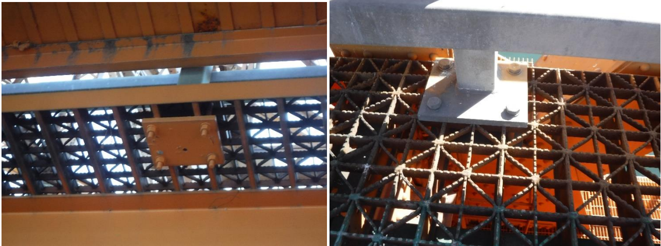
Figure 2: Existing Connection of Traffic Railing to Lift Span Deck
