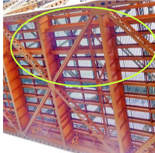
Typical Soffit (Rail Stringers Circled)
