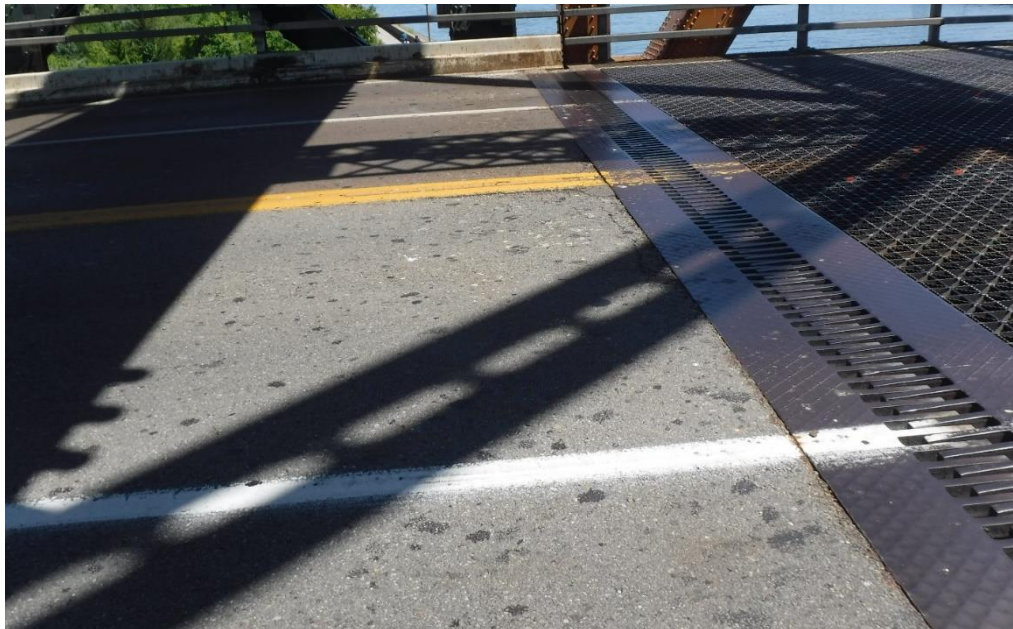
Figure 5 Finger Joint Connection
