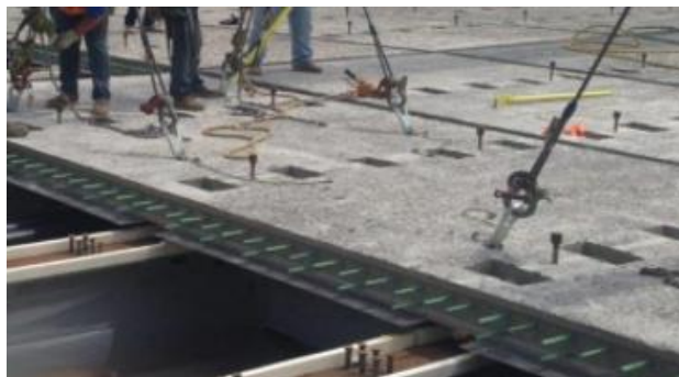
Figure 15: Precast concrete deck system 7
