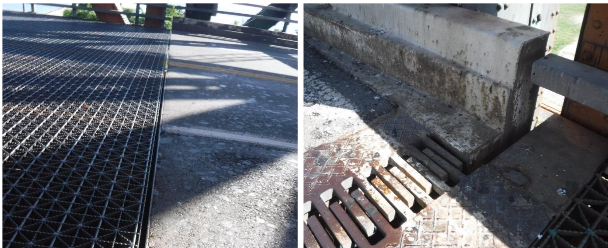
South End Joint with Lift Span
