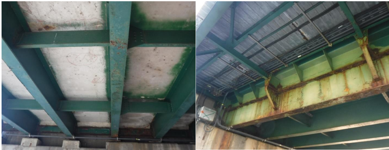
Figure 10. Typical Condition of Approach Span
