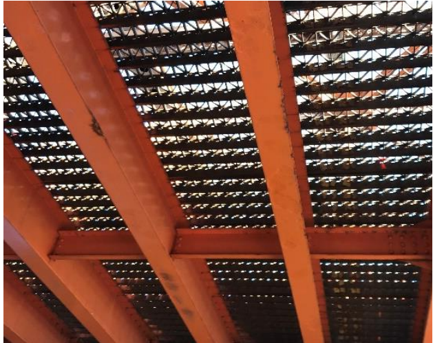
Typical Stringer Condition
