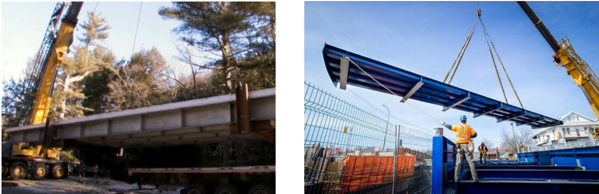
Figure 2: Craning of Deck on Stringers 2
