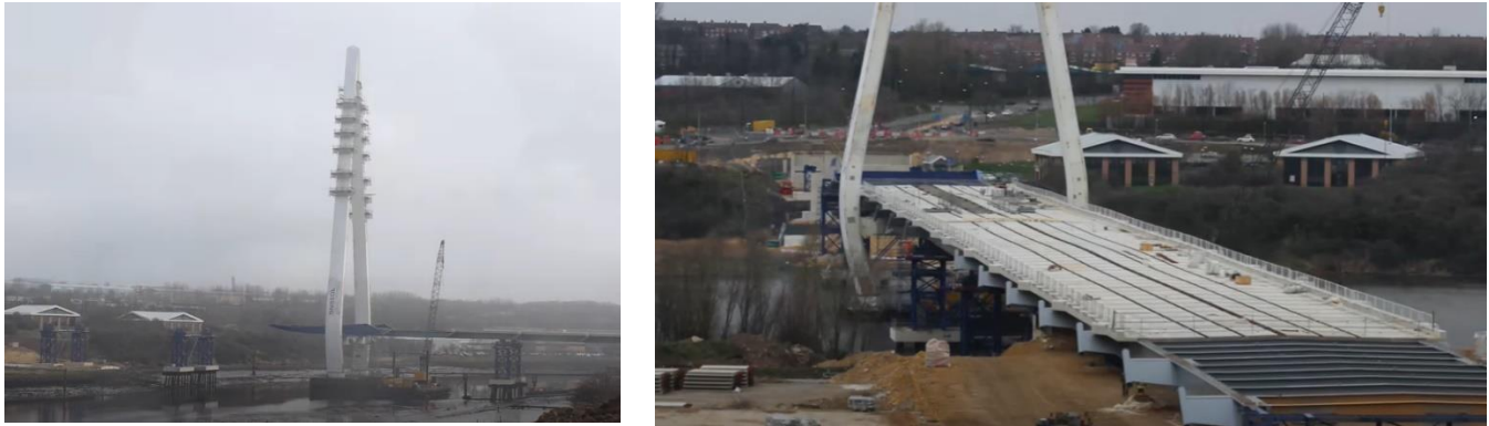
Figure 3: Launch of Bridge Deck 3
