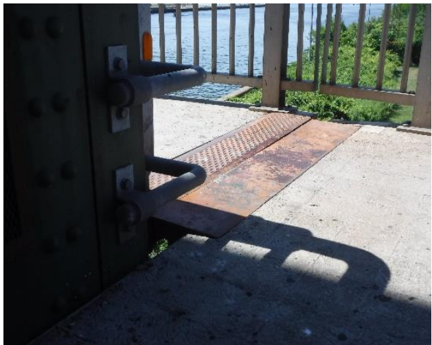
Figure 4. Sidewalk Expansion Joints
