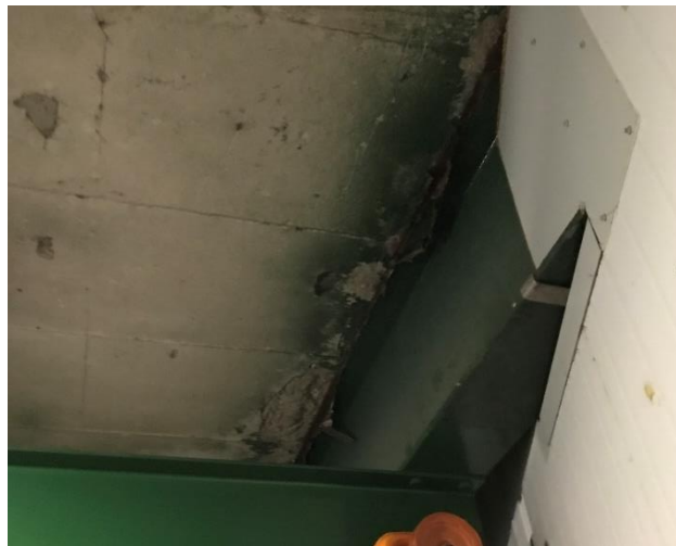
Inside the Span Lock Room
