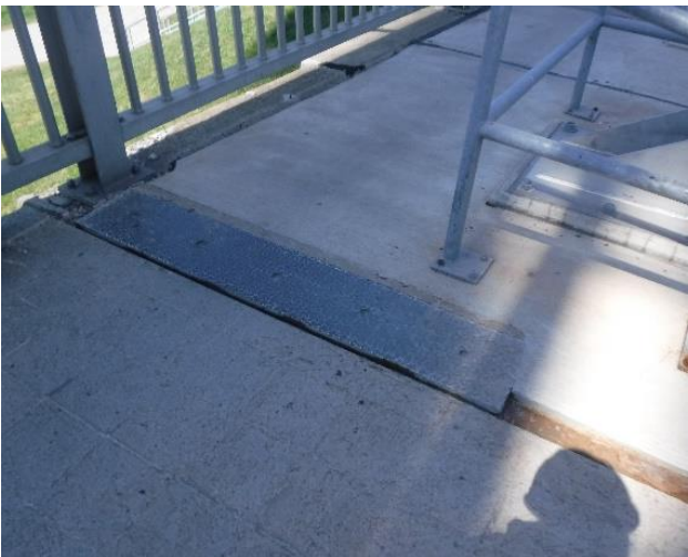
Figure 4. Sidewalk Expansion Joints
