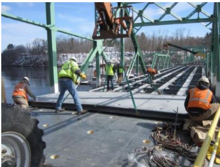
Figure 14: Fiber-reinforced polymer bridge decks supplied by Composite Advantage 15
