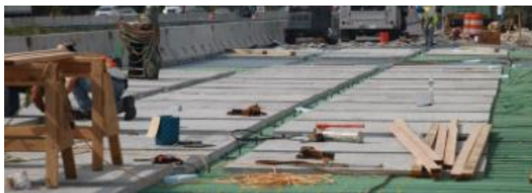
Figure 10: Concrete half-filled grid installation 7
