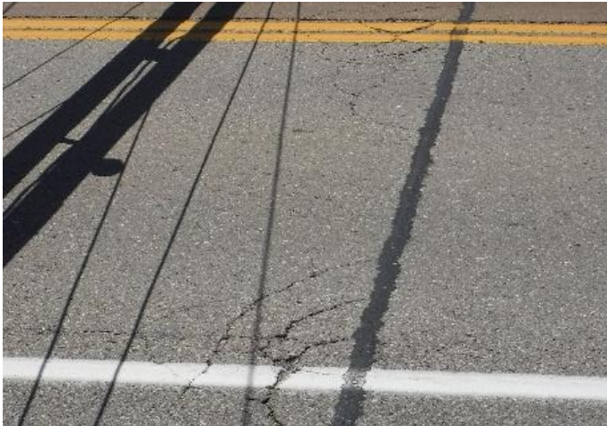
Figure 11 Typical Paved over Joint at Abutment
