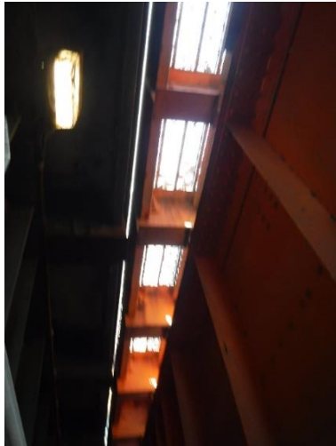
Underside of South End Joint with Lift Span
