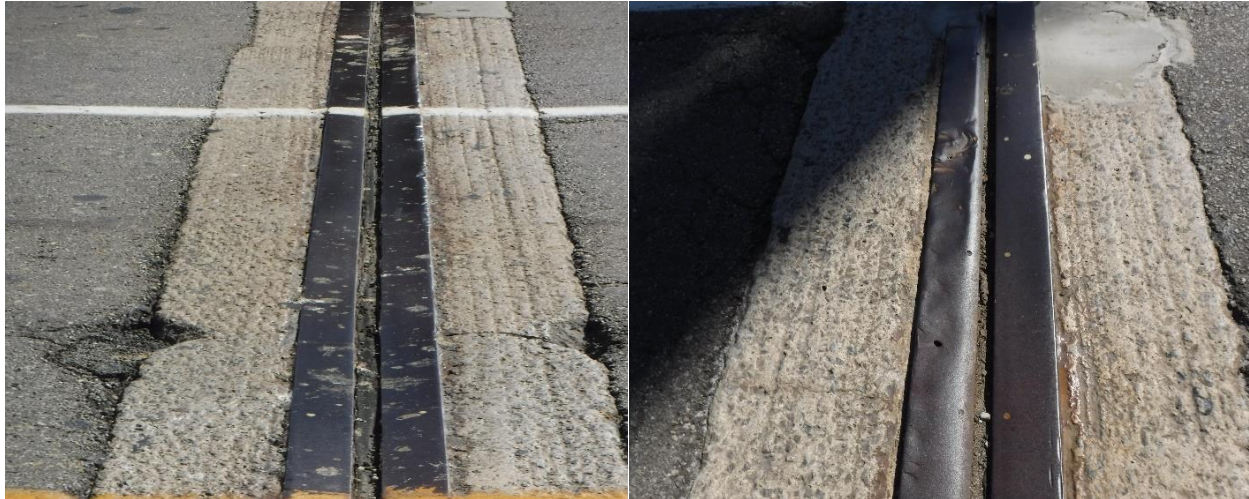
South Expansion Joint
