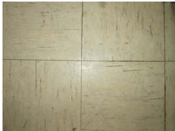
Figure 5 - The 12"x12" floor tiles in the office on the 2nd floor of the Main Garage Building contain asbestos (Sample 17).
