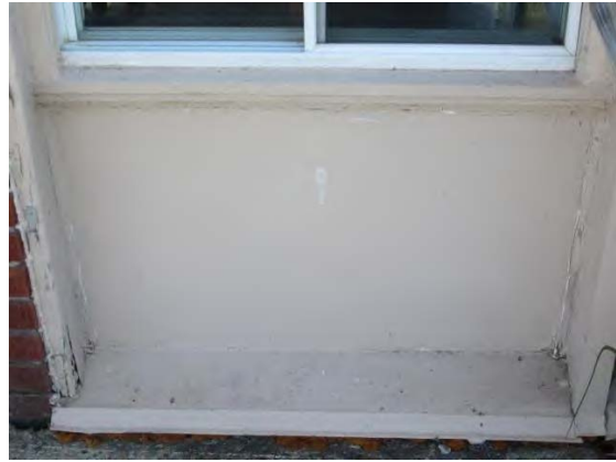
Figure 4 - Transite panels were observed under and over exterior windows of the Administration Building. This material contains asbestos according to Sample 14.
