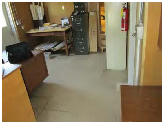
Figure 6 - Another view of the ACM floor tiles in the Garage Office.
