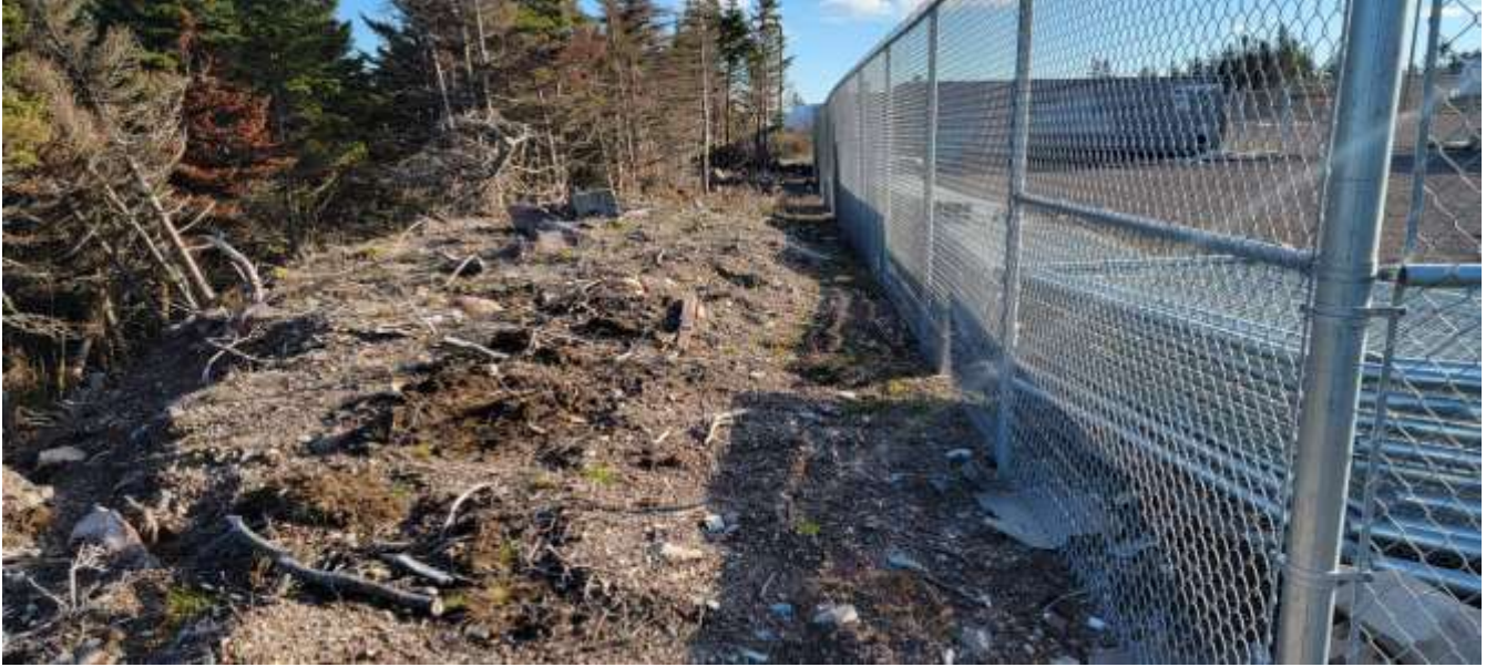
Photos 8: North side of storage pad
