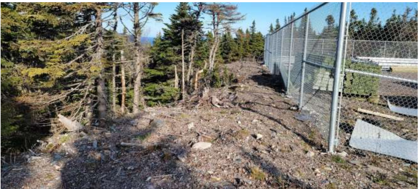
Photo 7: NW side of storage pad
