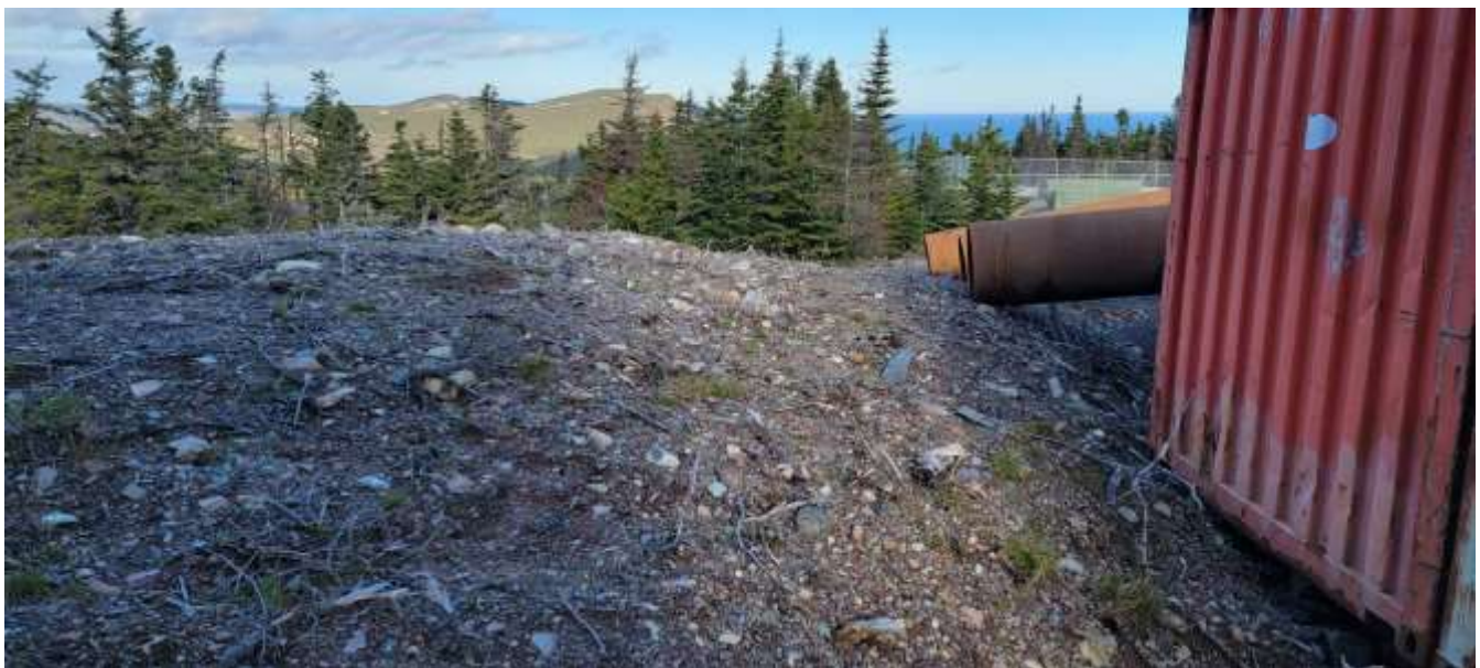
Photo 5: West side of storage pad
