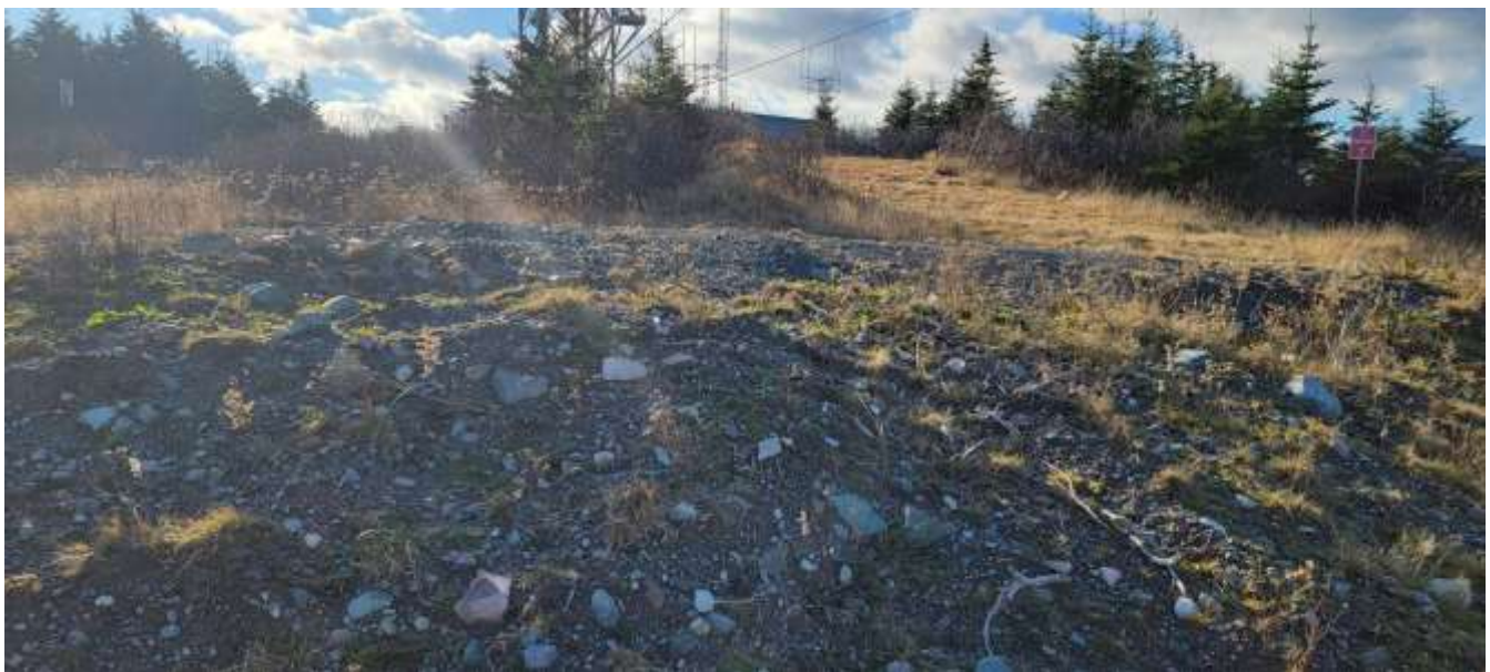
Photo 3: Buried 4800V (encased in concrete) see raised berm center
