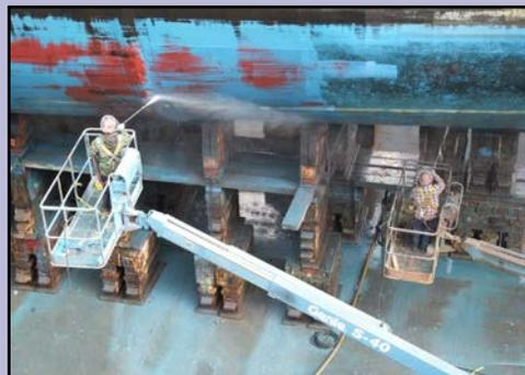
*Conventional pressure washing and ultra high pressure (UHP) washing use large amounts of water at high pressure to scour paint and biological material from the hulls of ships.*
