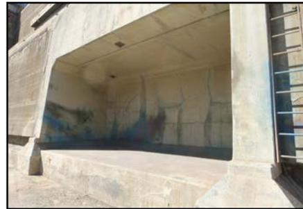
*Paint overspray due to INADEQUATE containment stabilizer pocket doors.*
