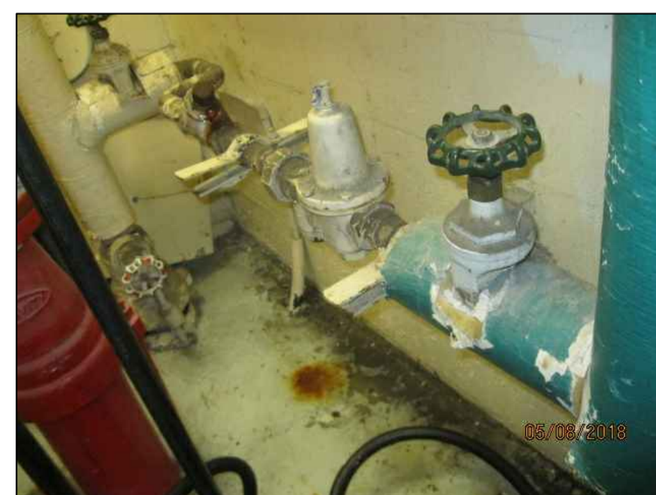
SEGREGATION UNIT - RELEVANT PHOTOS SCALE: NTS
