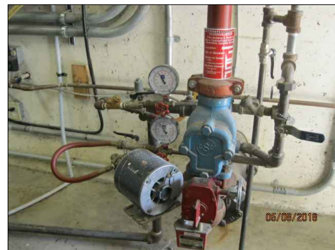
BUILDING LU5 - RELEVANT PHOTOS SCALE: NTS
