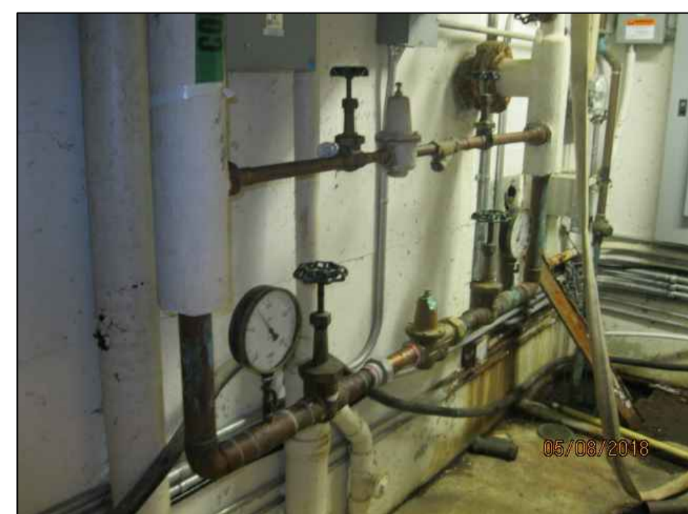
BUILDING LU5 - RELEVANT PHOTOS SCALE: NTS
