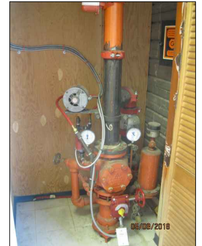
MAINTENANCE BUILDING - RELEVANT PHOTOS SCALE: NTS
