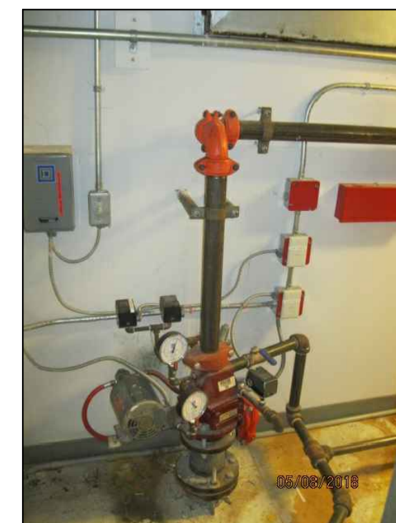
JENSEN BUILDING - RELEVANT PHOTOS SCALE: NTS
