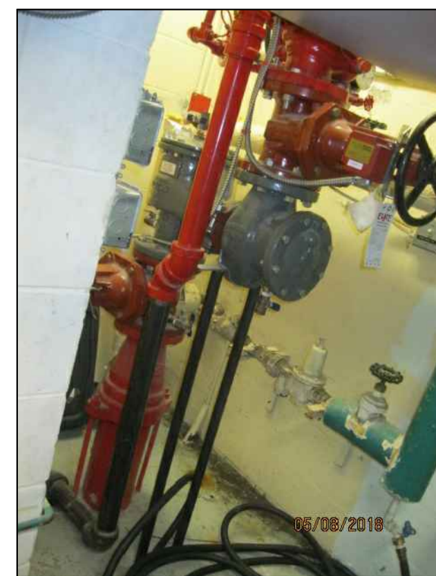
SEGREGATION UNIT - RELEVANT PHOTOS SCALE: NTS
