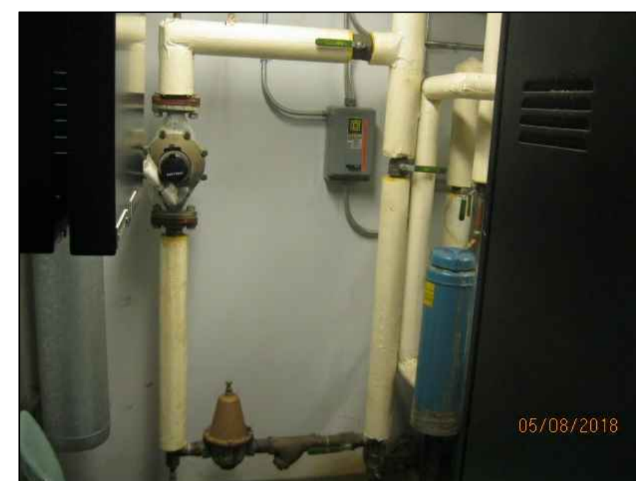
JENSEN BUILDING - RELEVANT PHOTOS SCALE: NTS
