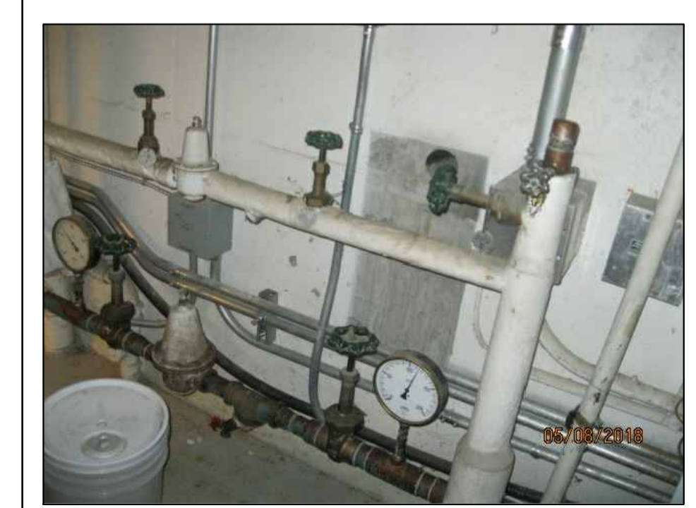
BUILDING LU4 - RELEVANT PHOTOS SCALE: NTS
