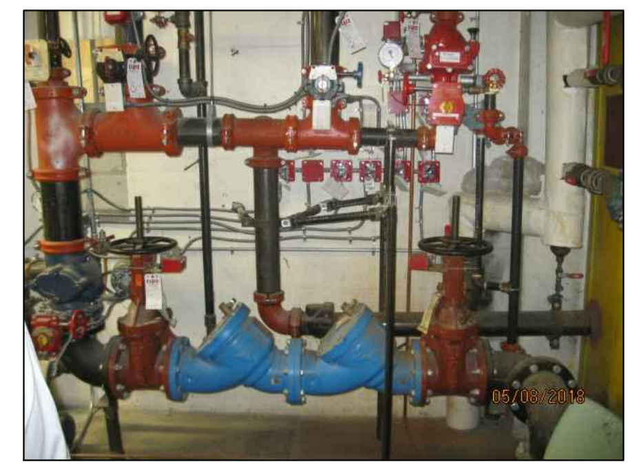
ADMIN BUILDING - RELEVANT PHOTOS SCALE: NTS
