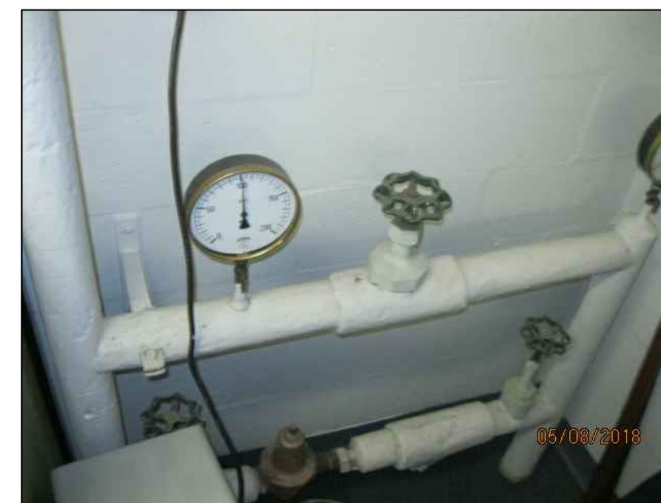
MAINTENANCE BUILDING - RELEVANT PHOTOS SCALE: NTS
