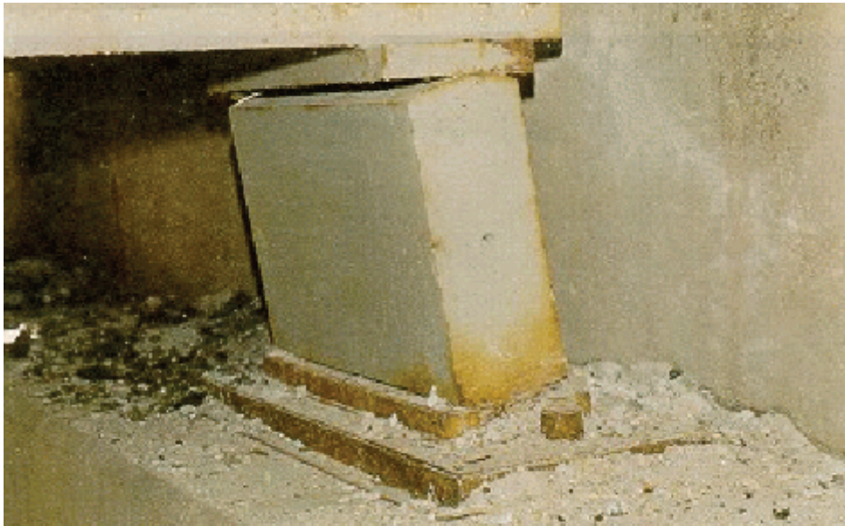
Figure A4.1.2(f) Steel Rocker Bearing
