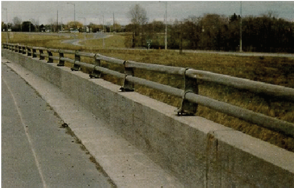
Figure A8.1.2(a) Parapet Wall
