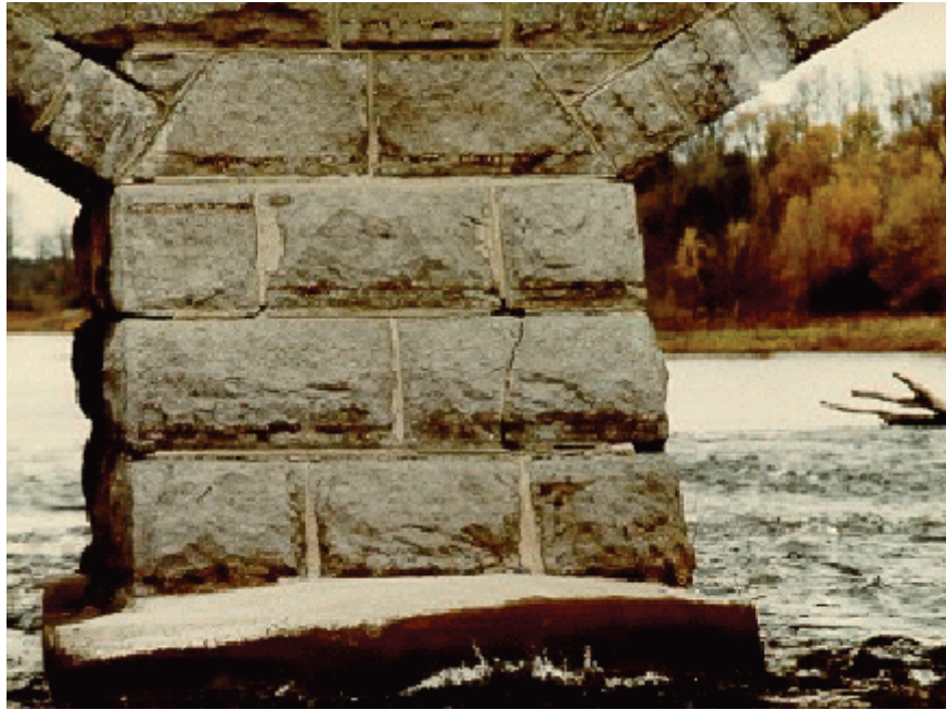
Figure A3.1.2(m) Masonry Pier
