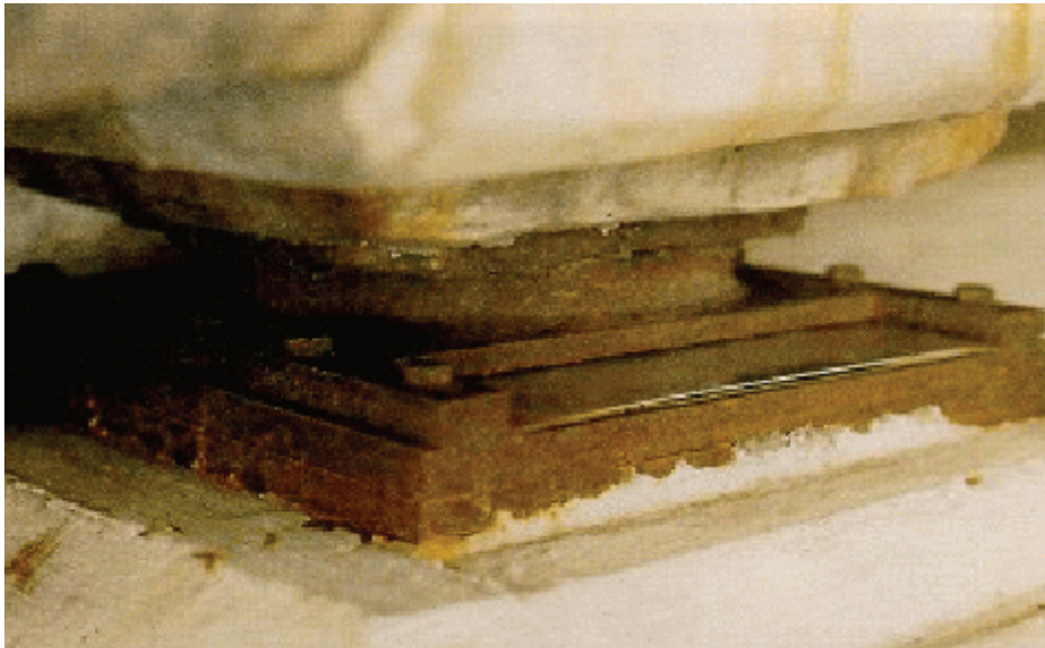
Figure A4.1.2(d) Disc Bearing
