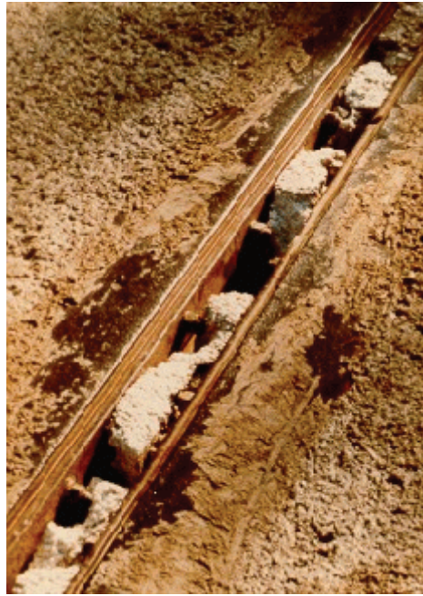
Figure A5.1.3(g) Horizontally Bolted Seal
