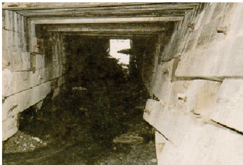
Figure A6.1.2(n) Wood Culvert
