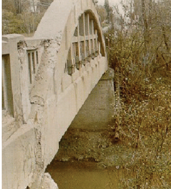
Figure A6.1.2(i) Concrete Bowstring Arch
