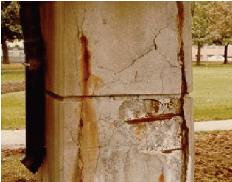
Figure A3.1.2(i) Concrete Pier Column
