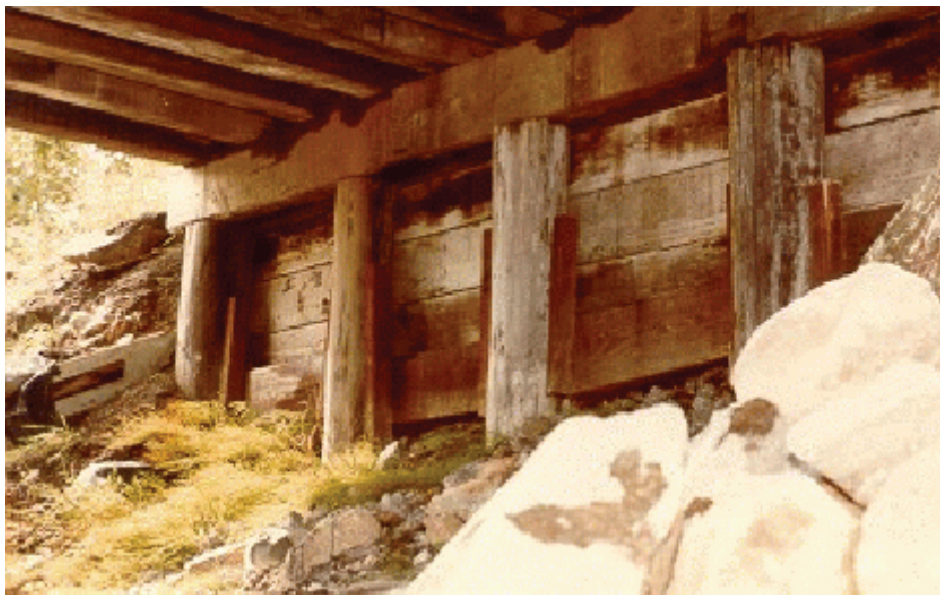
Figure A3.1.2(f) Wood Lagging – Abutment Wall
