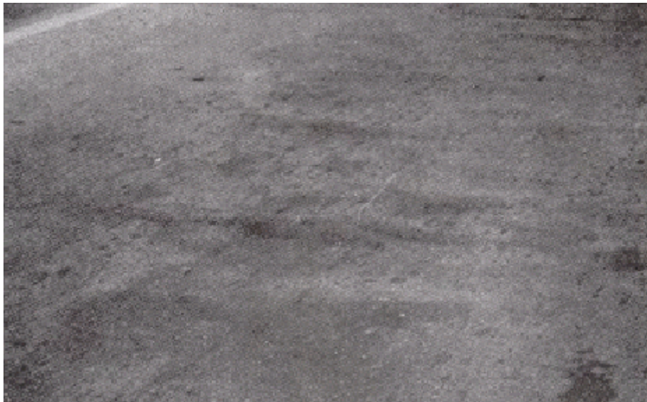
Figure 2.7.6 Severe Rippling
