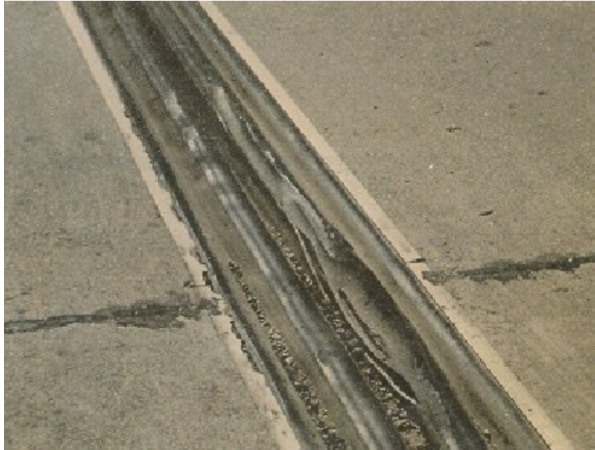
Figure A5.1.3(e) Multiple Seal Joint
