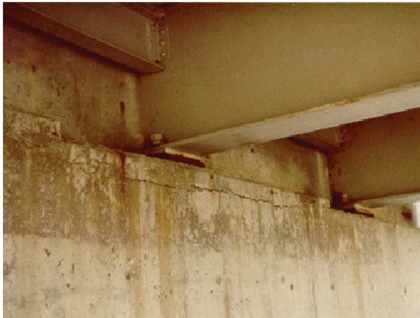
Figure A3.1.2(t) Concrete Bearing Seats
