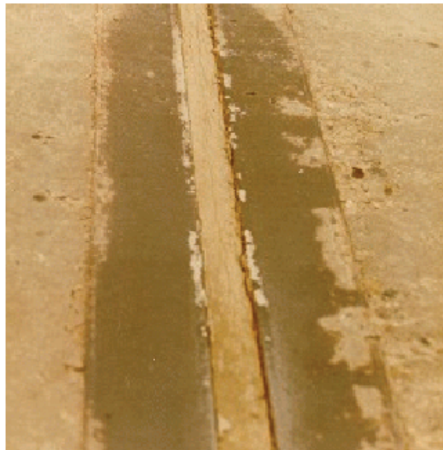
Figure A5.1.3(d) Ethylene Vinyl Acetate Seal
