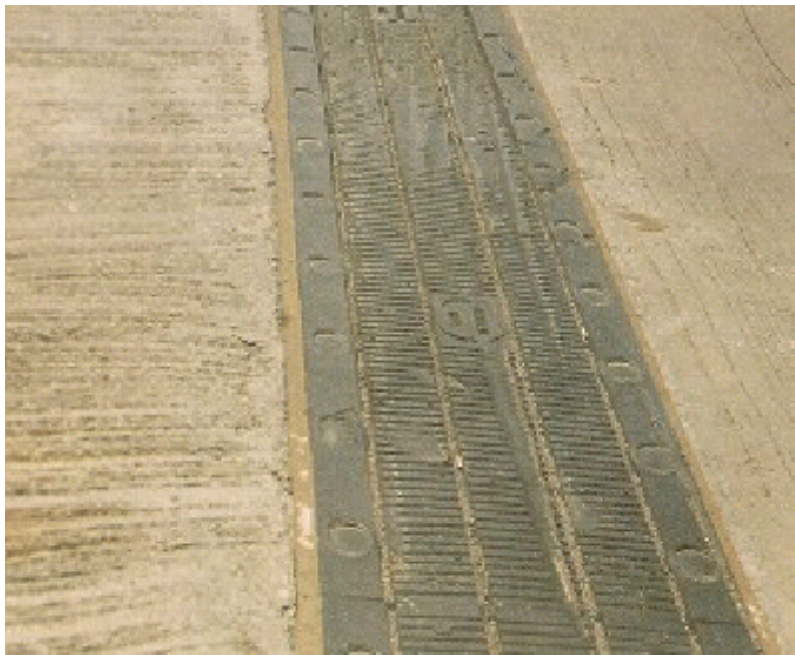
Figure A5.1.3(f) Rubber Cushion Joint
