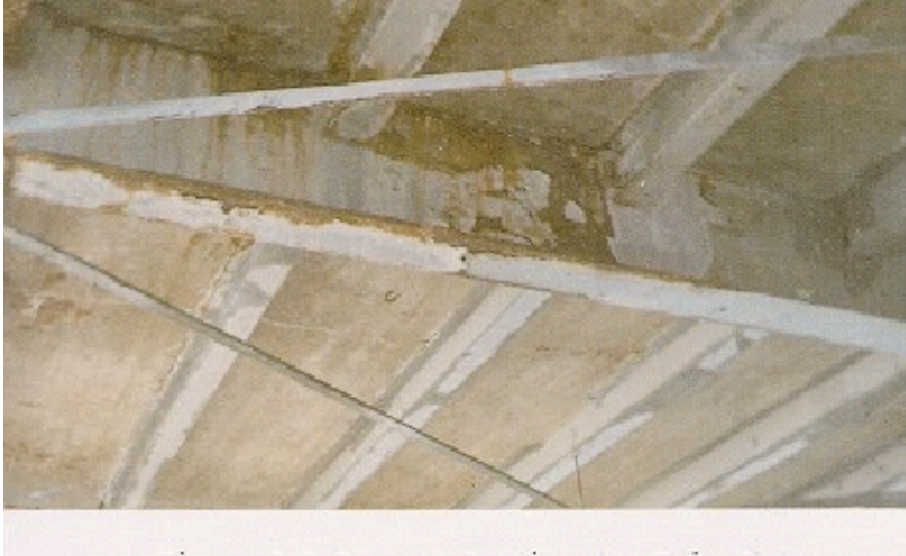
Figure A7.1.2(e) Soffit of a Thin Slab
