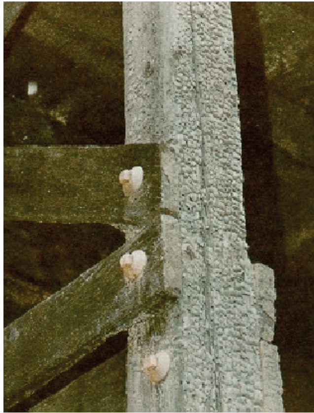
Figure 2.4.6(a) Medium Fire Damage on Wood
