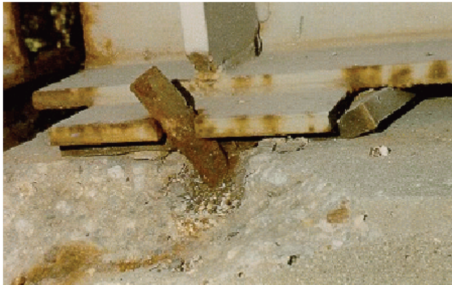
Figure A4.1.2(b) TFE Elastomeric Bearing
