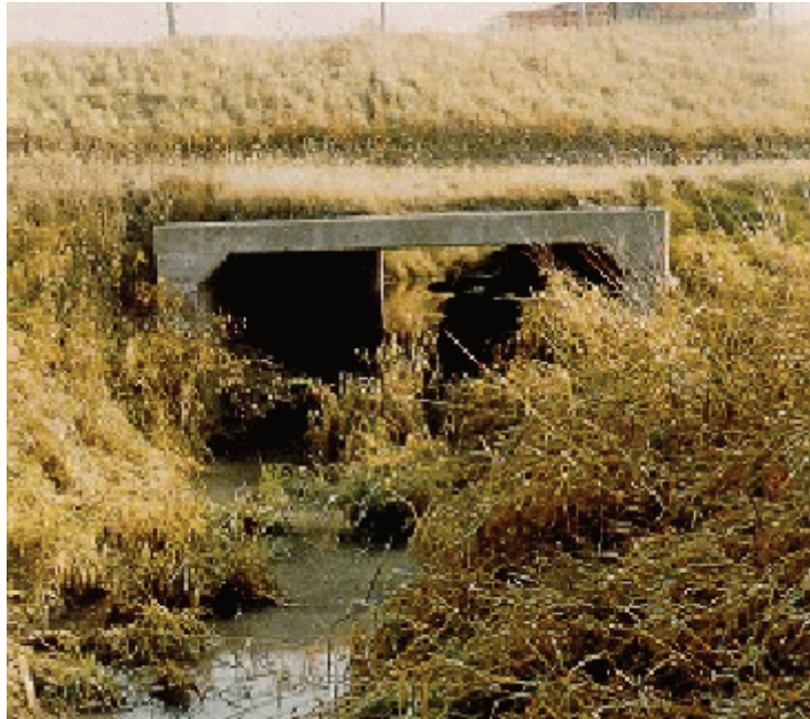
Figure A6.1.2(k) Concrete Open Footing Culvert
