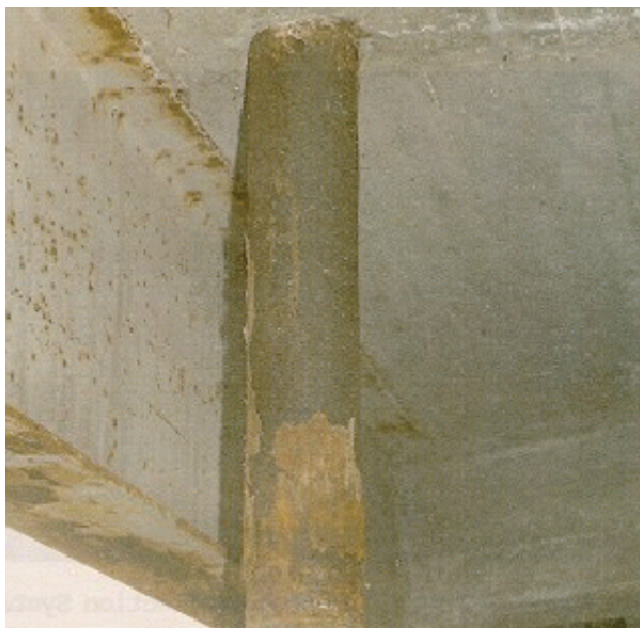
Figure A7.1.2(n) Steel Deck Drain
