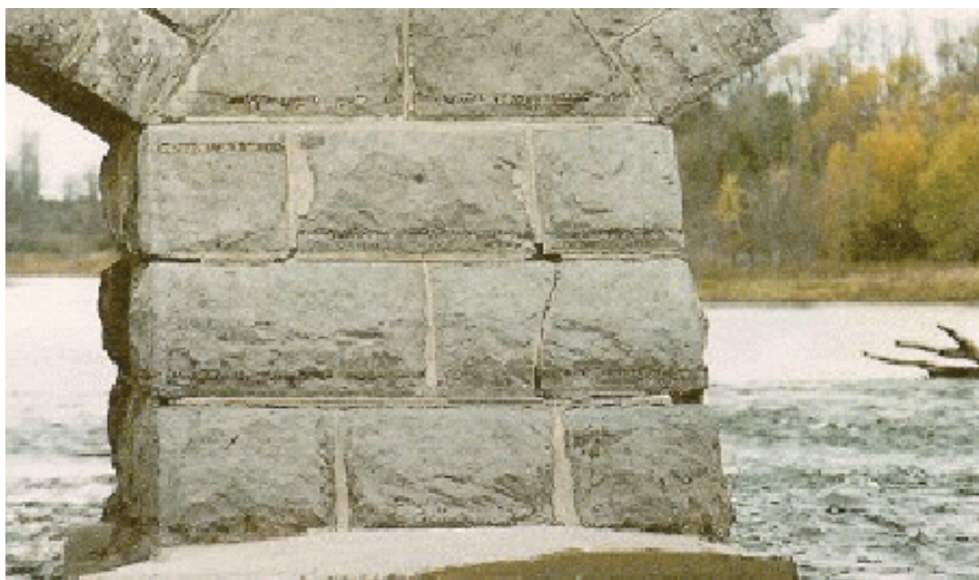
Figure 2.5.1 Wide Crack Through a Stone in a Masonry Pier
