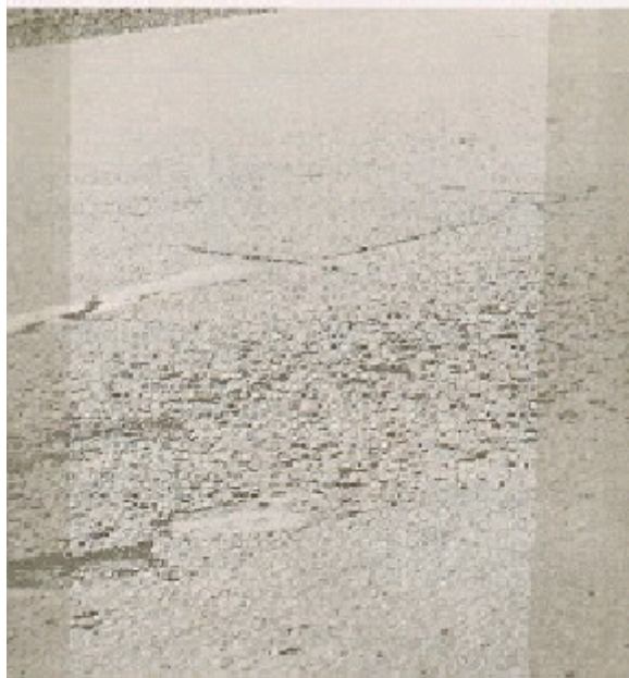
Figure 2.7.2 Severe Ravelling
