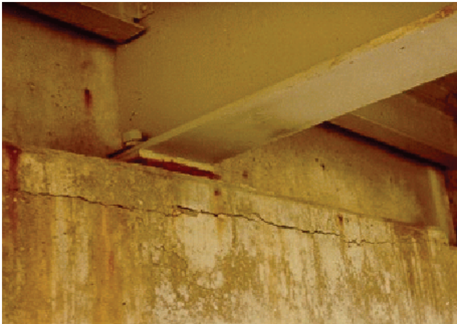
Figure A3.1.2(p) Concrete Ballast Walls
