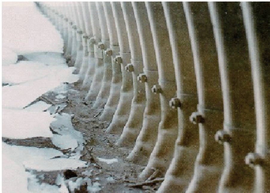
Figure A6.1.2(l) Multi-plate Pipe Arch
