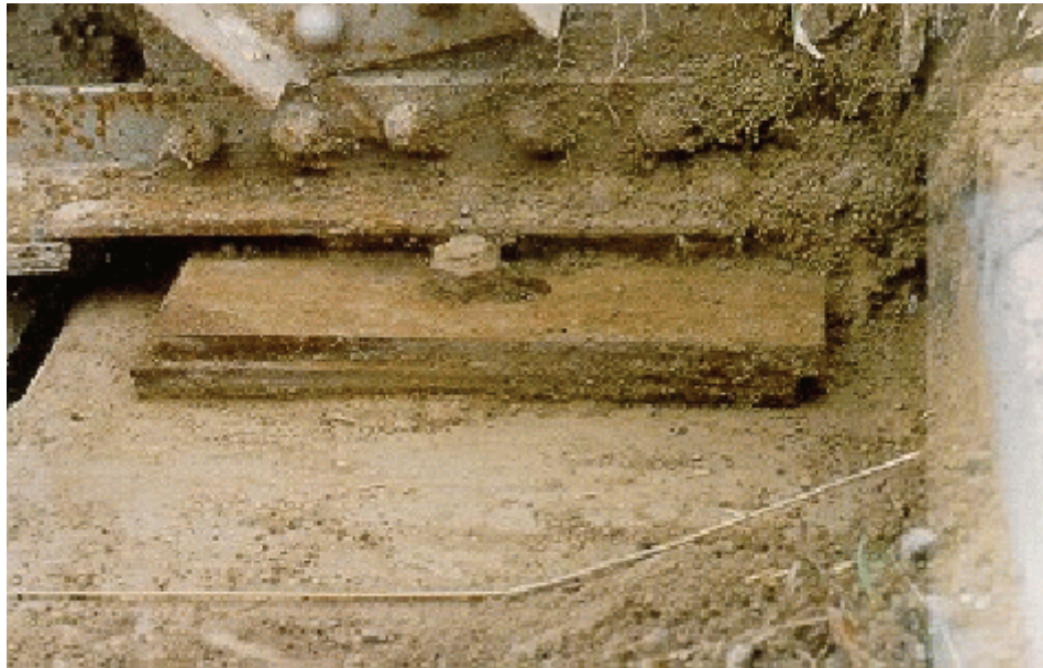
Figure A4.1.2(a) Steel Plate Sliding Bearing
