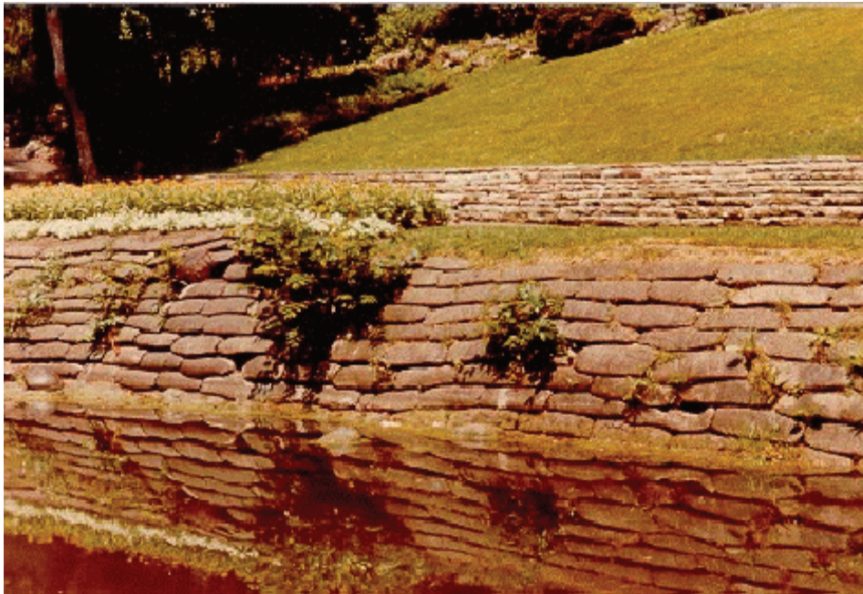
Figure A3.1.2(s) Bag Mortar Retaining Wall
