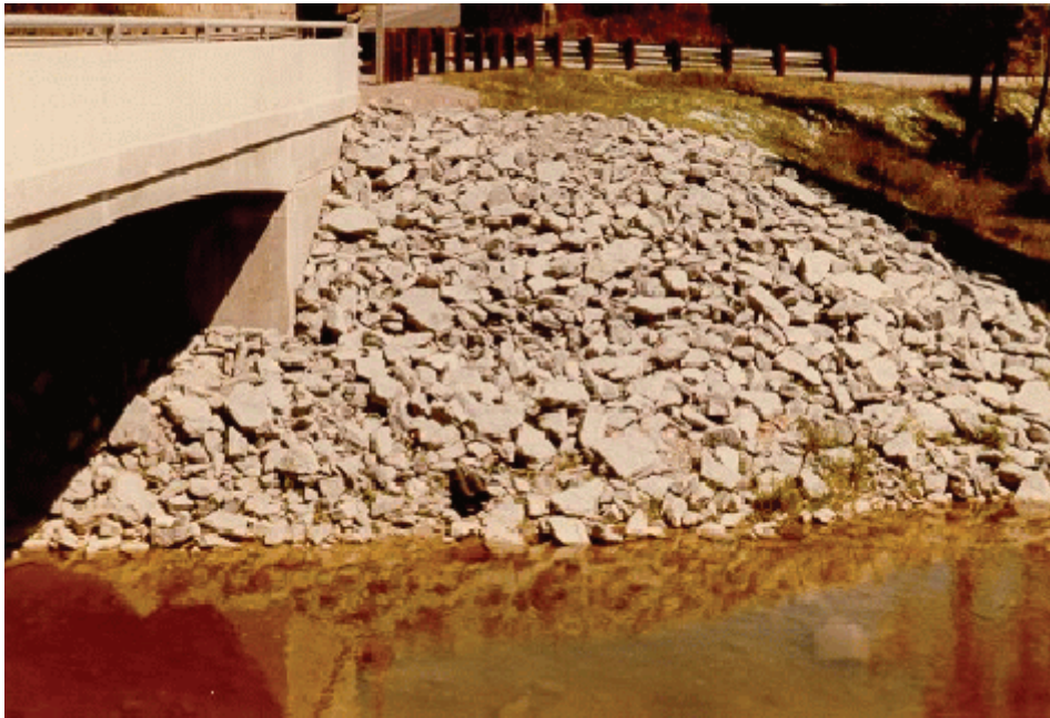
Figure A2.2.2(a) Random Rip-Rap Slope Protection
