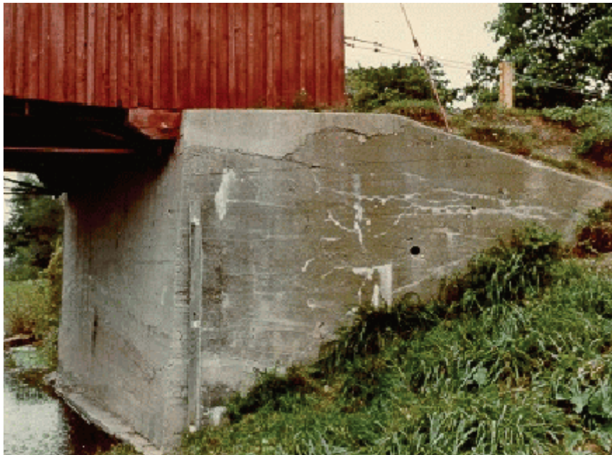
Figure A3.1.2(n) Concrete Wingwall
