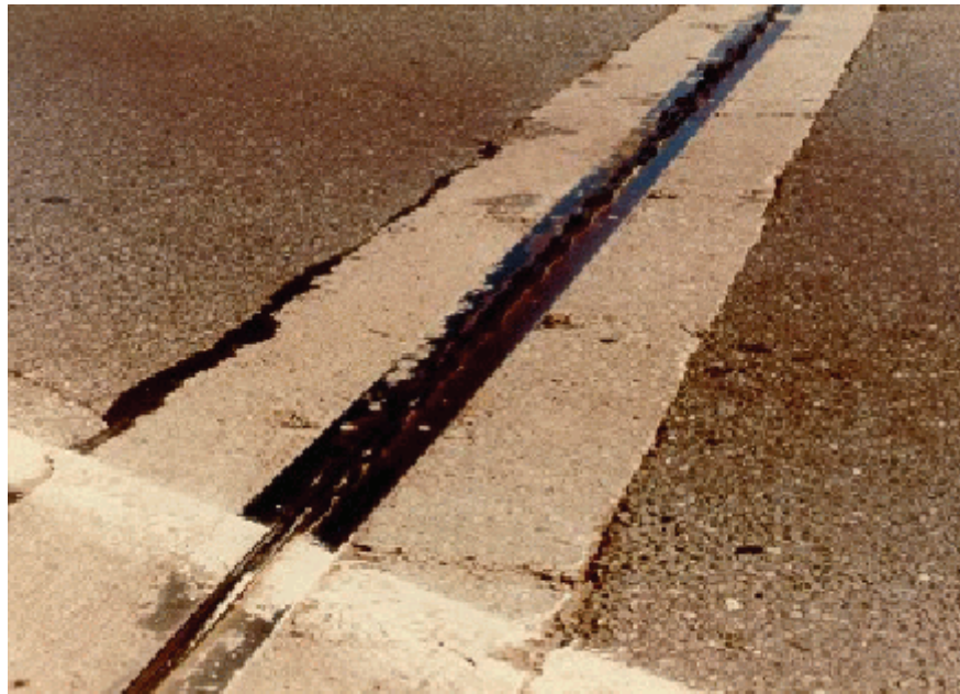
Figure A5.1.3(b) Compression Seal Joint
