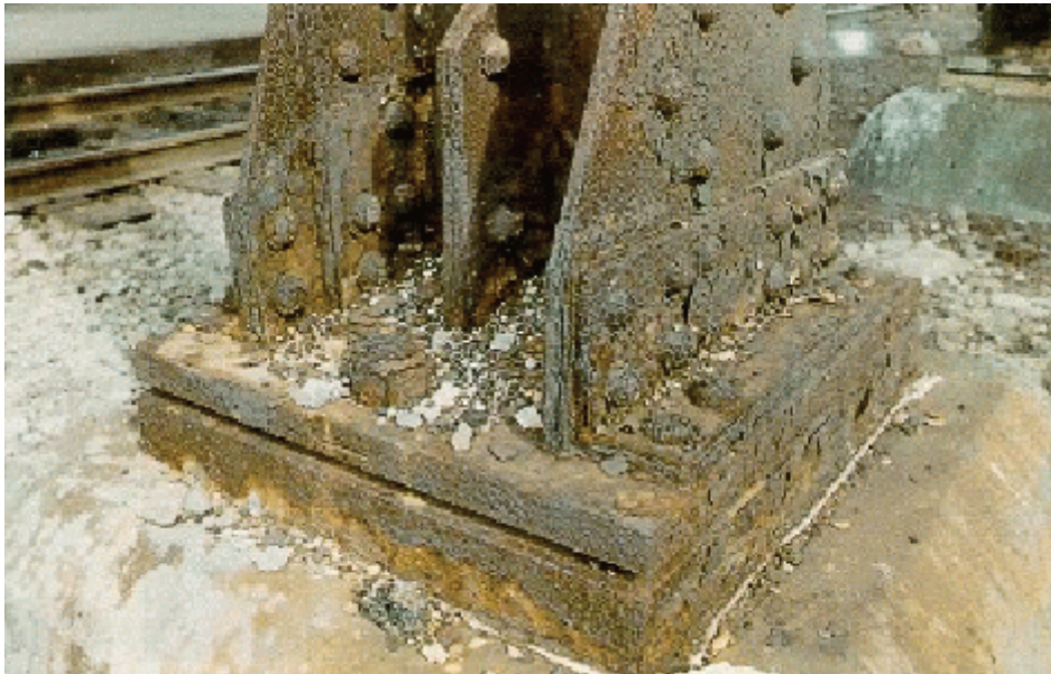
Figure A3.1.2(k) Steel Pier Bent Base
