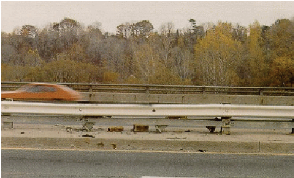
Figure A8.1.2(h) Steel Flex Beams
