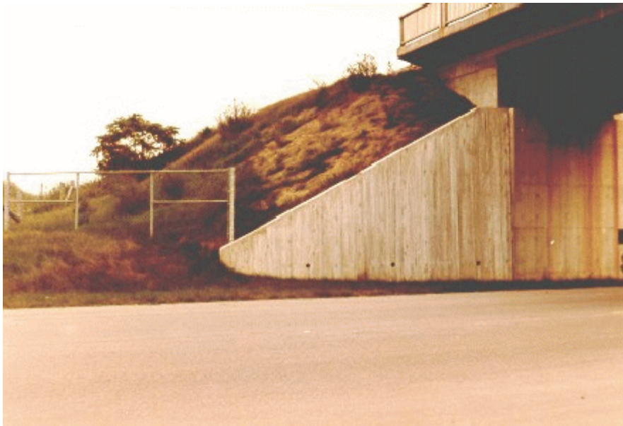
Figure A2.2.2(b) Grass Slope Protection
