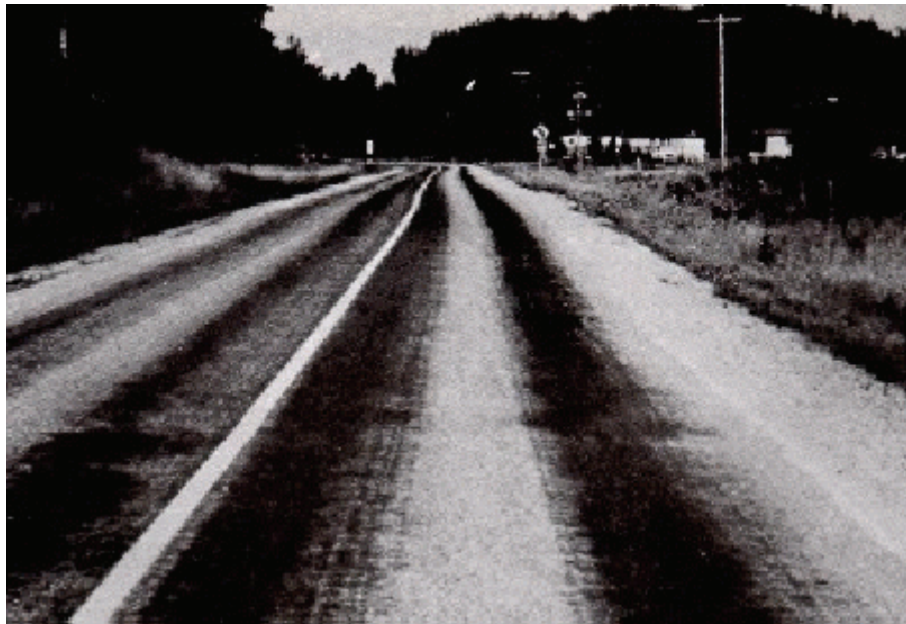
Figure 2.7.8 Slippery Surface
