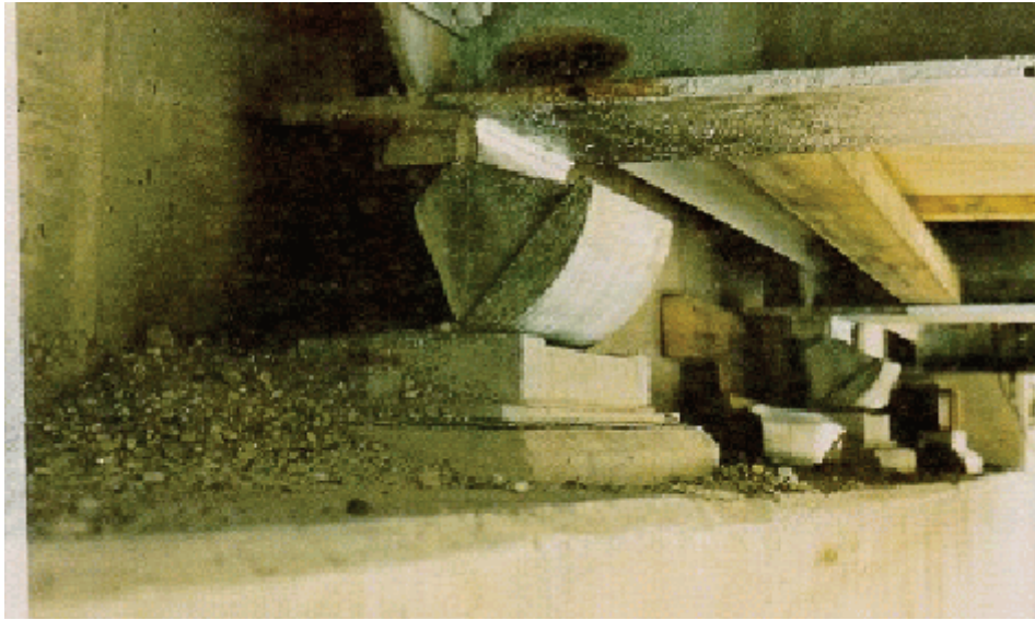
Figure A4.1.2(g) Steel Rocker Bearing
