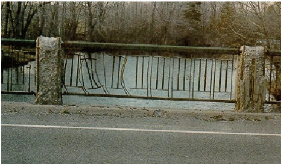
Figure A8.1.2(f) Steel Railing with Concrete Posts
