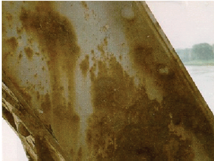
Figure 2.8.2(a) Undercutting
