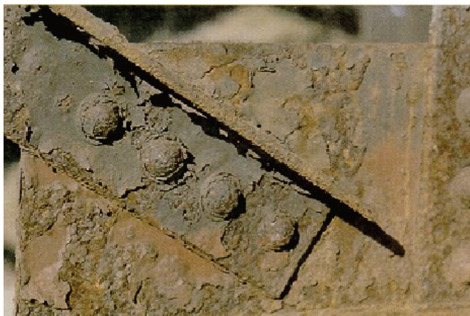
Figure A6.1.2(r) Sway Frame Connection
