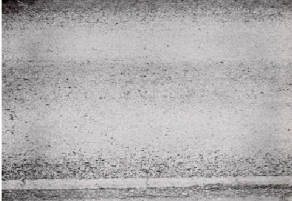
Figure 2.7.7 Severe Flushing
