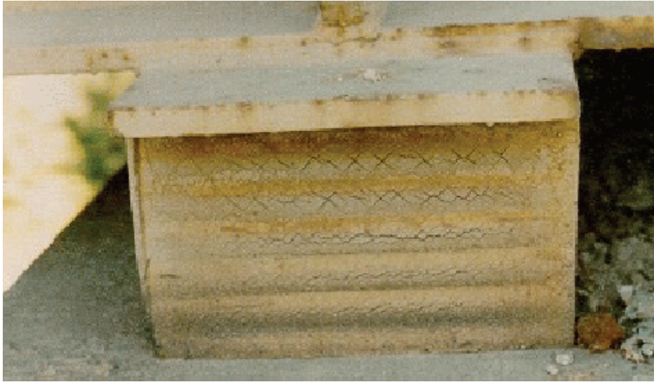
Figure A4.1.2(c) Laminated Elastomeric Bearing
