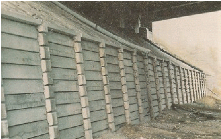
Figure A3.1.2(r) Precast Concrete Retaining Wall
