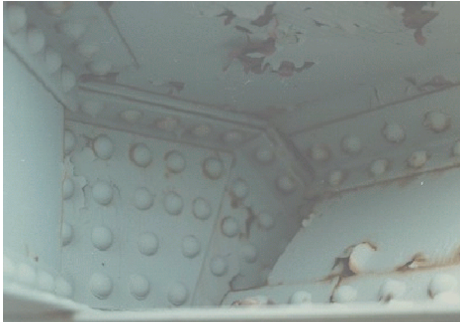
Figure A9.1.4(b) Connection of Primary Components
