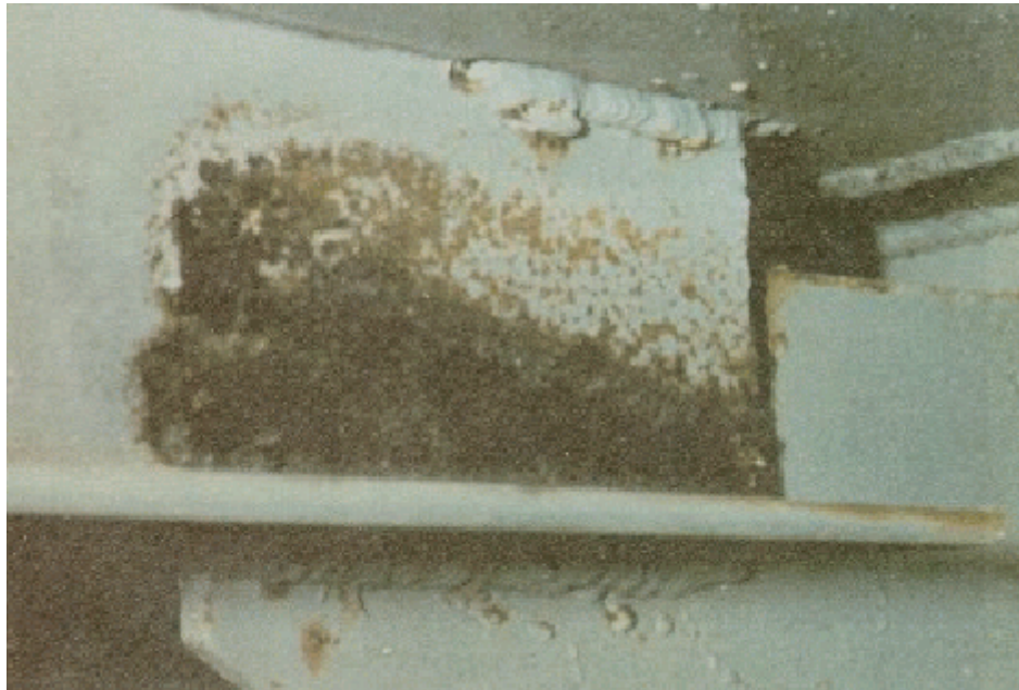
Figure 2.8.1(d) Chemical Attack
