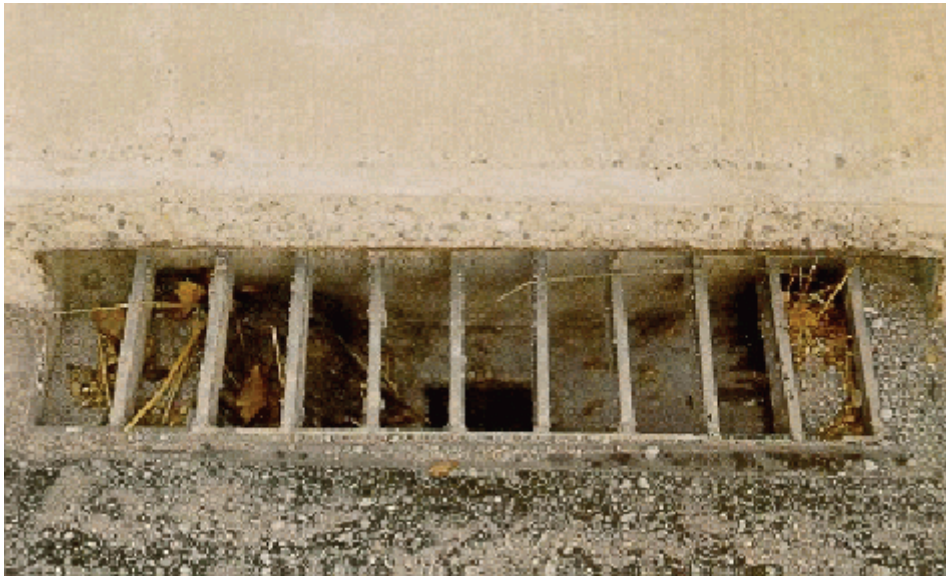
Figure A7.1.2(o) Deck Drain With Basin
