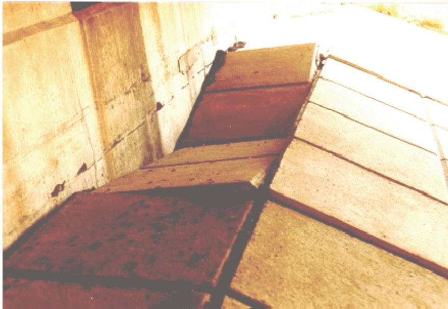
Figure A2.2.2(c) Cast-In-Place Concrete Slope Protection
