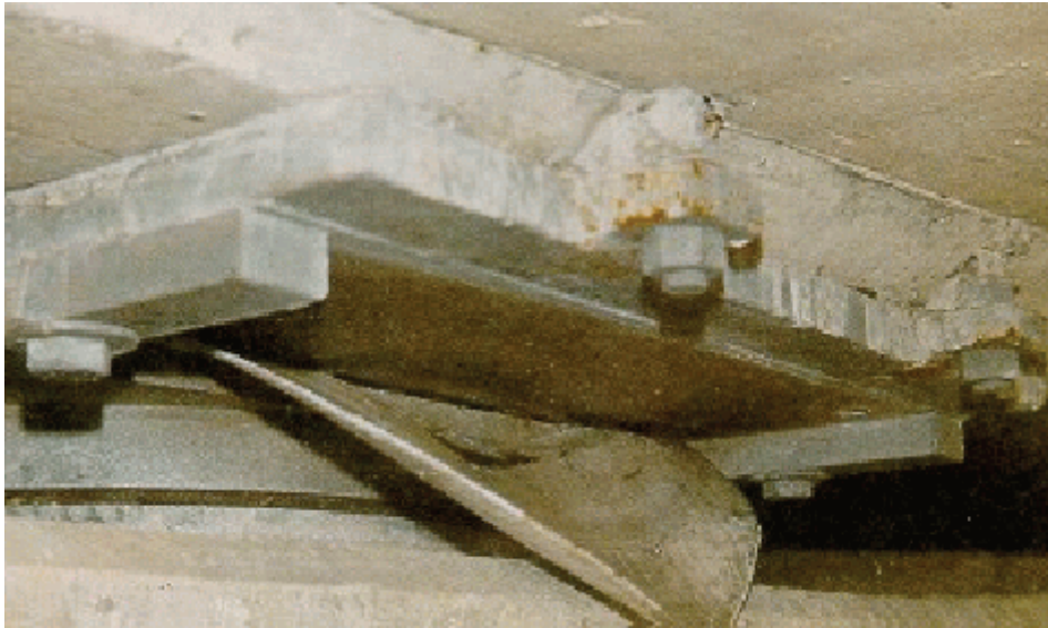
Figure A4.1.2.(e) Pot Bearing
