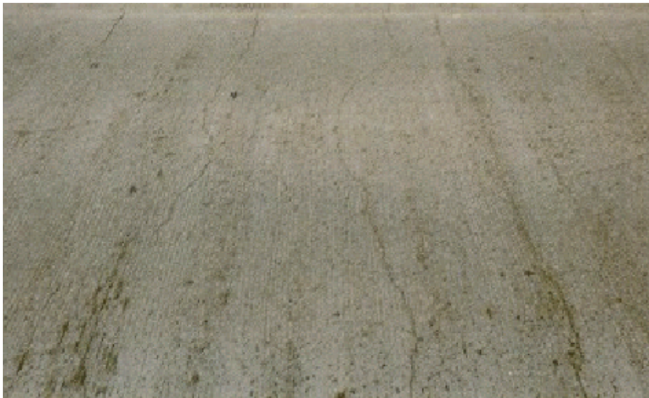
Figure A7.1.2(b) Exposed Concrete Deck
