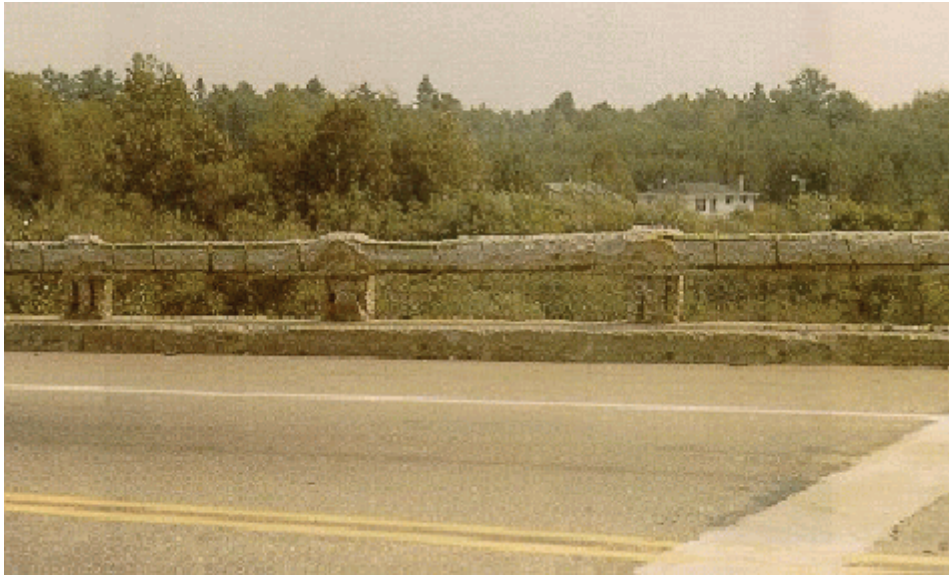
Figure A8.1.2(g) Concrete Guide Rail
