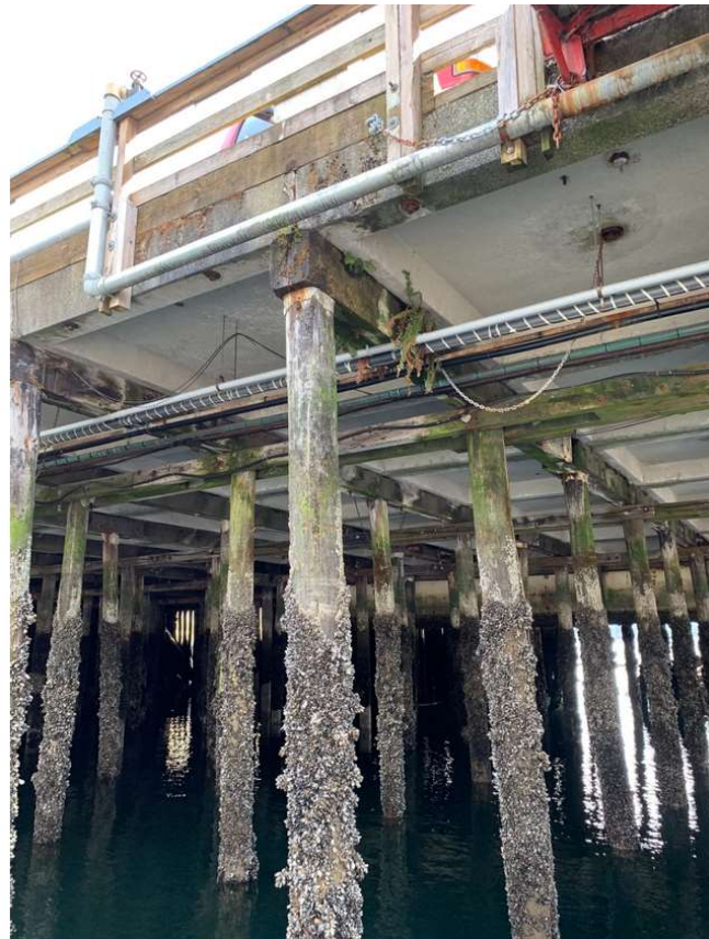
Utilities Interference for Cap Replacements (run under caps and secured to panels)
