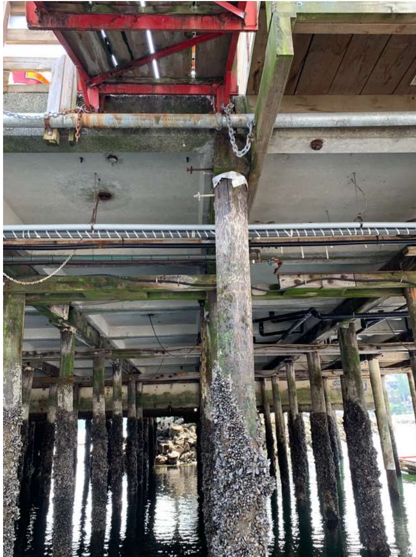
Utilities Interference for Cap Replacements (run under caps and secured to panels)
