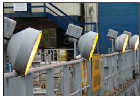
Changing the direction of spotlights can reduce light impact on neighbours.
