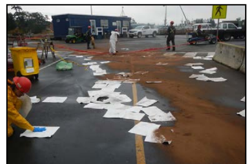
Recovery and clean up.
