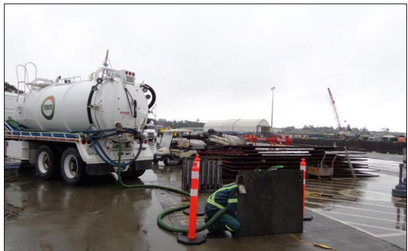
Lift Station Maintenance.
