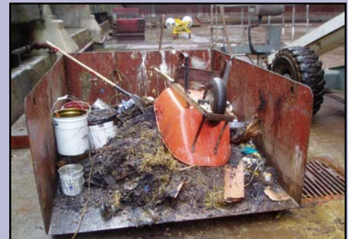
INADEQUATE waste grit storage.
