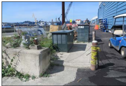
AUTHORIZED Sanitary Sewer Discharge point, Lift Station #11.
