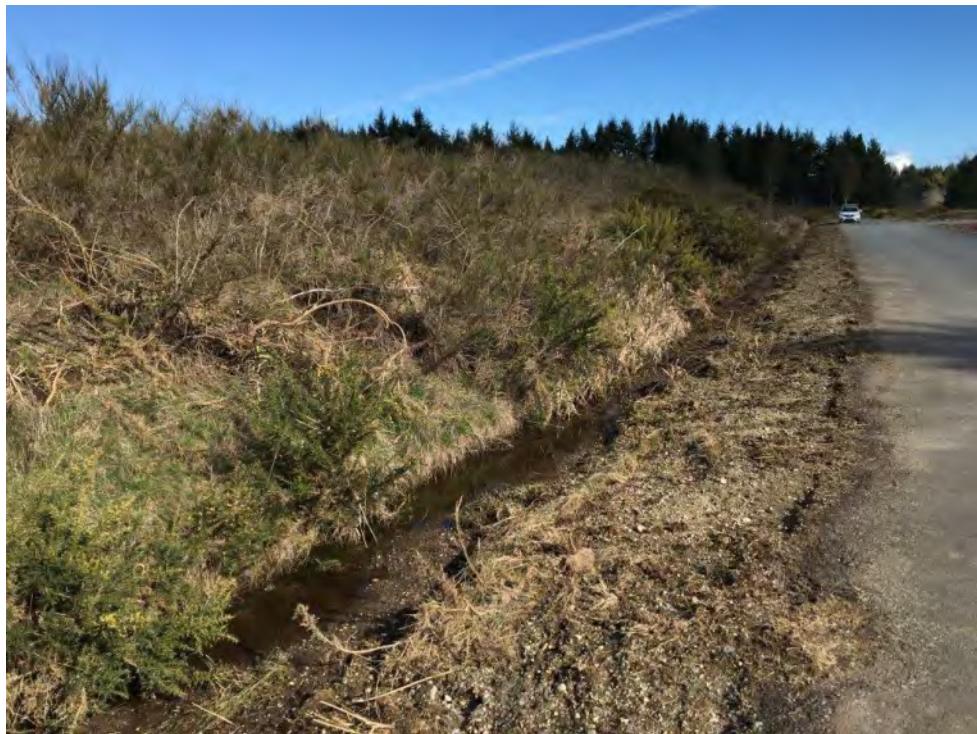
Photograph 12: Drainage ditch along access road.
