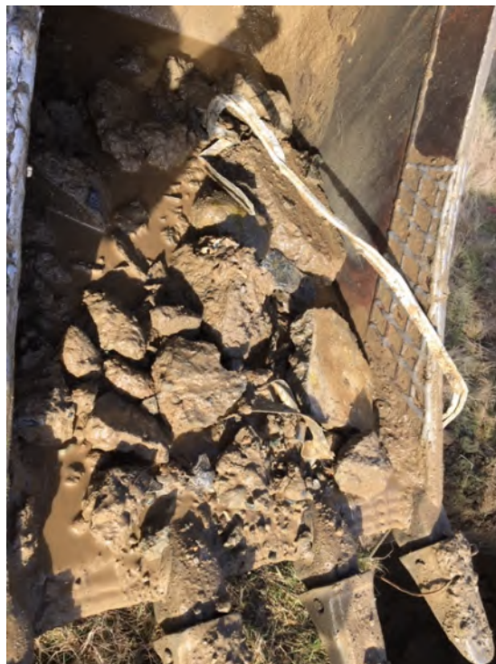
Photograph 2: Example of brick, metal and concrete encountered during test pitting in the debris unit
