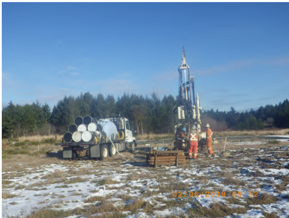
Photograph 4: Looking north during drilling at BH19-07D.
