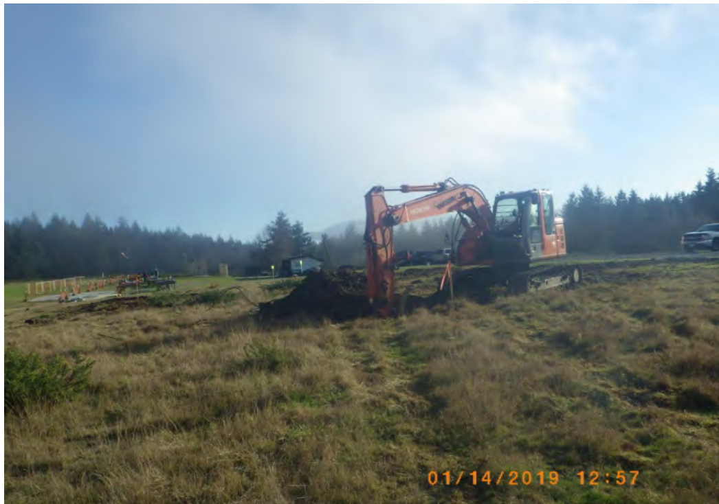
Photograph 6: Excavation of TP19-49 facing east towards PDQ hut.
