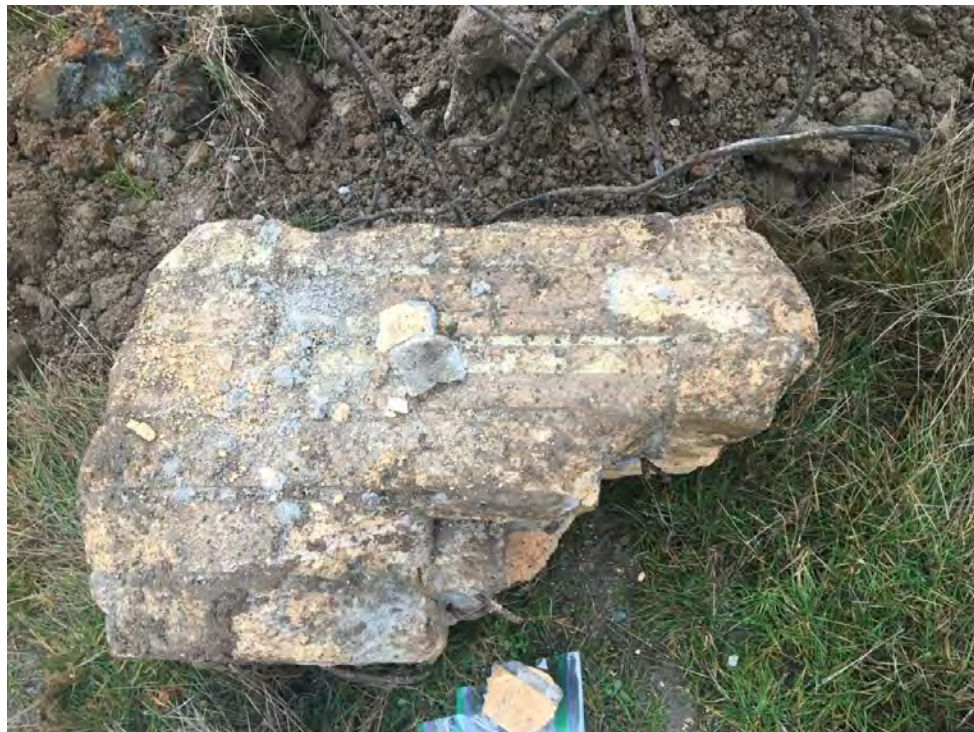
Photograph 4: View of concrete brick debris.
