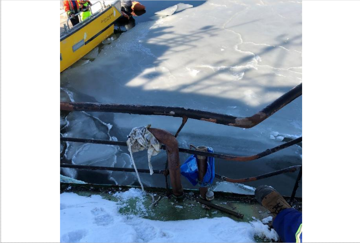
31. View of typical sounding pipe condition (3)
