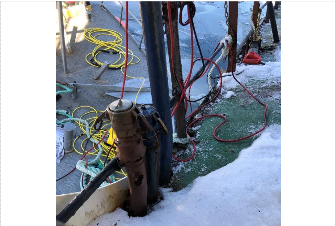
32. View of typical sounding pipes condition (4)
