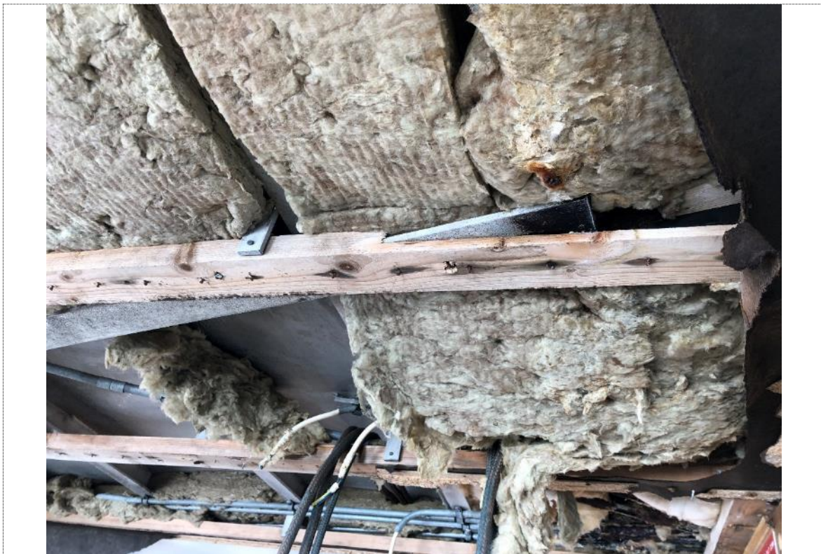
4. Bridge – view of ceiling
