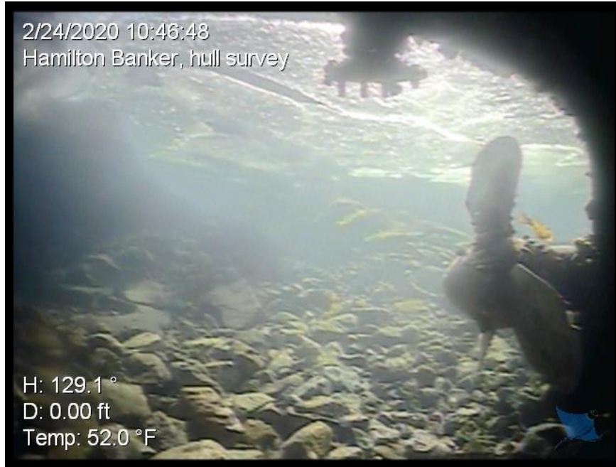
Figure 3 - Stern area showing damaged propeller.
