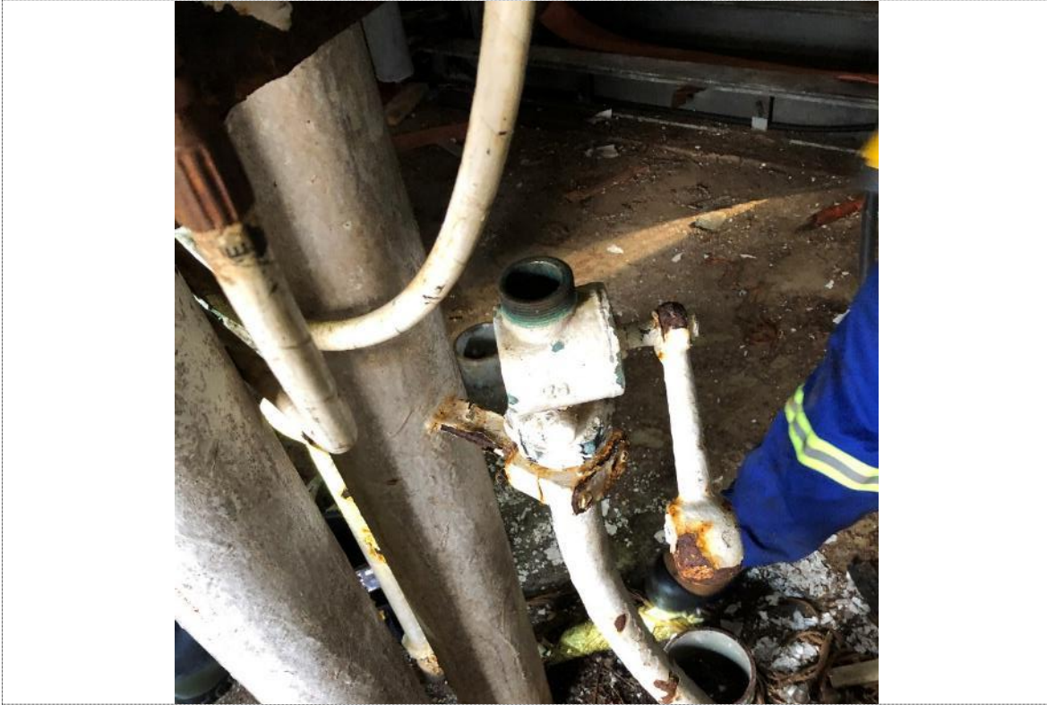
25. Pipes on processing deck prior to cutting to take sounding (1)
