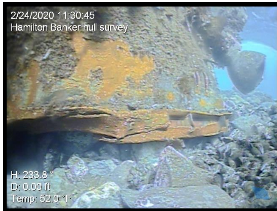
Figure 10 - Aft location showing damage to keel.
