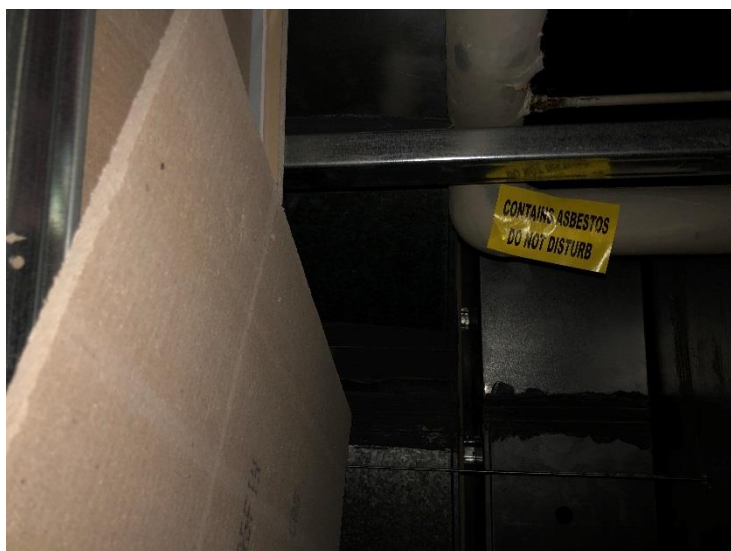
Photo 67: View of asbestos containing pipe insulation on pipe above ceiling tile in the "Maritime Unit" Room M07
