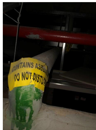
Photo 68: View of asbestos containing pipe insulation on pipe above ceiling tile in the "Maritime Unit" Room M07
