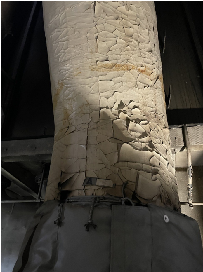
Figure1: Engine exhaust duct insulation
