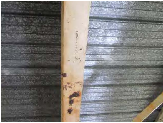
Figure 1 - Off-white paint on the metal structure in the Rearing Ponds areas is lead-containing (Samples LP-01 and LP-04) and is peeling in many locations.
